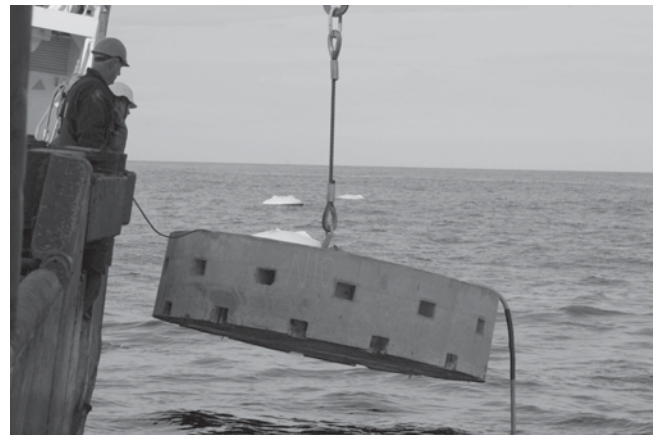
Fig. 5.3 Deployment of a Seabased Ltd wave-energy foundation perforated with 26 holes. Wave-absorbing buoys can be seen in the background (Langhamer and Wilhelmsson 2009, photo Olivia Langhamer)
