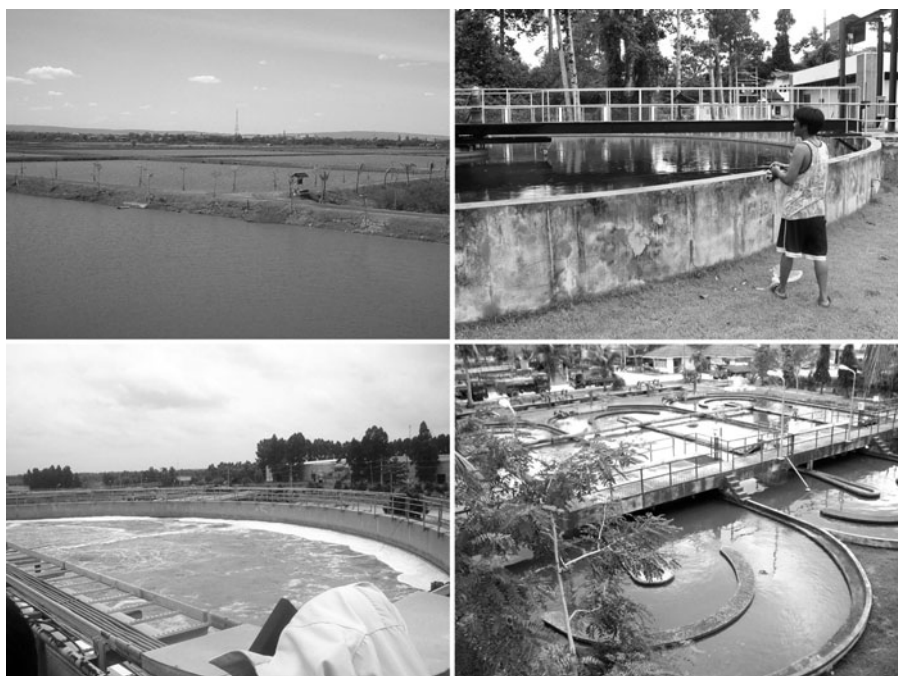
Figure 1-1. Wastewater treatment plants in Thailand. Clockwise from top left: a pond system in Sakon Nakhon; a man fishing in a stalled treatment unit in Samui; a denitrification system in Patong; and an aeration tank in operation in Prachinburi.
