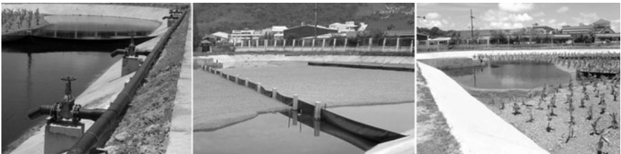
Figure 8-6. (Left to right) Inlet pond, gravel filter before being planted, and outlet pond.
