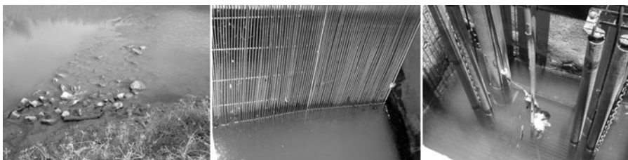
Figure 8-5. Pak Bang inlet structure ( left to right ): damming the river, screen, and pumps.
