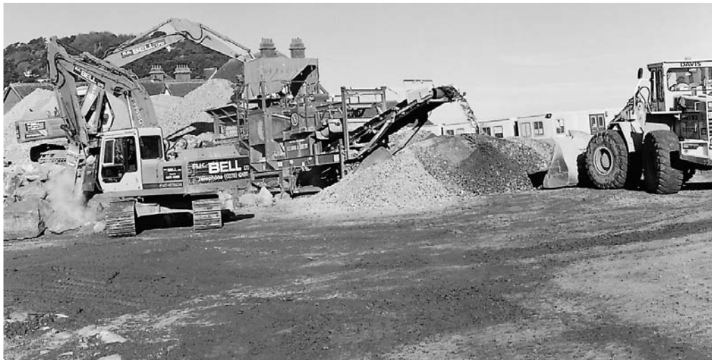
Figure 5.43. Crushing concrete from the old seawall into aggregate for use as a sub-base (courtesy of the Environment Agency)
