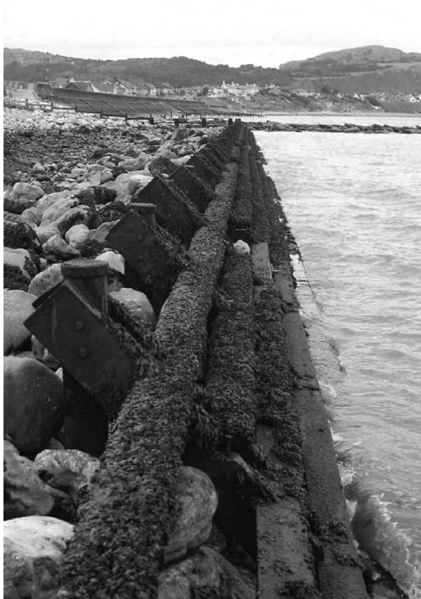
Figure 5.19. Timber and rock revetment, West Wales (courtesy of HR Wallingford)
