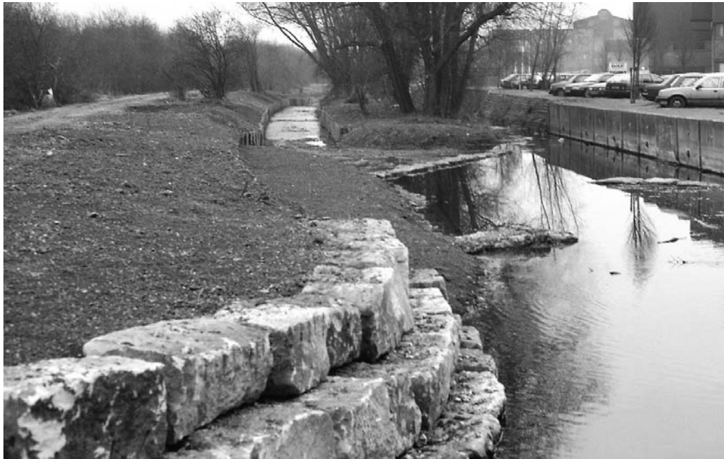
Figure 5.16. Blockstone as a retaining wall and internal groynes to define a low flow channel, Wraysbury River, Poyle (courtesy of the Environment Agency—Thames Region)
