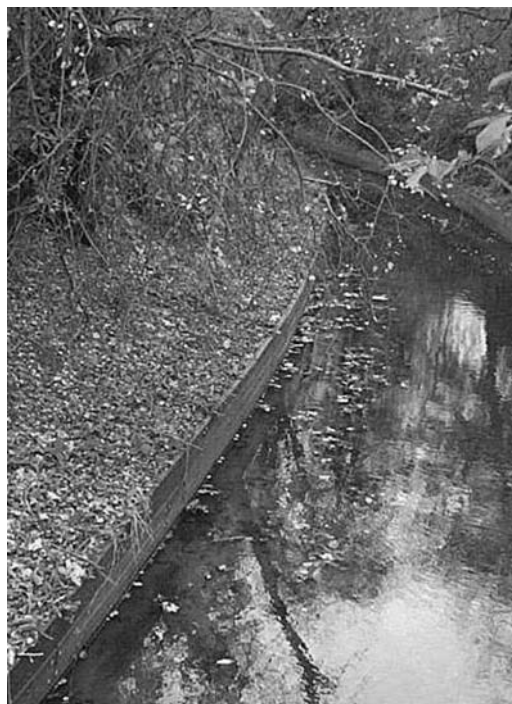
Figure 5.55. Recycled plastic toe boarding, Edgware Brook, North London (courtesy of the Environment Agency)
