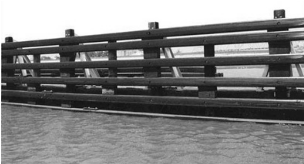
Figure 5.52. Recycled plastic timber used in a guide wall on the Port Allen Lock on the Mississippi River (courtesy of SEAWARD)
