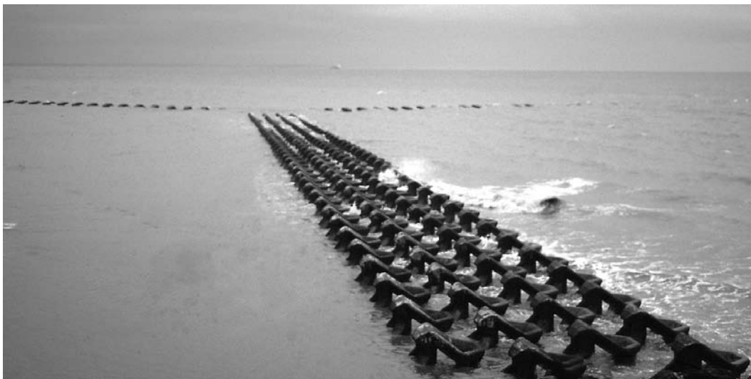
Figure 5.35. Precast concrete fish-tailed groyne, New Brighton, Wirral (courtesy of HR Wallingford)
