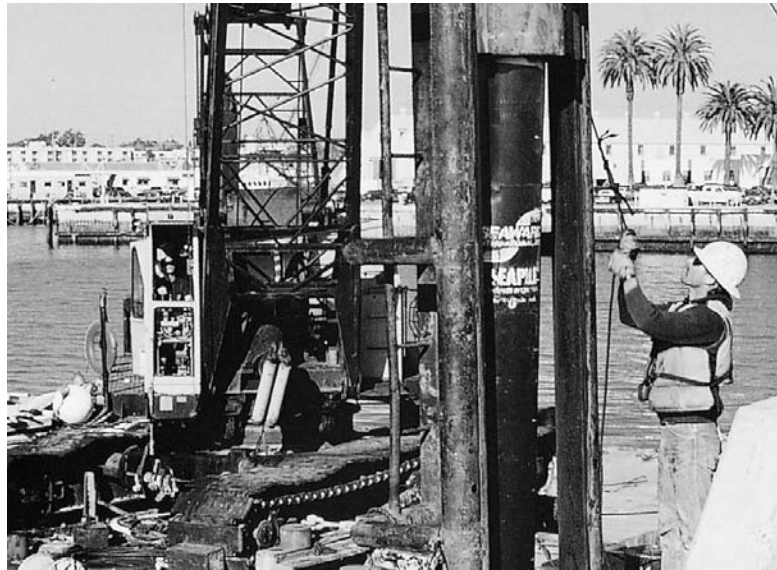
Figure 5.53. Installing recycled plastic piling (courtesy of SEAWARD)
