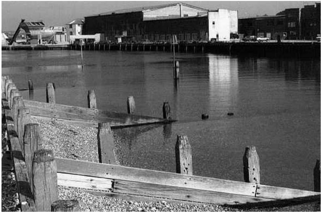
Figure 5.22. Timber groyne field in estuary, Southwold (courtesy of Tom Stevenson)
