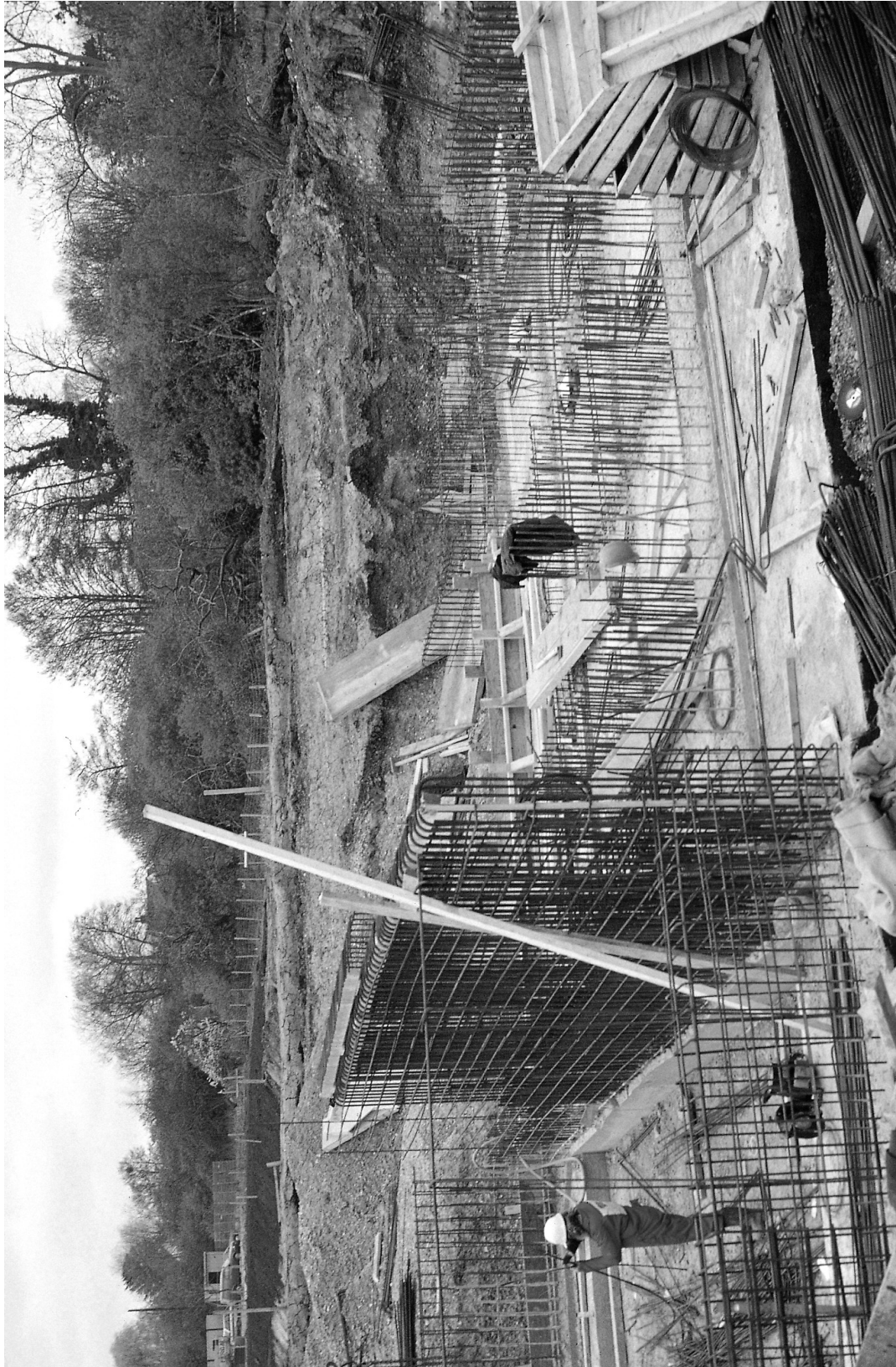
Figure 5.49. Reinforced concrete construction of a new control structure at Tanhouse Farm, Colnbrook, on the Colne Brook (courtesy of the Environment Agency)
