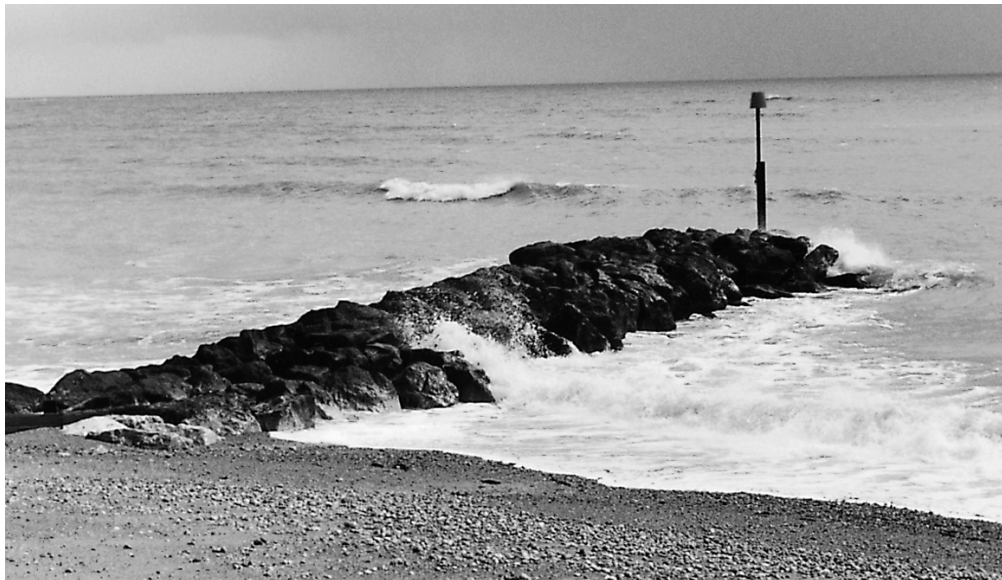
Figure 5.11. Rock groyne, Pagham Harbour, West Sussex (courtesy of HR Wallingford)
