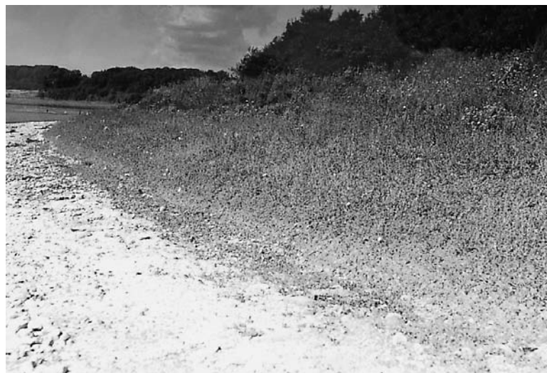
Figure 5.3. Open Stone Asphalt Revetment, Arlington reservoir, Sussex (courtesy of Hesselberg Hydro 1991 Ltd)
