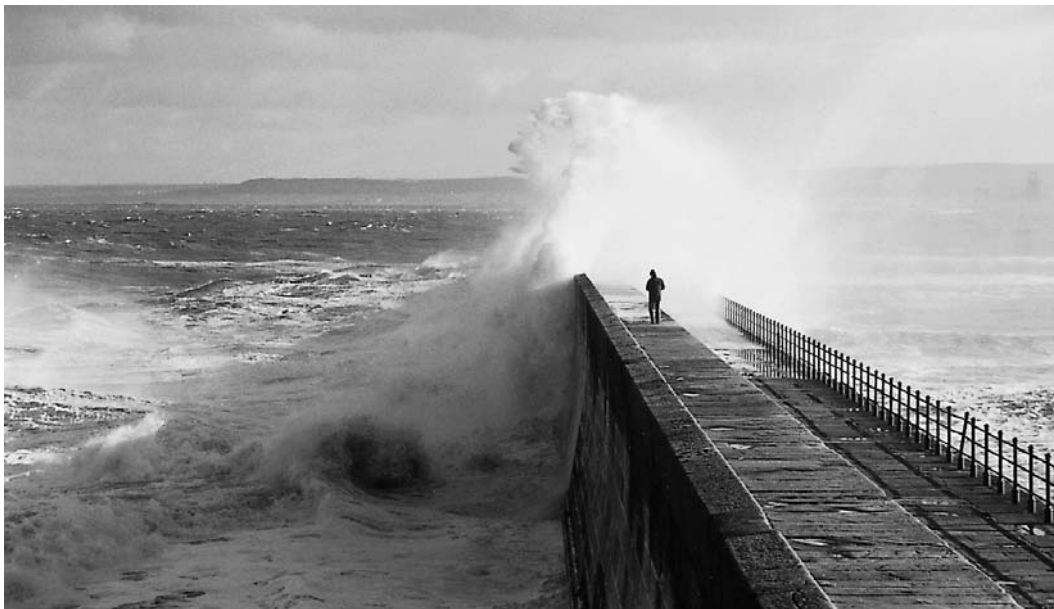
Figure 5.39. Breakwater, masonry blocks with concrete decking, Hartlepool, Durham (courtesy of HR Wallingford)
