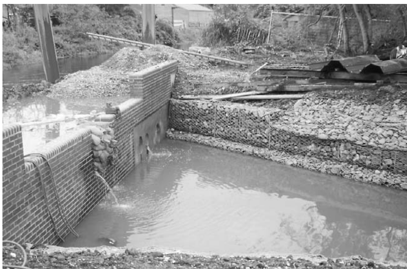
Figure 5.13. Box gabion wall below reno mattress slope protection adjacent to brick clad steel pile weir, Fray's River, Uxbridge (courtesy of the Environment Agency—Thames Region)
