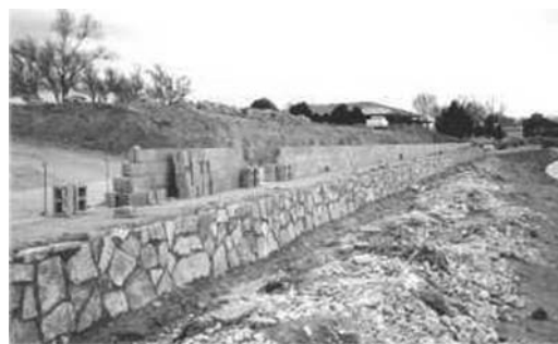
Figure 5.63. Constructing the retaining wall above the concrete coated tyre bales (courtesy of Encore Systems)
