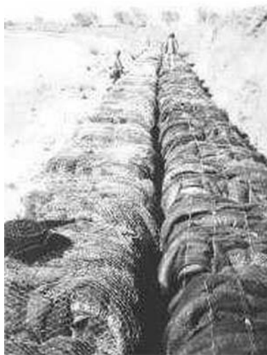
Figure 5.62. Placing the tyre bales in the trench (courtesy of Encore Systems)
