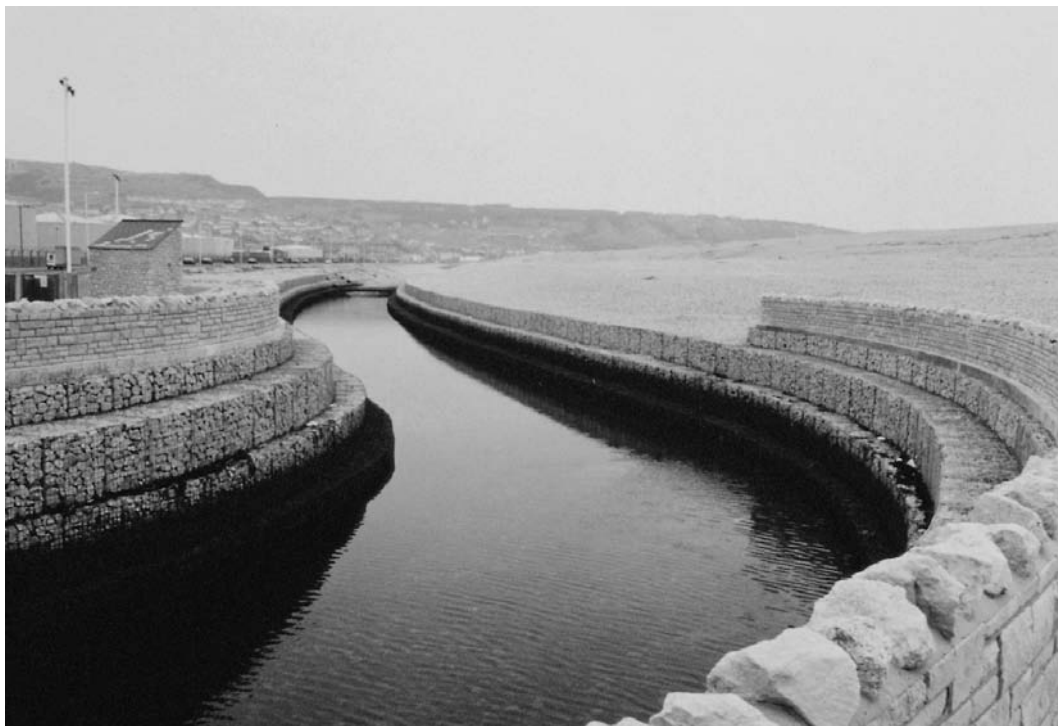
Figure 5.9. Gabion river bank protection, Chesil Beach, Portland Harbour (courtesy of HR Wallingford)
