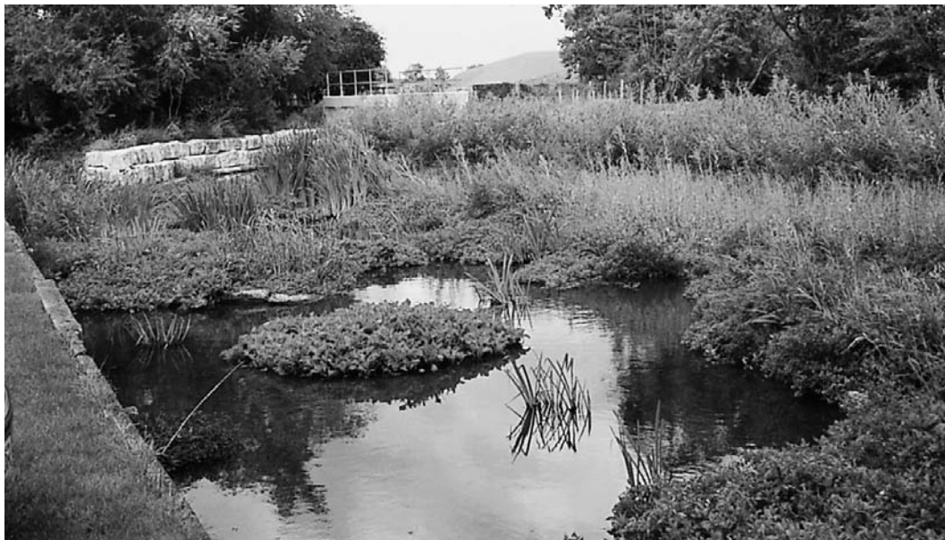
Figure 5.17. Blockstone as a retaining wall and internal groynes to define a low flow channel, Wraysbury River, Poyle, 12 months later than Figure 5.16 (courtesy of the Environment Agency—Thames Region)
