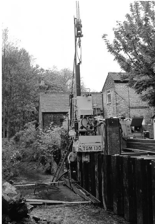
Figure 5.47. Steel sheet piling using a rig that avoids vibration and minimises noise, Wraysbury River at Staines (courtesy of the Environment Agency—Thames Region)
