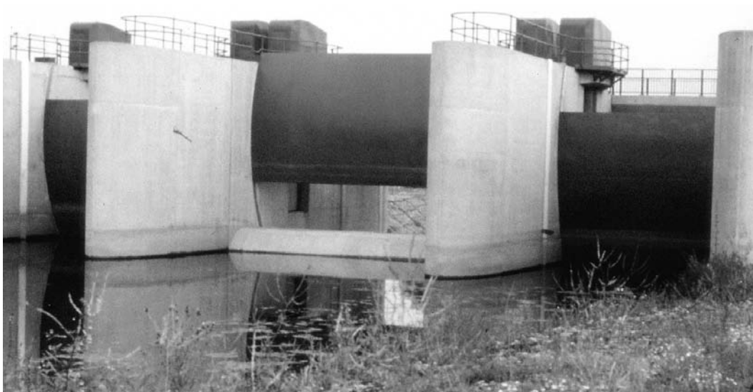
Figure 5.48. In-situ concrete structure with large steel gates, River Medway, Tonbridge Flood Storage Reservoir (courtesy of David Hockin)
