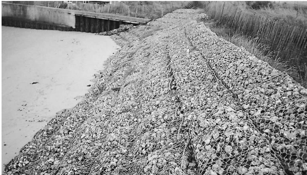
Figure 5.6. Gabion revetment, Brancaster, Norfolk (courtesy of HR Wallingford)
