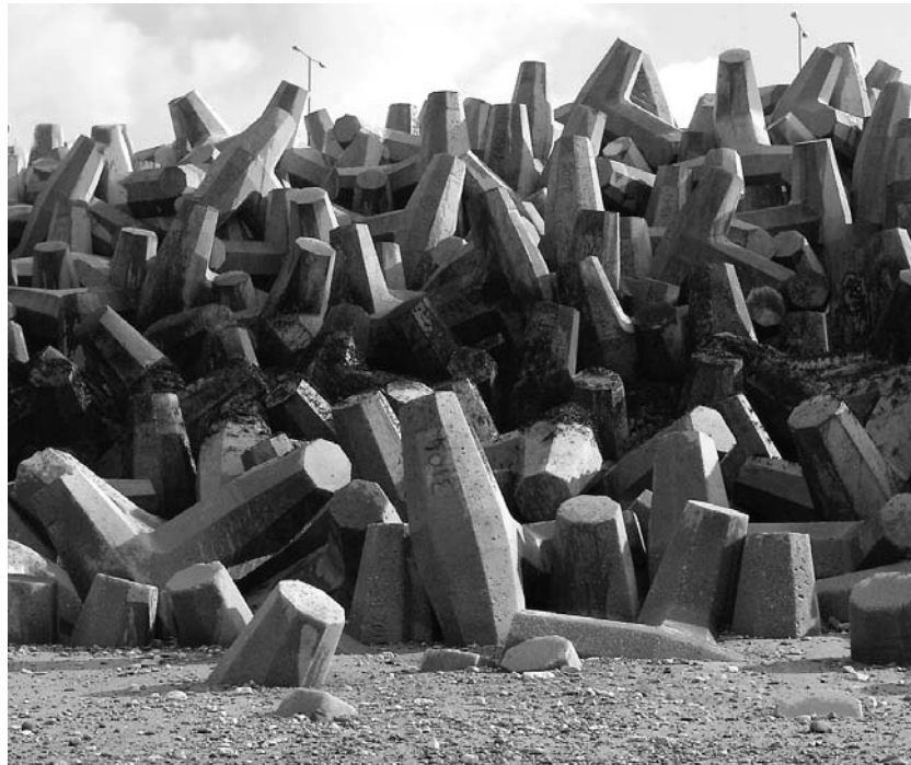
Figure 5.36. Dolos, precast concrete interlocking armour units, Penmaen Head, A55 trunk road, North Wales (courtesy of HR Wallingford)
