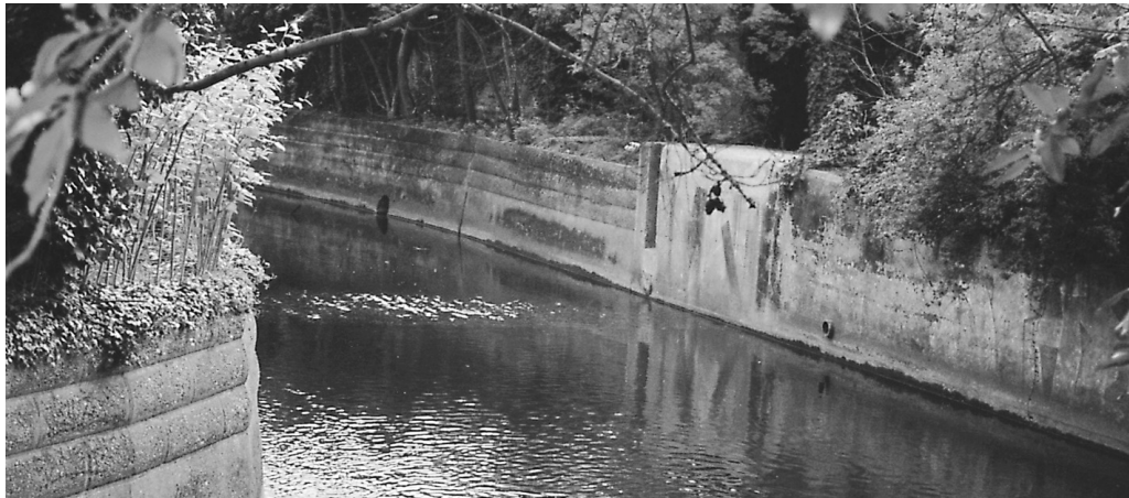
Figure 4.4. Derelict Autoweir, Whitton Road, River Crane after demolition works and reinstatement of the rock and gravel bed (courtesy of the Environment Agency)
