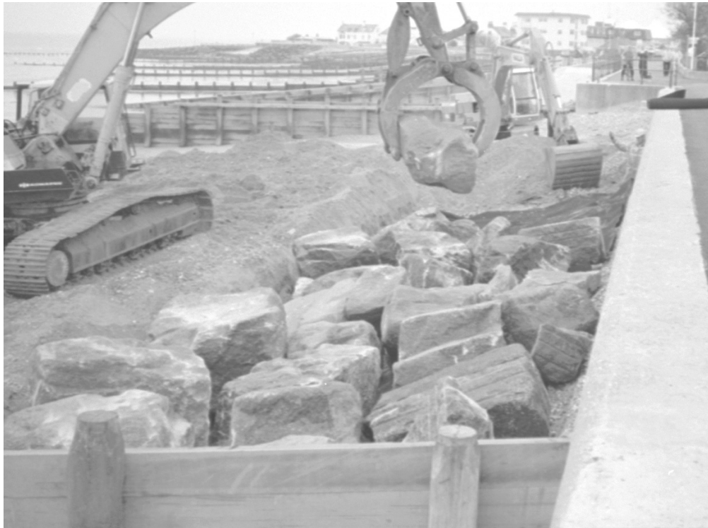
Figure 5.10. Placing armourstone in Felpham sea defences (courtesy of Arun District Council)
