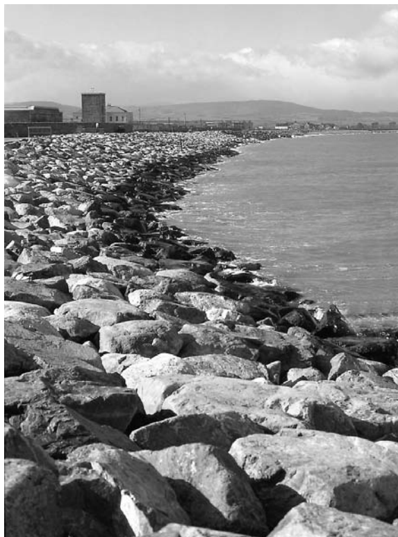
Figure 5.7. Rock armourstone revetment, Arklow, County Wicklow, Ireland (courtesy of HR Wallingford)
