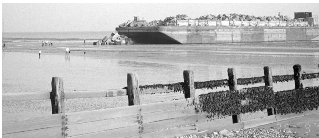
Figure 5.18. 'Waste' rock transported from Norwegian quarries by barge for use in sea defences at Felpham, West Sussex (courtesy of Arun District Council)
