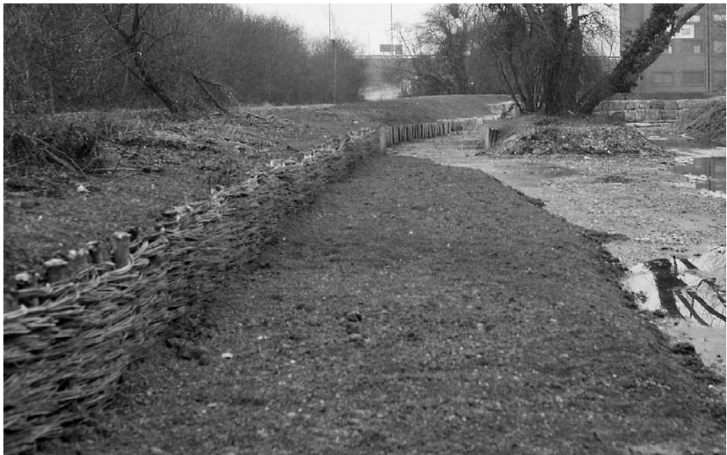
Figure 5.23. Willow spiling used as a low retaining wall, Wraysbury River, Poyle (courtesy of the Environment Agency—Thames Region)
