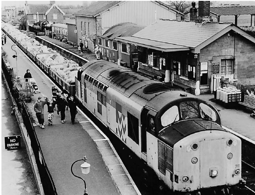
Figure 5.44. Delivery of primary rock armour by rail (courtesy of the Environment Agency)
