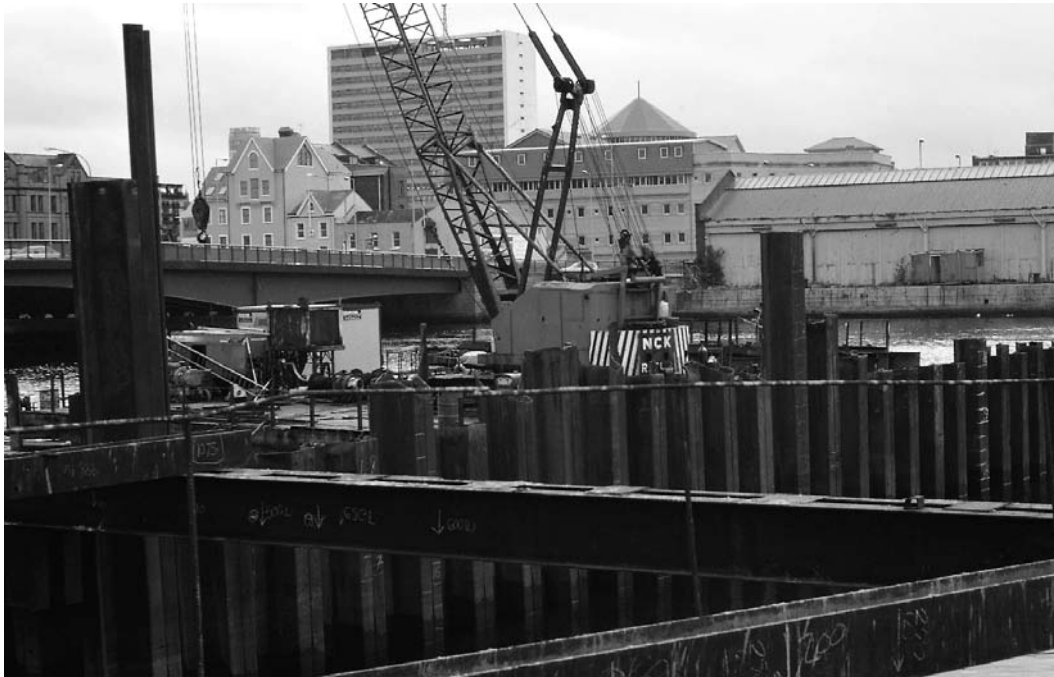
Figure 5.50. Reinforced concrete construction utilising a large amount of temporary steel piling, Lagan Weir, Belfast (courtesy of A. T. Pepper)
