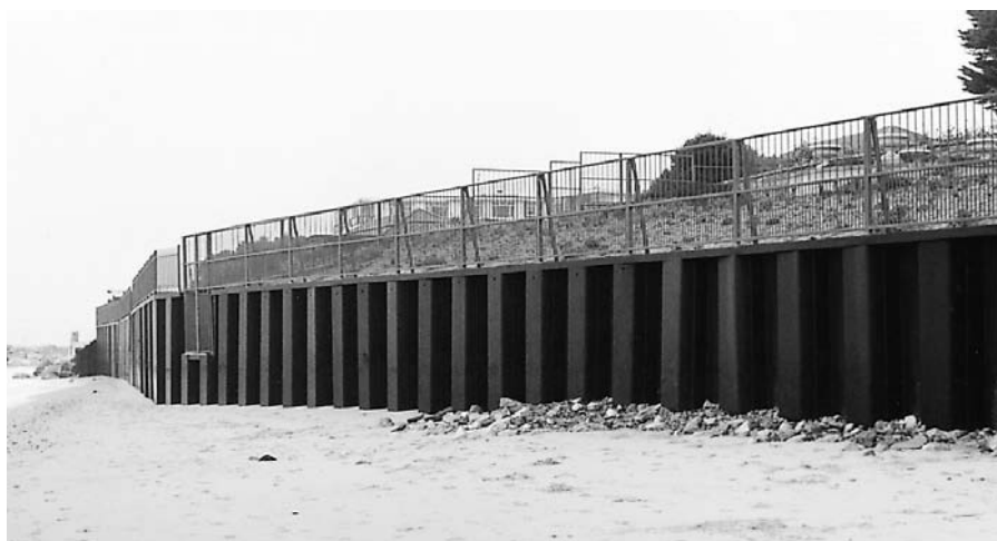
Figure 5.46. Steel sheet piling, concrete and reinforcing steel at Sandbanks, Poole Bay, Dorset (courtesy of HR Wallingford)
