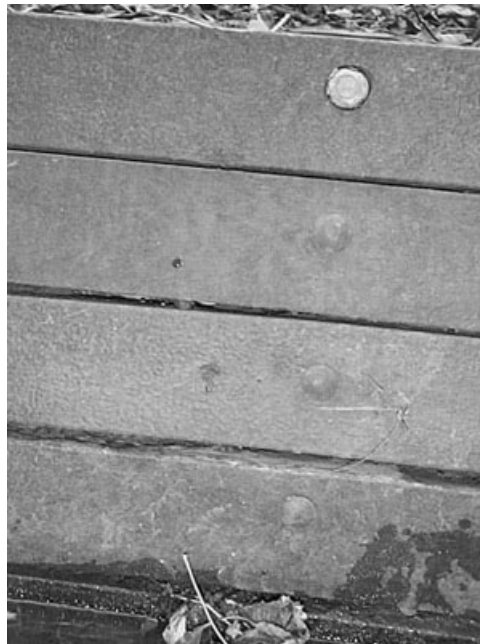
Figure 5.56. Recycled plastic toe boarding, Edgware Brook, North London (courtesy of the Environment Agency)
