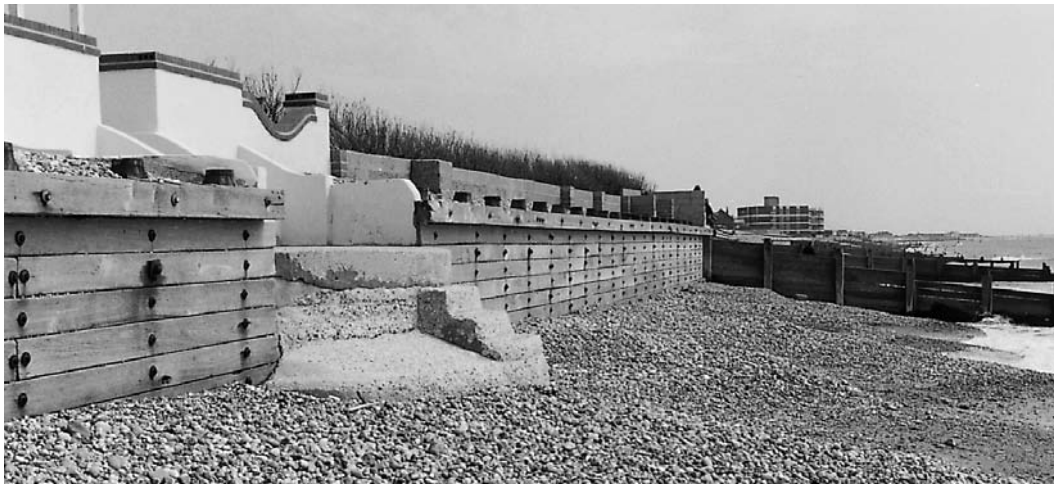
Figure 5.21. Timber seawall and groyne field, East Wittering, West Sussex (courtesy of HR Wallingford)
