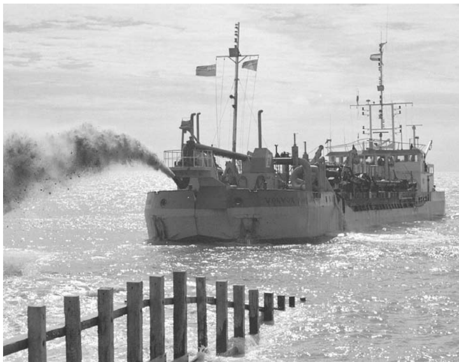
Figure 5.32. Spraying aggregate directly onto the foreshore for use in beach renourishment (courtesy of Arun District Council)
