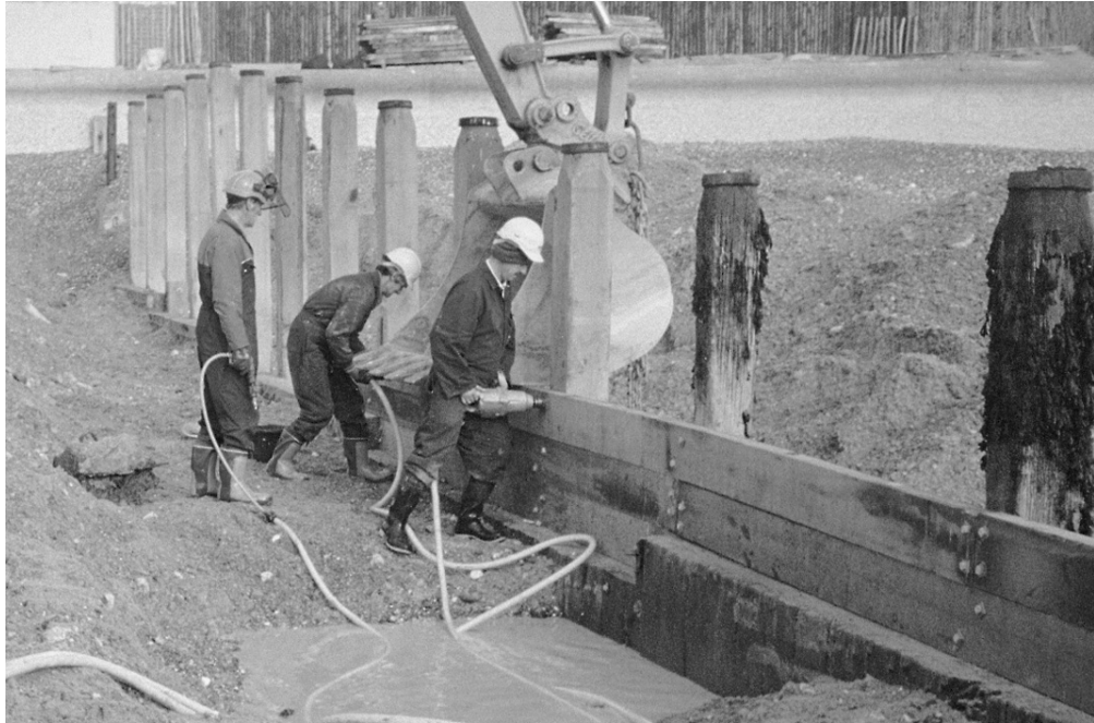
Figure 5.28. New timber being installed above recycled timber sheet piling (courtesy of Arun District Council)
