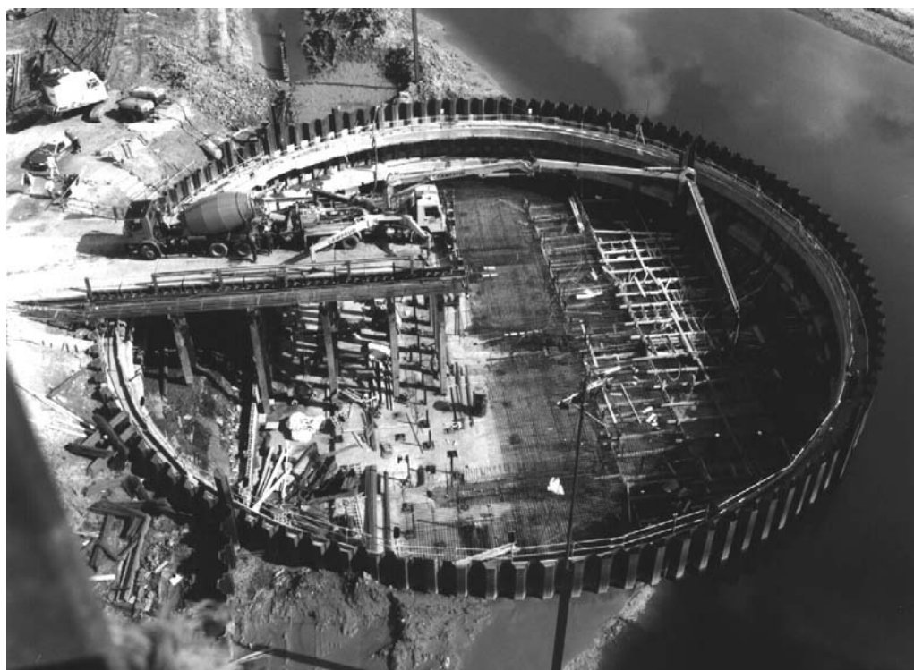
Figure 5.51. Temporary cofferdam used during the construction of Welmore Sluice (courtesy of the Environment Agency)
