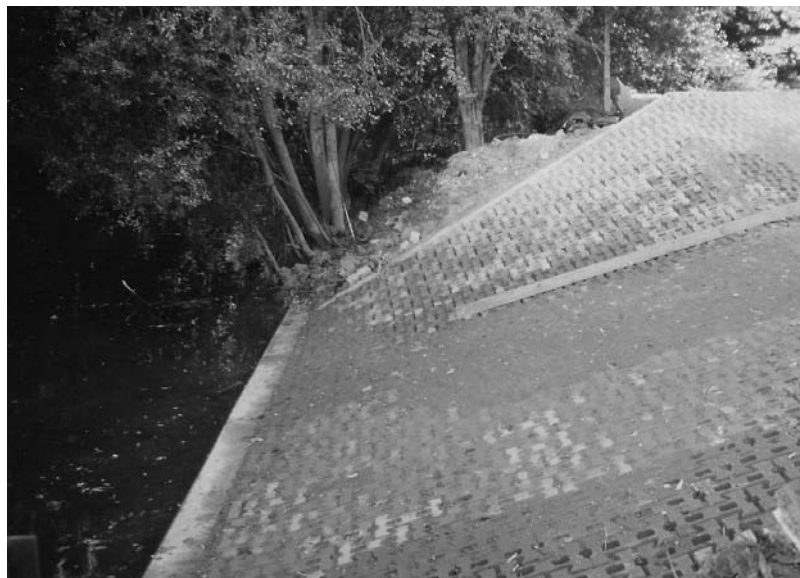
Figure 5.41. Cellular concrete revetment, Staines Bypass Channel outfall to River Thames (courtesy of the Environment Agency—Thames Region)
