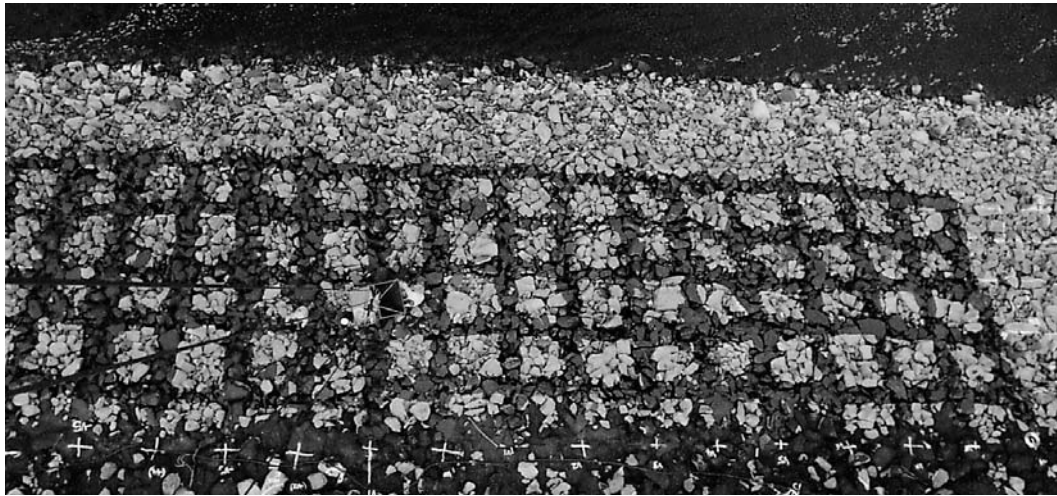
Figure 5.2. Pattern grouted revetment, Megget reservoir, Scotland (courtesy of Hesselberg Hydro 1991 Ltd)
