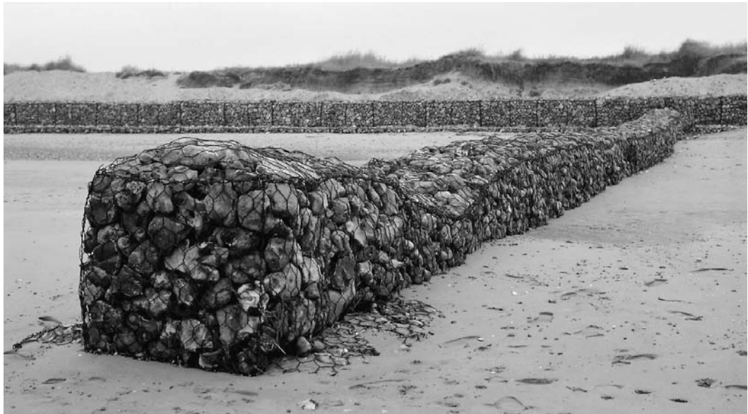
Figure 5.8. Gabion groyne and seawall, Hunstanton, North Norfolk (courtesy of HR Wallingford)
