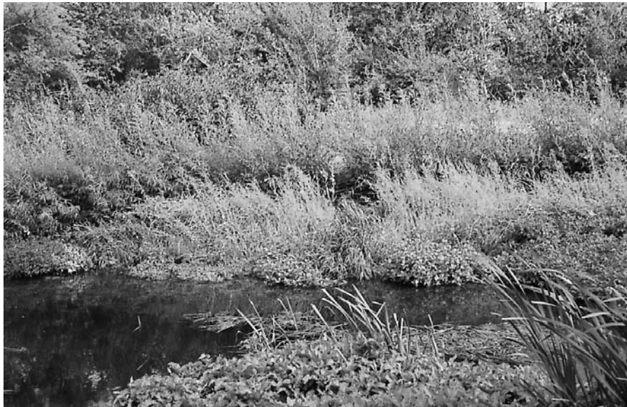
Figure 5.24. Willow spiling used as a low retaining wall, Wraysbury River, Poyle. View of spiling from opposite bank showing growth after 12 months (courtesy of the Environment Agency — Thames Region)
