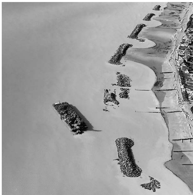
Figure 5.12. Barge delivering armourstone for use in offshore breakwaters, Elmer, West Sussex (courtesy of Arun District Council)
