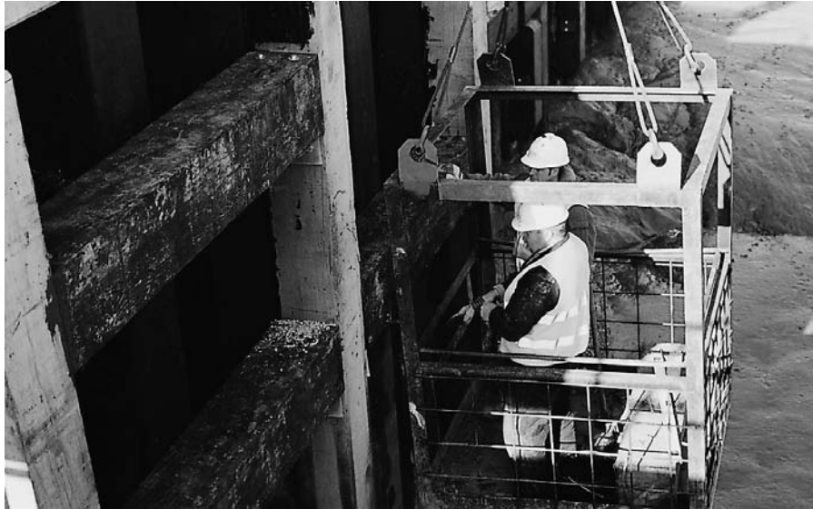
Figure 5.29. Engineers inspecting the work done to put the 130 year old beams in place
