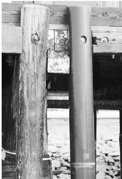
Figure 5.54. Composite marine piling installed as a replacement to a traditional wood fender pile (courtesy of SEAWARD)
