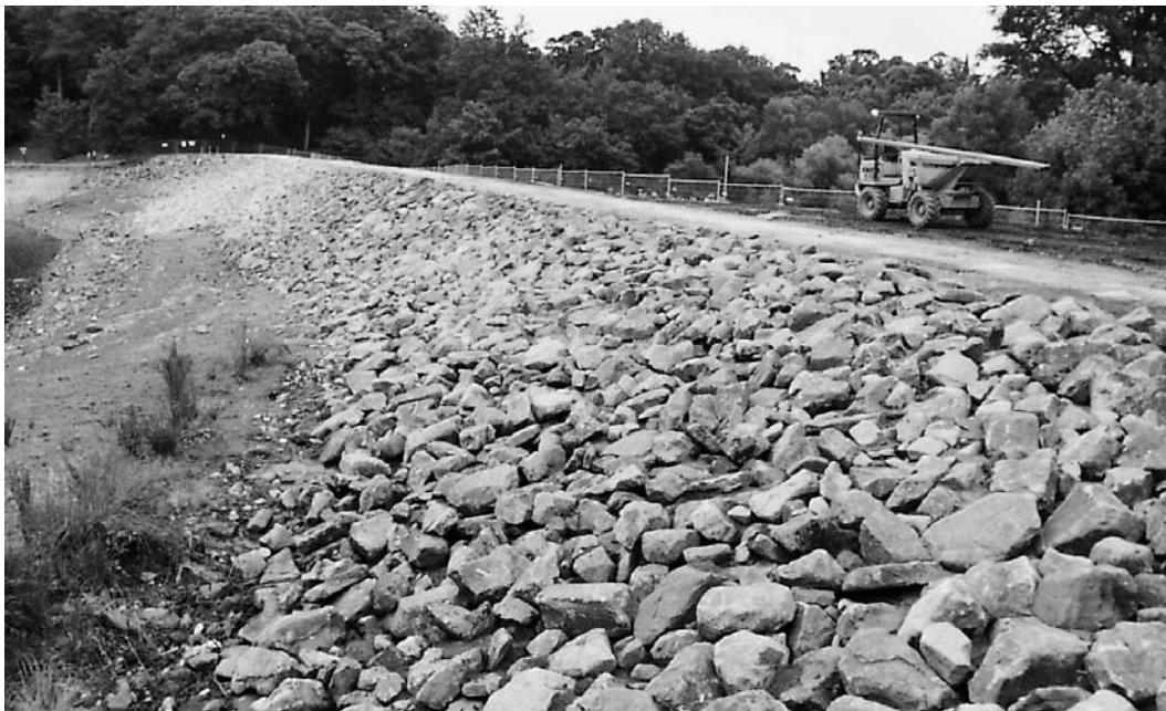
Figure 5.5. Grout around rock to retain natural appearance, Waterloo Lake, Leeds (courtesy of Hesselberg Hydro 1991 Ltd)
