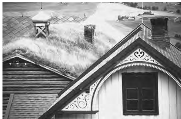
Figure 3.16 Ecoroofs are an update on traditional sod roofs—an example of revisiting past technologies to meet sustainability goals. (Photo: Kim Sorvig.)
