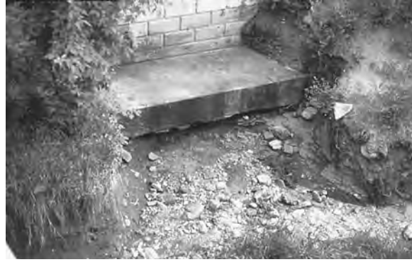
Figure 2.I2 Rigid structures protect only the soil they can shield from water. Along the hard edges, erosive undercutting is actually increased. (Photo: Kim Sorvig.)
