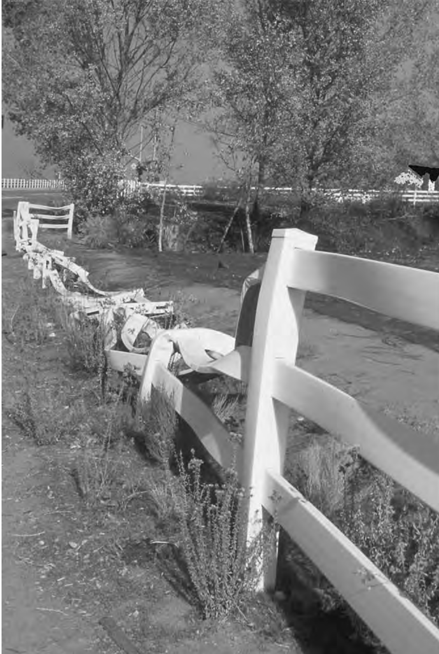
Figure 2.17 In fire-adapted ecosystems, structures must adapt. Plastic fencing melted and the house (right rear) narrowly escaped (San Diego area). (Photo: Kim Sorvig.)
