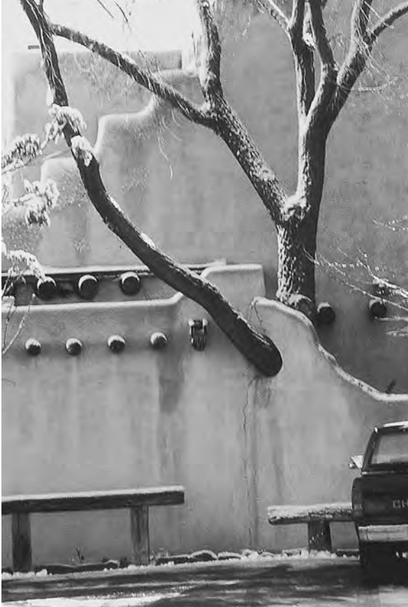
Figure 6.9 Adobe is one of the most flexible materials to work with, and inspires site-specific construction that celebrates existing features like this tree. (Photo: Kim Sorvig.)
