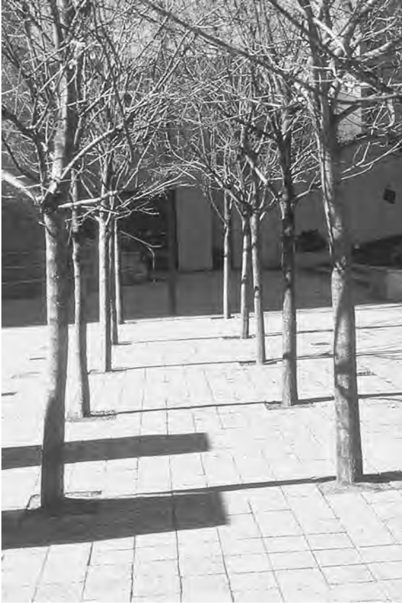
Figure 5.13 Henry Arnold has used open-jointed unit pavers at large plazas in Atlanta GA, Brooklyn NY, and Newport NJ, usually with extra aeration vents. ( Project and Photo: Henry Arnold. )
