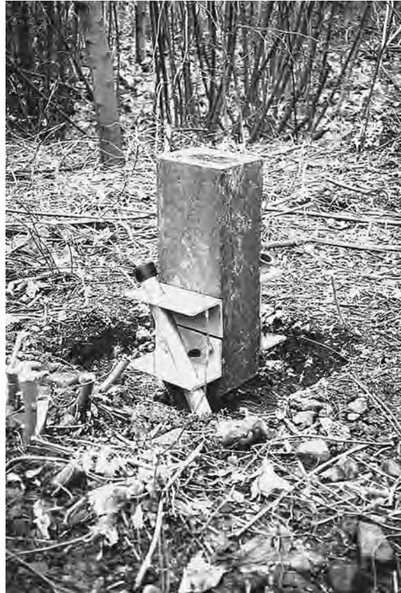
Figure 6.16 Recycled plastic lumber piers support decks along the Upper Charles River near Boston. Metal “pinned foundations” cause almost no site disruption and can be removed or adjusted easily. (Project and Photo: Carol R. Johnson and Associates.)
