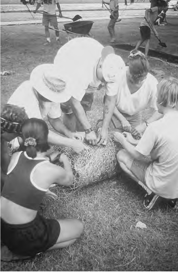
Figure 4.13 University of Oregon landscape students fabricated “soil burritos” of fabric, soil, and chicken-wire for a campus restoration, demonstrating a simple, inexpensive method. ( Project and Photo: Professor Stan Jones.)
