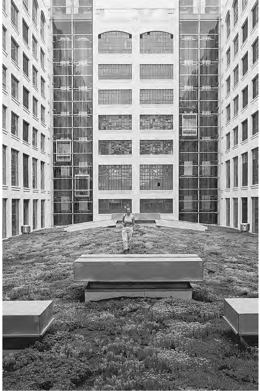
Figure 3.17 Montgomery Park Business Center (Baltimore) boasts a thriving lightweight greenroof. (Project: Katrin Scholz-Barth. Photo: Kai-Henrik Barth.)
