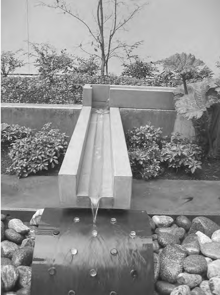
Figure 4.23 Close-up of I0th@Hoyt stormwater conveyances. (Project: Steve Koch. Photo: Stuart Echols.)
