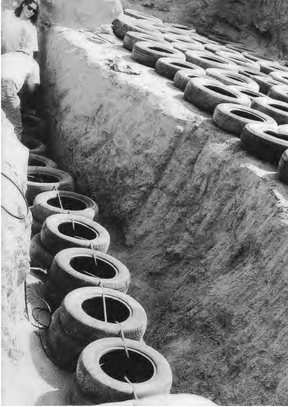
Figure 6.14 Check dams reuse waste tires to stabilize an arroyo in Arizona. Tires in trench form a footing for the dam at the upper level. (Project and Photo: Stuart Hoenig and Joshua Minyard.)
