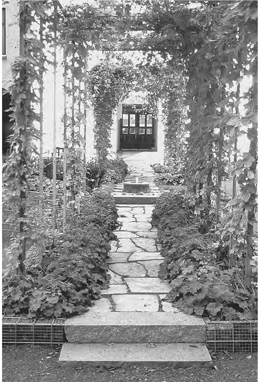
Figure 6.4 Salvaged during demolition, roof tiles form curbs and gutters, and fill gabion-like planted walls in this urban garden in Oslo, Norway. Crushed tile surfaces paths, and serves as concrete aggregate. Stone, too, is second hand. (Project: Snøhetta Landskapsarkitekter. Photo: Rainer Stange.)
