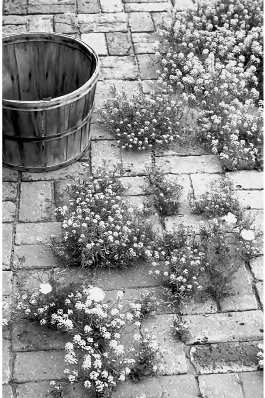
Figure 5.12 In small-scale, low-traffic areas, unit pavers can even support wildflowers. (Project: R. and V. Sorvig. Photo: Kim Sorvig.)
