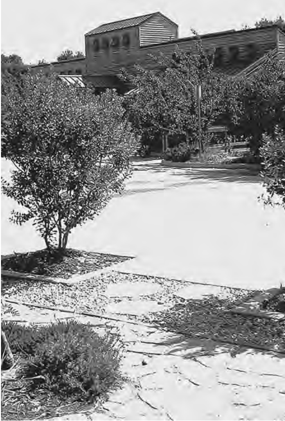
Figure 6.5 Broken concrete, reused in slabs or crushed as aggregate, demonstrate John Lyle's concepts at the Institute for Regenerative Studies. (Project and Photo: John Lyle.)
