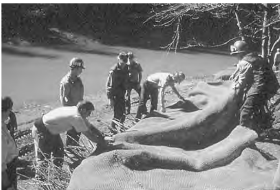
Figure 3.2 Lakeshore stabilization at Whiskeytown CA. Soil wraps are being constructed on top of brushlayers. (Project: Salix Applied Earthcare. Photo: John McCullah.)
