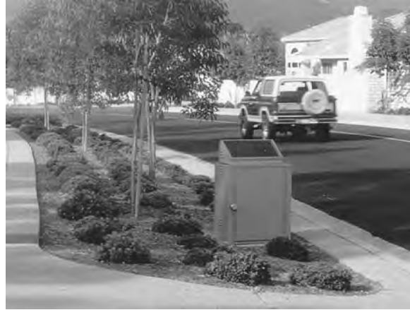
Figure 4.24 This large Photocomm solar irrigation controller uses an inverter to provide 110V AC power to standard valves. (Photo: Photocomm/Golden Genesis Co.)
