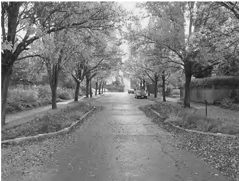
Figure 5.16 “Green streets” (like Siskyou St., Portland OR) collect water from wider areas with parking, and infiltrate it in “bump-out” planted areas that also help traffic calming. (Project: Portland Bureau of Environmental Services. Photo: Kevin Robert Perry and Portland Bureau of Environmental Services.)
