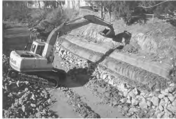
Figure 3.4 Brushlayer installation can be done by hand or aided by equipment. (Project and Photo: Biohabitats Inc.)
