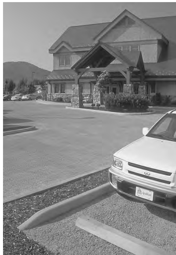
Figure 5.3 Porous parking is separated from standard driving lanes. This stormwater management tactic can also create strong aesthetics. (Project: Spaceplan (arch.); Petrus (pervious paving). Photo: Bruce Ferguson.)
