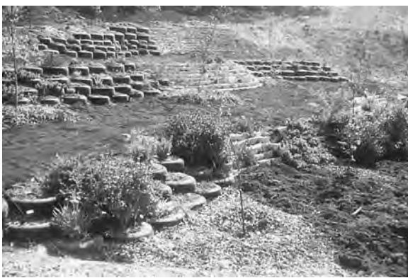
Figure 6.13 Tires and broken concrete achieve unexpected elegance as terraces at the Institute for Regenerative Studies. (Project and Photo: John Lyle.)
