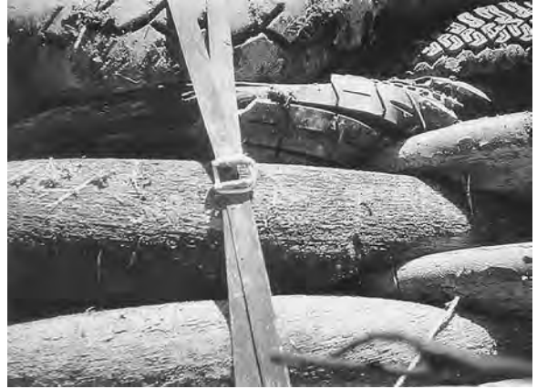
Figure 6.15 Strapped in place, tires form a strong flexible structure that traps sediment and eventually supports plants. Some systems incorporate live staking. (Project and Photo: Stuart Hoenig and Joshua Minyard.)
