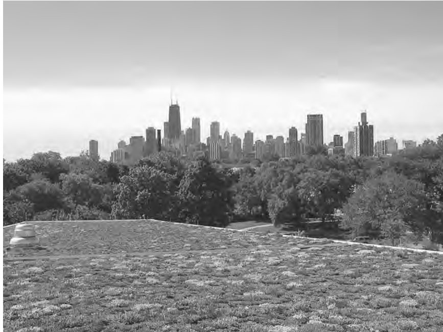
Figure 3.13 Lightweight, “extensive” greenroof covers Peggy Notebaert Nature Museum in Chicago. (Project: Conservation Design Forum. Photo: Andrea Cooper, Conservation Design Forum.)
