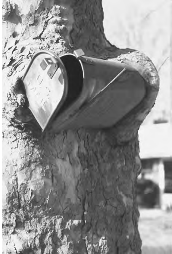
Figure 10.3 Neither wind nor rain . . . but this Sycamore stopped the U.S. mail. Growth and change are inevitable landscape forces that design and maintenance must work with, not against. (Photo: Kim Sorvig.)
