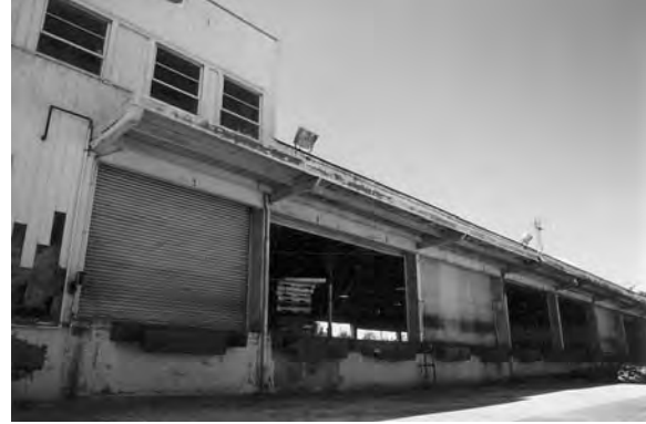
Figure 6.6 This unpromising site was reborn as a garden—without major demolition. (Photo: Jeffrey Miller.)
