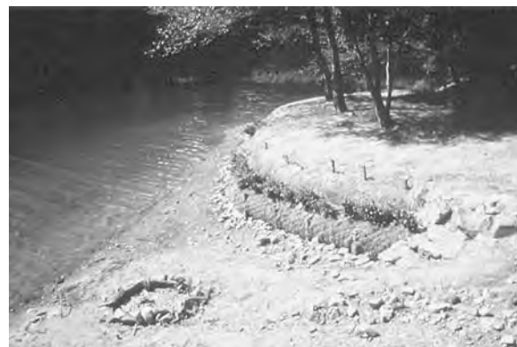
Figure 3.3 Three weeks later, willow twigs are sprouting between wrapped soil layers. The willows will be at water level once the lake is refilled. (Project: Salix Applied Earthcare. Photo: John McCullah.)
