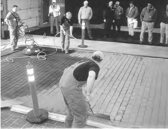
Figure 5.17 Decorative color coatings for asphalt can lighten the surface, decreasing heat-island effects. Integral color, mixed into hot asphalt, is also becoming available. (Photo: StreetPrint, Scott Hind.)
