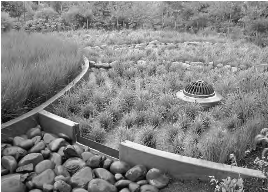
Figure 5.6 This bioswale, part of Glencoe School’s green street in Portland OR, uses check dams, a “flash-board” level-setting device in the weir, and overflow drain to treat and infiltrate stormwater. (Project: Portland Bureau of Environmental Services. Photo: Kevin Robert Perry and Portland Bureau of Environmental Services.)
