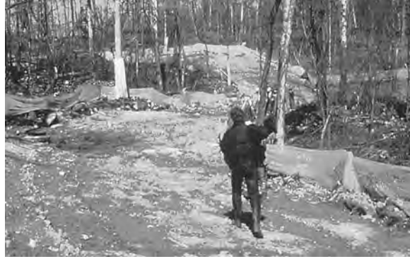
Figure I.6 This easement, in Loudon County VA, is less than half as wide as the utility’s standard. Note the site protection fence. ( Project: Park Authority, HOH Associates, and Rhodeside and Harwell. Photo: Doug Hays.)
