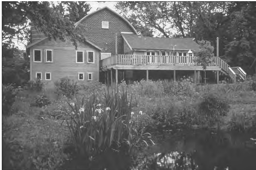
Figure 4.30 Indian Creek Nature Center (Cedar Rapids IA) illustrates Alex Wilson's vision of constructed wetlands doubling as flowerbeds. (Project and Photo: NAWE.)
