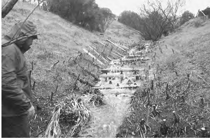
Figure 3.5 Fabric anchored with logs, live stakes, and fast-sprouting grass, in place only a few weeks when this storm struck, survived with no losses. (Project and Photo: Andrea Lucas.)
