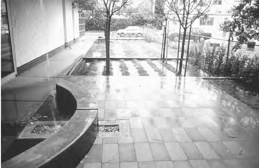
Figure 4.20 Rainwater from a roof drain is caught in a gravel basin and routed to furrows in the garden at the Denver offices of designer Bill Wenk. (Project and Photo: Bill Wenk.)
