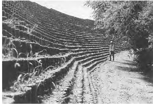
Figure 3.11 Cellular containment materials are flexible honeycombs filled with soil or gravel. A single layer can form a drivable surface; stacked as shown, cells form a greenwall. (Photo: Webtec. ↻)
