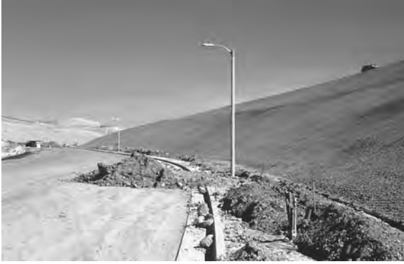
Figure 2.8 Conventional grading insists on uniform, planar slopes. Until recently, objections to this approach have been aesthetic, but recent research shows environmental disadvantages, too. (Photo: H. J. Schor.)
