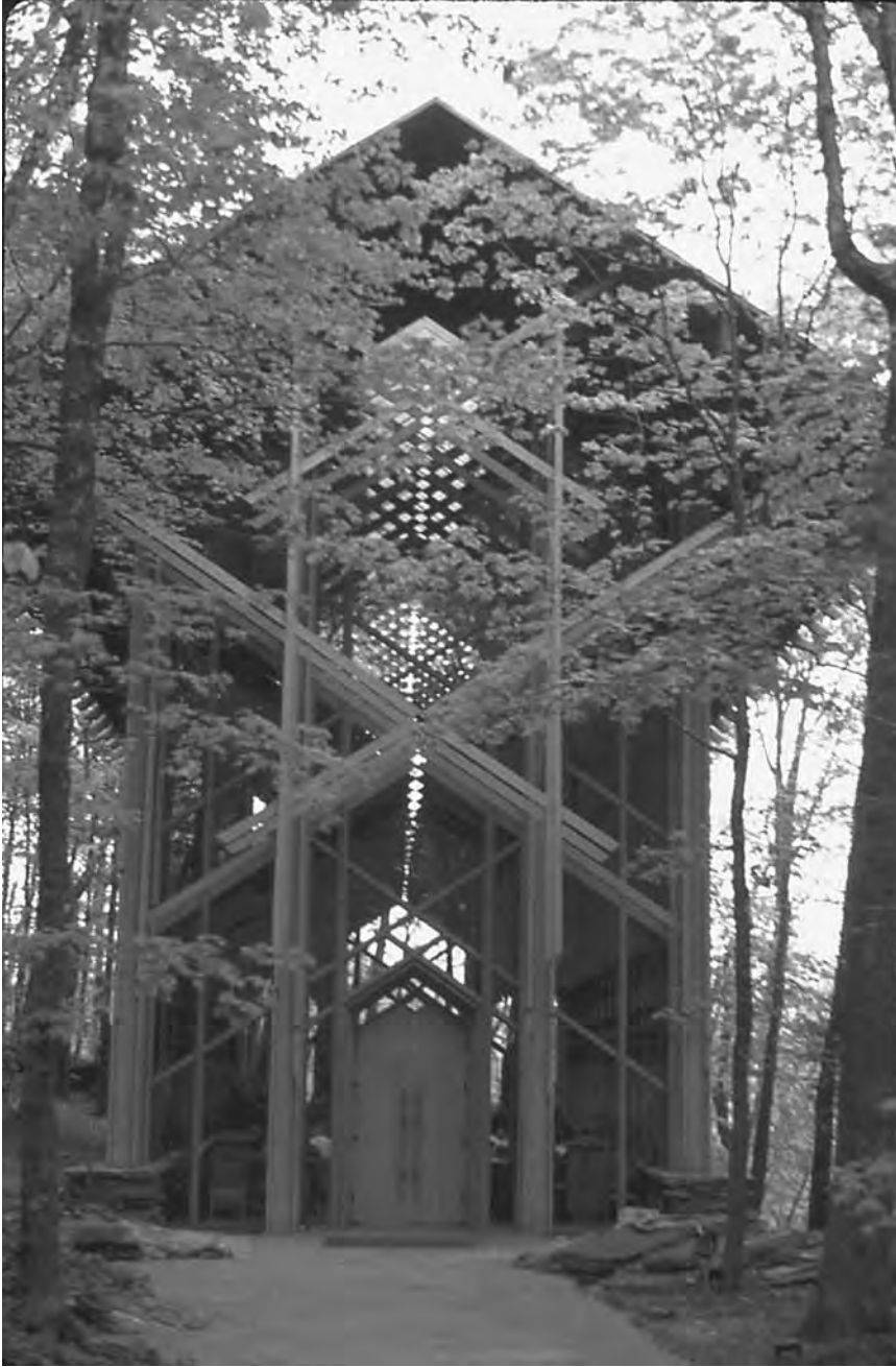
Figure I.14 Thorncrowne Chapel is a national treasure, in part because nonmechanized construction preserved its relationship to the woods. ( Project: E. Fay Jones. Photo: Stephen Schreiber.)
