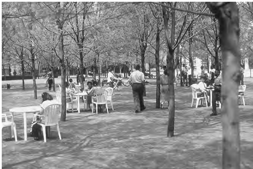
Figure 5.4 Stone screenings over air-entrained soil at MetroTech in Brooklyn create a permeable surface with the feel of traditional French public spaces. (Project and Photo: Henry Arnold.)
