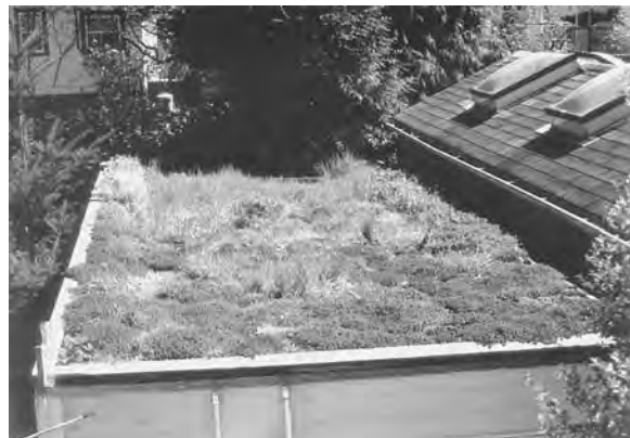
Figure 3.20 Even small-scale ecoroofs decrease runoff, support habitat, and clean the air. Tom Liptan replaced his conventional garage roof with this one. (Project and Photo: Tom Liptan.)
