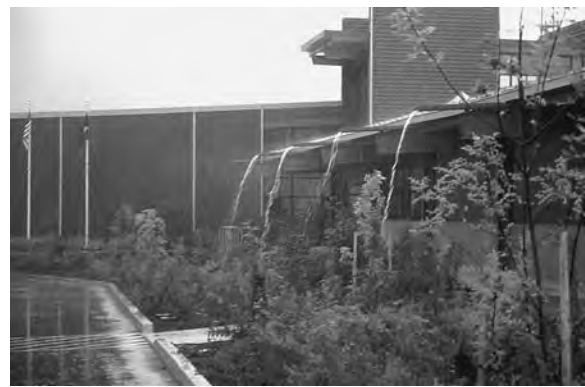
Figure 4.21 Collected on the Portland Water Pollution Control Lab's roof, water spouts from scuppers in rhythmic jets. (Project: Robert Murase. Photo: Tom Liptan.)
