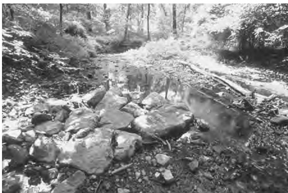
Figure 4.15 Stone deflector in restored Wheaton Branch unobtrusively guards the stream bank from floods. (Project: Washington Council of Governments. Photo: Walt Callahan.)
