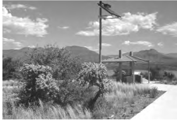
Figure 7.1 Solar electricity for lights and other uses saved hundreds of thousands in utility installation at Cholla Campground, near Phoenix. Operating costs are near zero. (Project: USFS. Photo: Kim Vander Hoek.)
