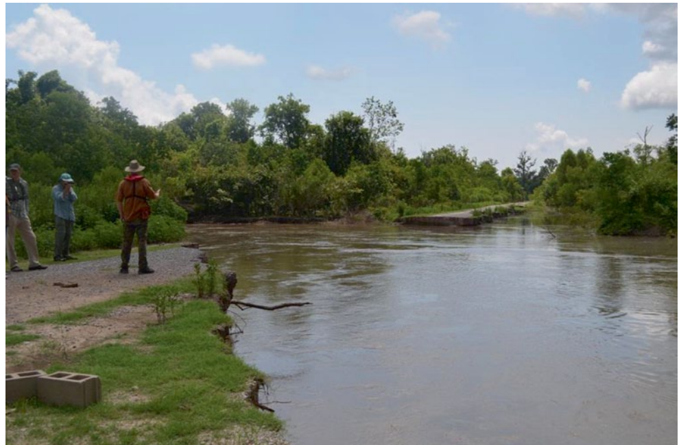
Fig. 28 Mardi Gras Pass crevasse formed on east bank at RK 73 in February 2011 as the river dropped. (Lopez et al. 2013)
