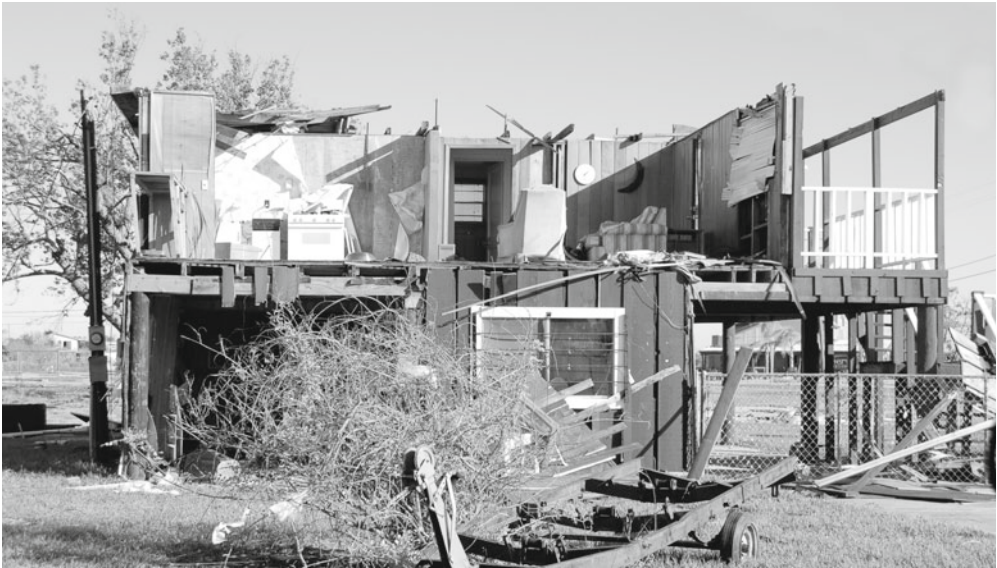
Figure 5.2. Single-family housing destroyed on Galveston Island. (Credit: Shannon Van Zandt, Destroyed Structure , 2008.)
