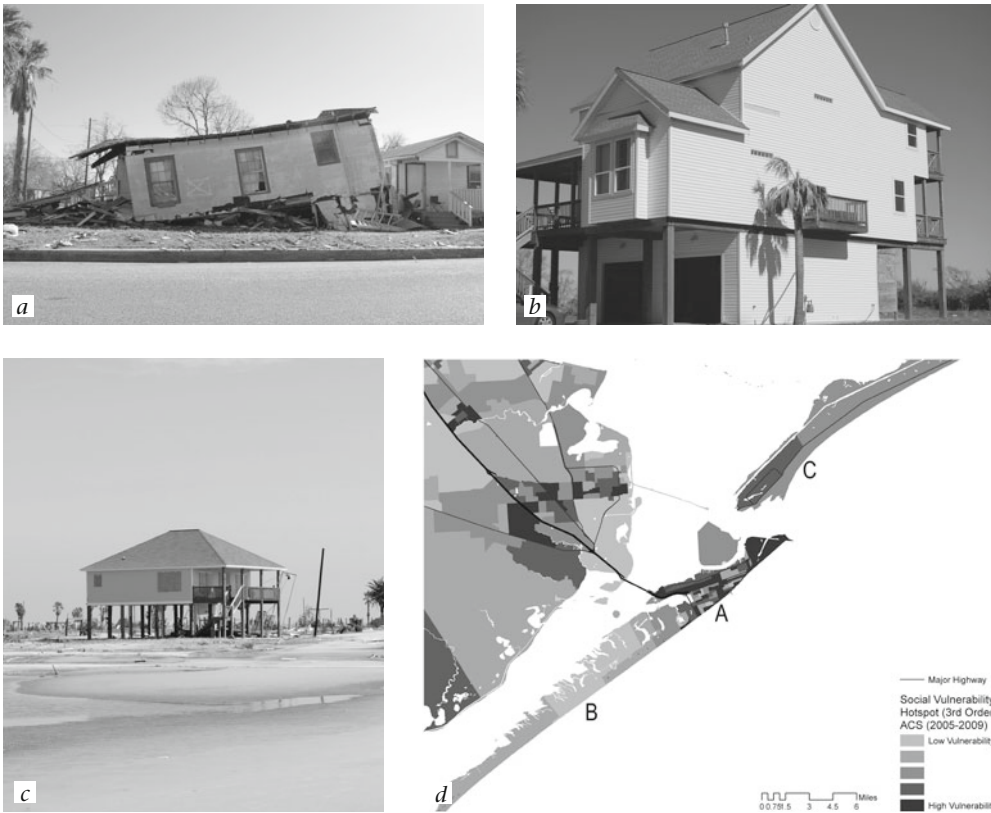
Figure 6.9. (a) In the urban core of Galveston, many lower-quality homes are elevated only a foot or less off the ground, if at all. Here, a poorly constructed home has slid off its foundation, and the other structural systems have also collapsed. (Credit: Shannon Van Zandt, 2008.) (b) In contrast, a West End vacation home sits well above the surge level. A block off the Gulf Coast, these high-quality homes sustained only wind damage, which, as seen here, was minimal. (Credit: Shannon Van Zandt, West End , 2008.) (c) Bolivar Peninsula sustained widespread damage and devastation due to surge waters. Many homes were wiped clean away because they were not built above FEMA base flood elevations. This home is left standing in a neighborhood destroyed by Hurricane Ike. (Credit: Jocelyn Augustino, FEMA, 2008.) (d) Compare the social vulnerability with the damage index in figure 6.8. You can see that many of the least socially vulnerable areas suffered the least amount of damage. The urban core and downtown (a) are particularly socially vulnerable, and so the impacts in this area will be longer lasting, with slow recovery rates.
