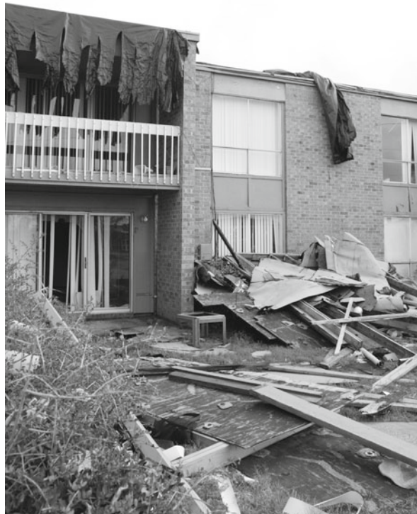
Figure 5.3. Multifamily housing destroyed on Galveston Island. (Credit: W. G. Peacock.)
