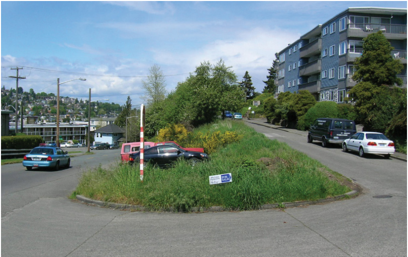
Weeds and overgrown vegetation plague the street medians on Gilman Drive West, Seattle.
