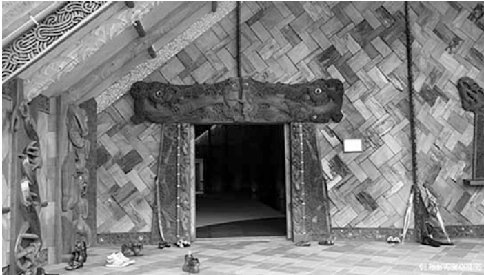
Figure 3.3 The front of Ngakau Mahaki marae is clearly constructed of recycled wooden slats.
