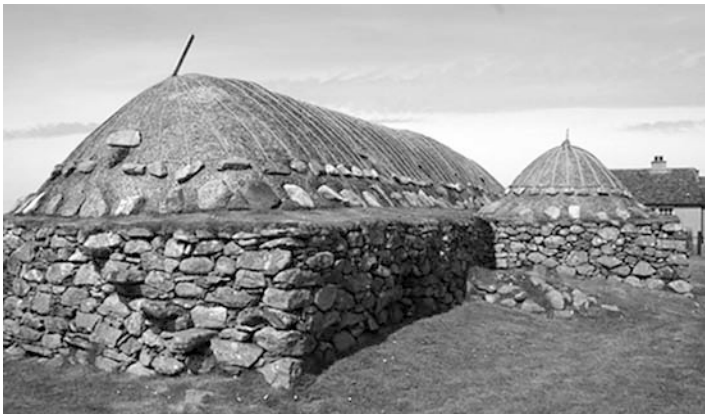
Figure 3.2 The “black house” conserved at Arnol, Isle of Lewis (note the steps built into the wall for easy access to the roof).
