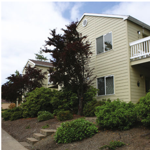
Briar Ridge, Corvallis, OR A planted berm, which provides privacy from the adjacent public street, creates a subtle and attractive transition.
