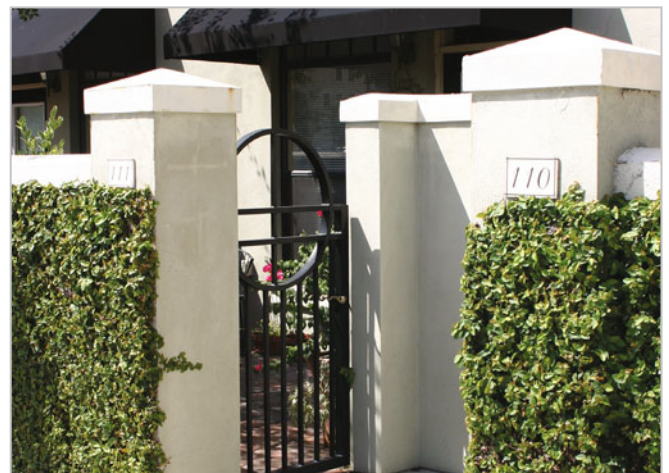
Baldwin Park, Orlando, FL A lowered green wall facing a parking area.
