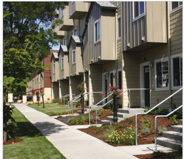
1875 Alder Street, Eugene, OR The front doors to this development open directly onto the street. The stoops and front gardens provide an attractive green edge to the sidewalk and street realm.
