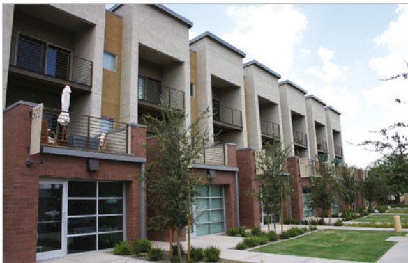
Multifamily units at Town Lake Tempe in Arizona open directly on to the street with front doors and balconies.
