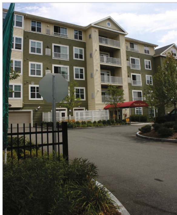
Parkside Crossings, Chelsea, MA An entrance to the site is not gated and other types of safety features are utilized.
