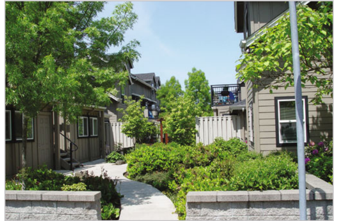
Sheldon Village, Eugene, OR Articulated building façades open on to a vibrant central courtyard among this multifamily housing community.
