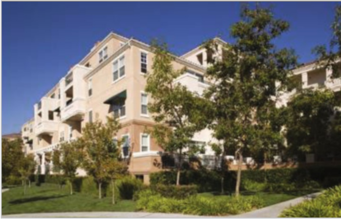
Highly articulated building façades create interest and reduce the feeling of monotonous and repetitious building design.
