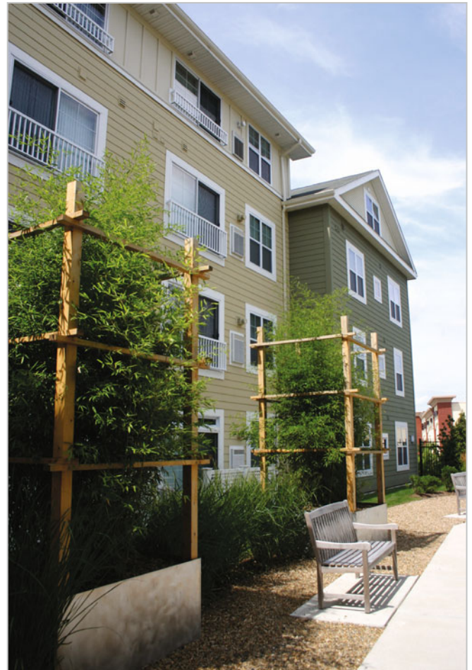
Site features at Parkside Commons in Chelsea, MA include benches, large planters, and fences. These features provide variation and interest for residents.
