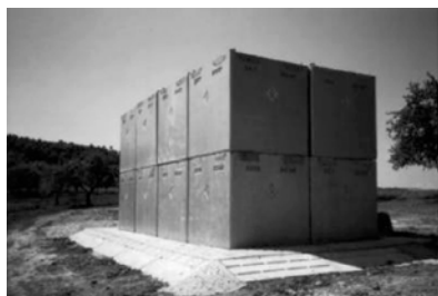
Photo 4. Hermetically sealed steel-concrete containers “BB cubes” for disposal of obsolete and POPs pesticides
