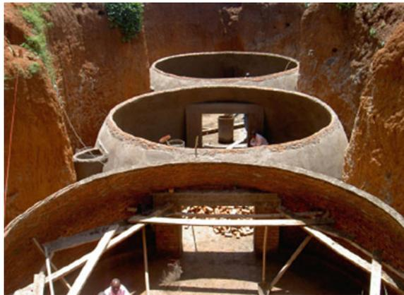
**Fig. 6.3** Internal baffle wall
