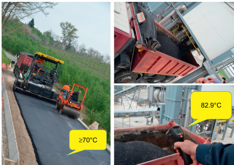
Fig. 14.8 HWMA production using wet sand technology.
