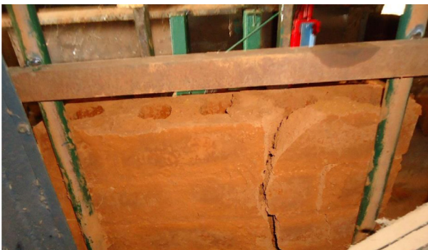
Fig. 13.22 Typical failure pattern (rear view).
