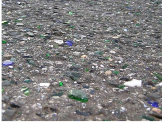
Fig. 5.8 Surface of a road constructed using glassphalt.
