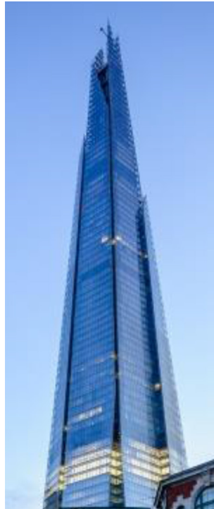
Fig. 5.4 Solar control glass is required in buildings which have large areas of glass façades.
