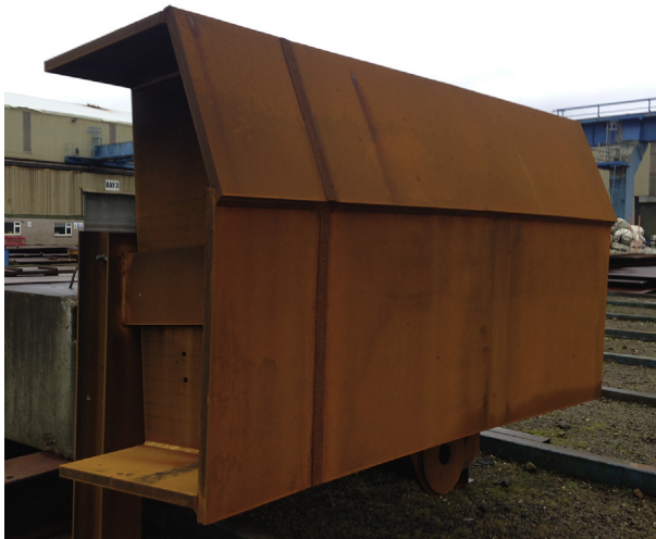
Fig. 6.1 Patina forming on weathering steel.
