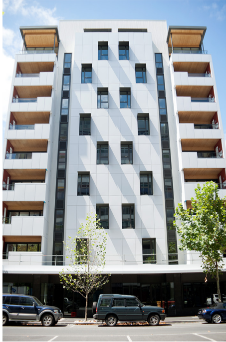
Fig. 8.11 Forté building, Melbourne, Australia. Courtesy Forest & Wood Products Association.
