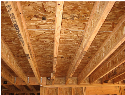
Fig. 8.9 Oriented strand board flooring supported on I-beams with OSB webs. Photograph courtesy APA, Tacoma, USA.
