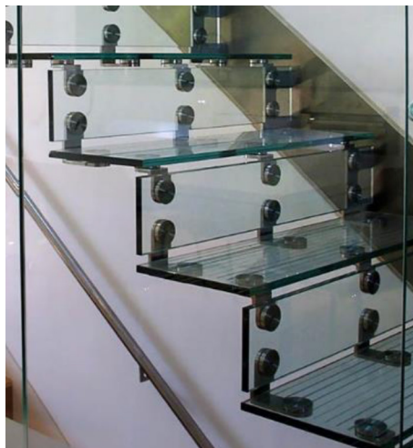
Fig. 5.11 Although bolted joints are widely used, they limit the effectiveness of load-bearing glass structural members.
