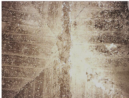
Fig. 10.4 The concrete of the vaulted construction in the Coliseum c.75 AD. Philip L. Owens collection 2003.
