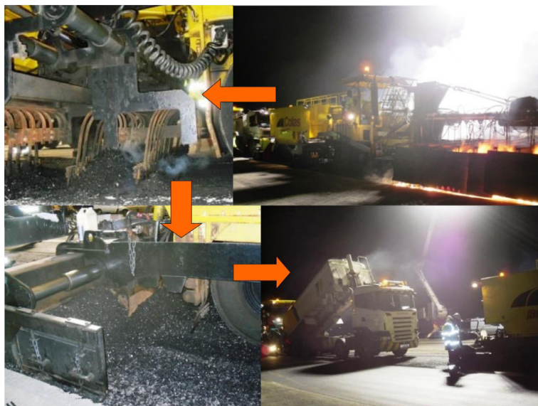
Fig. 14.5 Repave process: heating, scarifying and compaction.
