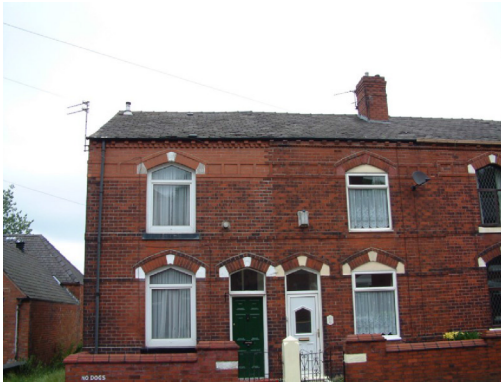
Fig. 11.9 Example of replacement brickwork.
