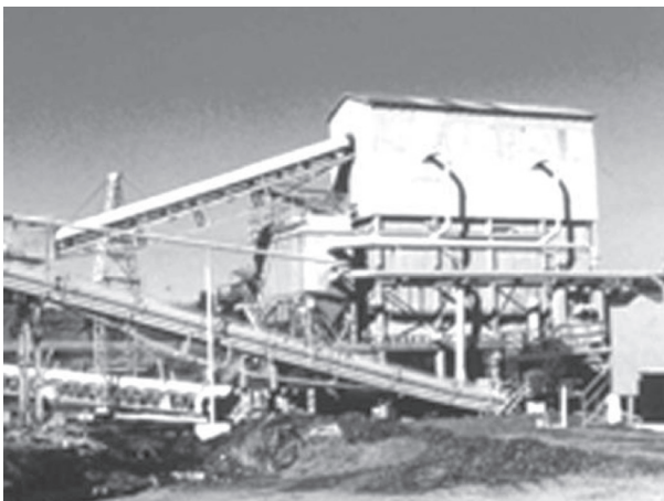
Fig. 9.4 Equipment in sound-deadening, vacuum-equipped enclosure.
