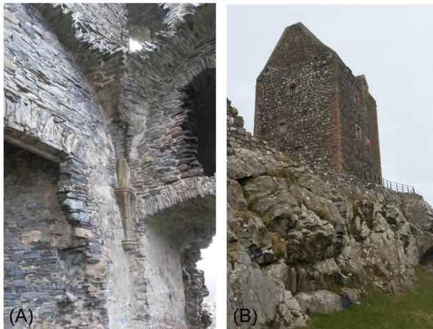
Fig. 12.3 (A) Auchindoun Castle (Scotland, UK): squared rubble walling material with dressed sandstone elements. (B) Smailholm Tower (Scotland, UK): whin walling picked out with sandstone decoration.
