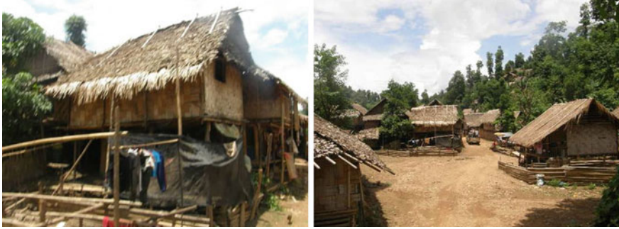
Fig. 4.8 Residential buildings. Source Photo taken by study team
