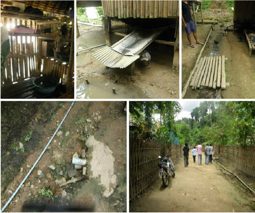
Fig. 4.41 Household water disposal/zinc trough holding wastewater/wastewater channels. Source Photo taken by study team
