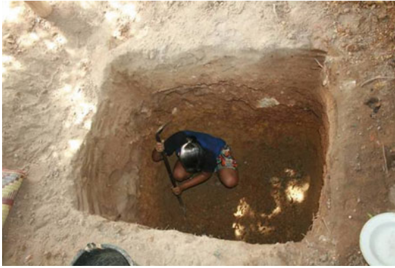
Fig. 4.49 Lavatory with septic tank in the shelter of evacuee. Source Photo taken by study team
