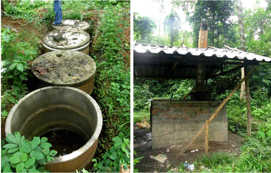
Fig. 4.43 Concrete hole for hazardous waste/incinerator for hazardous waste. Source Photo taken by study team
