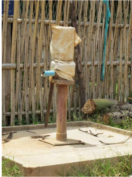
Fig. 4.71 Ground water pump. Source Photo taken by study team
