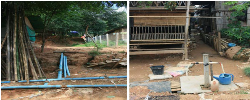
Fig. 4.15 Water distribution inside the temporary settlement. Source Photo taken by study team
