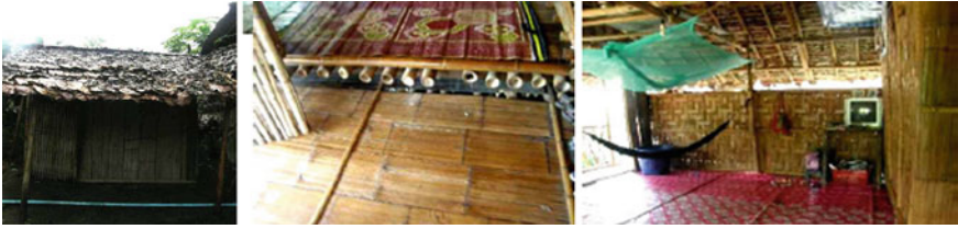
Fig. 4.37 Dried leaf for roofing, and bamboo used for walls, floors and house structure. Source Photo taken by study team
