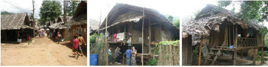
Fig. 4.34 One-storey/two-storey house/two-storey raised floor houses. Source Photo taken by study team
