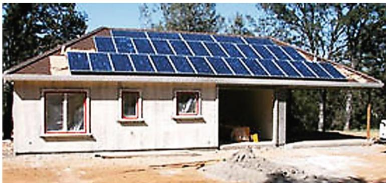
**Fig. 3.24** A 4.4-kW photovoltaic roof installation (<http://www.californiasolarco.com>)
