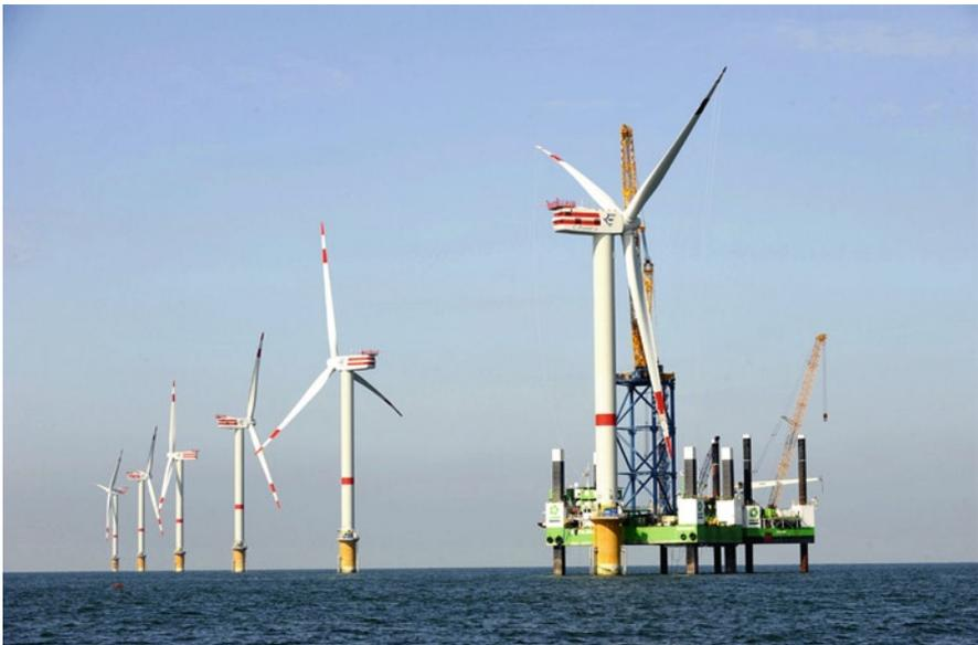
**Fig. 3.9** Erecting an offshore array of REpower's 5-MW turbines (<http://www.repower.de/>)
