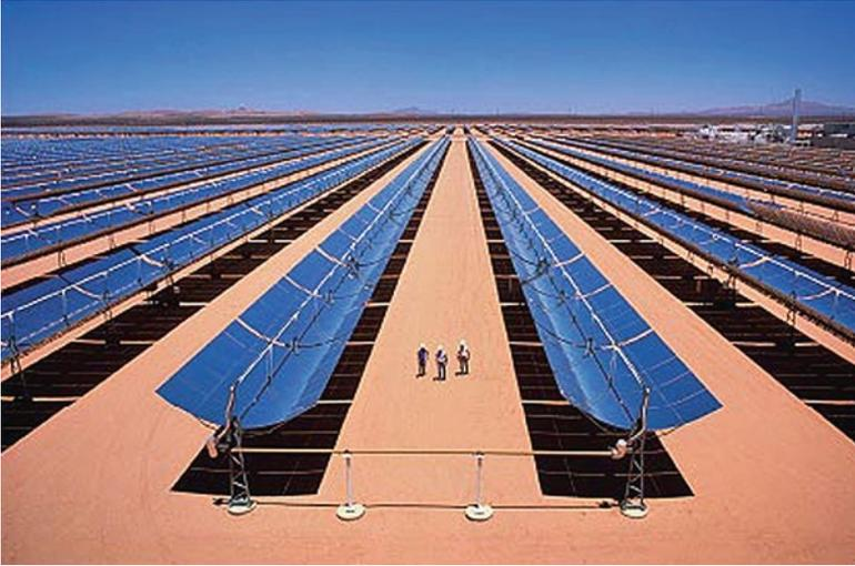
**Fig. 3.26** A parabolic trough system (<http://thoughtsonglobalwarming.blogspot.com/2008/03/solar-thermal-company-says-it-could.html>)
