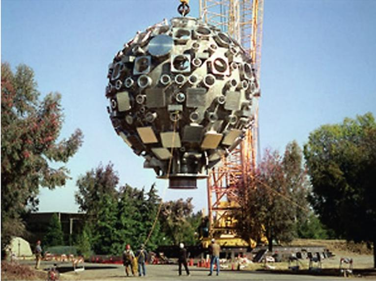
**Fig. 10.51** The NIF target chamber being lifted into the building (<https://www.llnl.gov/str/Atkinson.html>.)
