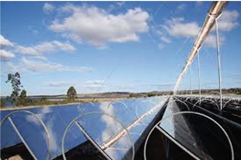
**Fig. 3.27** A linear array of mirrors that rotate to follow the sun ([http://www.instablogsimages.com/images/2007/09/21/ausra-solar-farm\\_5810.jpg](http://www.instablogsimages.com/images/2007/09/21/ausra-solar-farm_5810.jpg))
