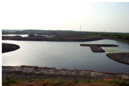
5. Completion of shoal (2009. 05. 06)
