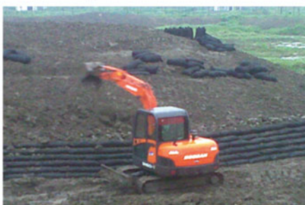
8. Construction of the quick-infiltration ecological system (2009. 06. 26)
