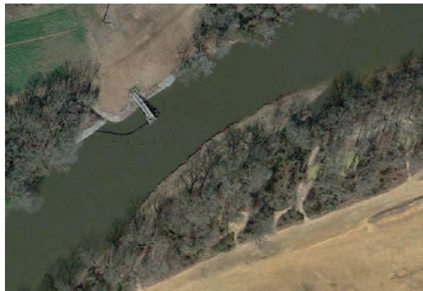
Fig. 3.16 2012 view of Goldsboro raw water intake on Neuse River showing guide wall upstream of intake for smoothing the approach flow to the submerged vane system located off the end of the structure; six buoys are installed outside the vane system to warn boaters. (Source: DitigalGlobe)
