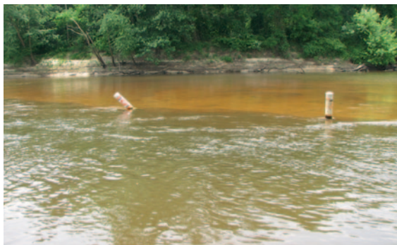
Fig. 3.23 Vane system deflecting bed load around intake screens in Tar River, N.C. (Courtesy of the Greenville Utilities Commission)
