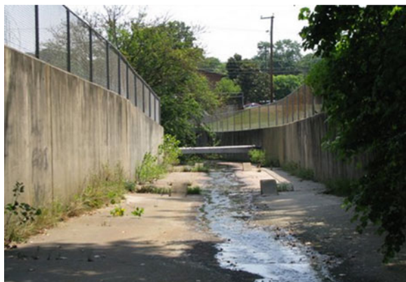
Fig. 7 Reedy Creek, Richmond, Virginia (USA). Impervious surfaces have replaced the natural stream channel and habitat. The channel was designed to remove stormwater from residential, commercial, and industrial land uses (Photo by the first author)
