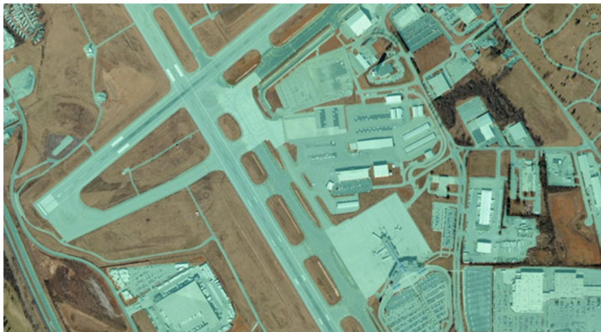
Fig. 5 An example of the photo-overlay technique in GIS, delineating man-made surface cover (cyan polygons) to help identify a transportation land use within an urban area. Completed within GIS using high-resolution (15 cm by 15 cm pixel size) 2008 aerial photos from the Virginia Base Mapping Program. Area location is northwest Roanoke, Virginia, USA; the airport dominates the photo. Source: Image provided by the first author
