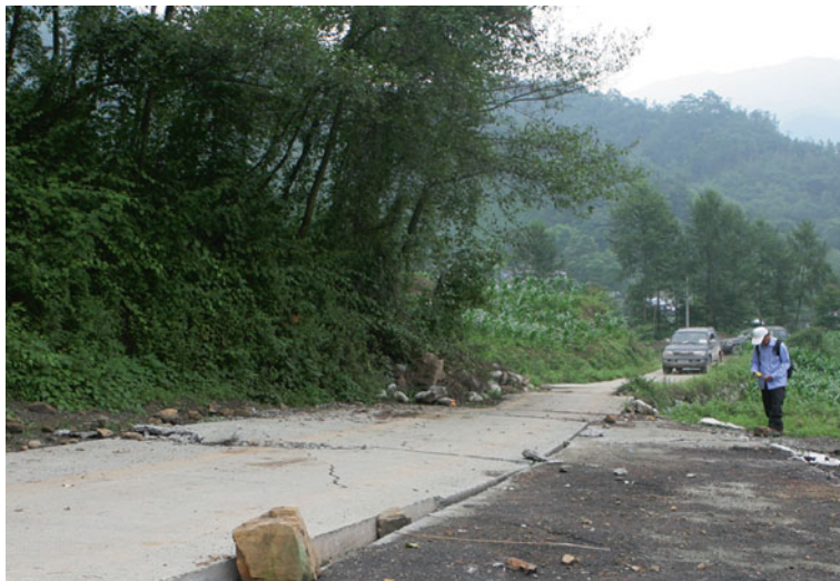
Fig. 4.113 Brittle fracturing of cement pavement on the west of Bailusi gully, Tongji Town, Pengzhou City. The northwest side of the road was uplifted about 1.55 m in total, associated with 30 cm left-slip offset. Viewed to south
