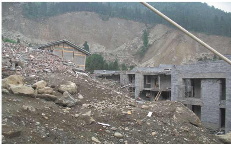
Fig. 4.24 The NW-wall of the foundation of the construction site of the “Chengdu’s impression” buildings at Donglinsi Village, Lommenshan Town, Pengzhou City was uplifted along N40°E direction for 2.5 m with a 2.2 m right-slip offset. Besides, collapse also occurred. Viewed to north
