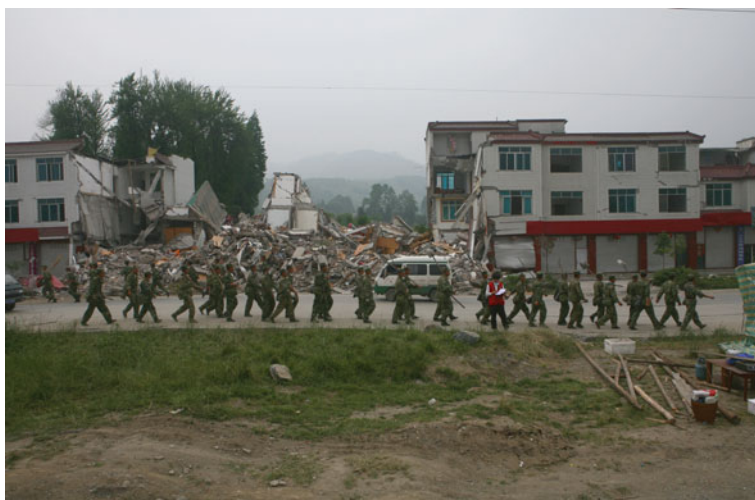
Fig. 4.170 A NW-trending fault-related fold scarp cuts the road in Xiaoyudong Town to form an about 1.09-m-high scarp. The houses on the scarp were completely collapsed. Viewed to northwest
