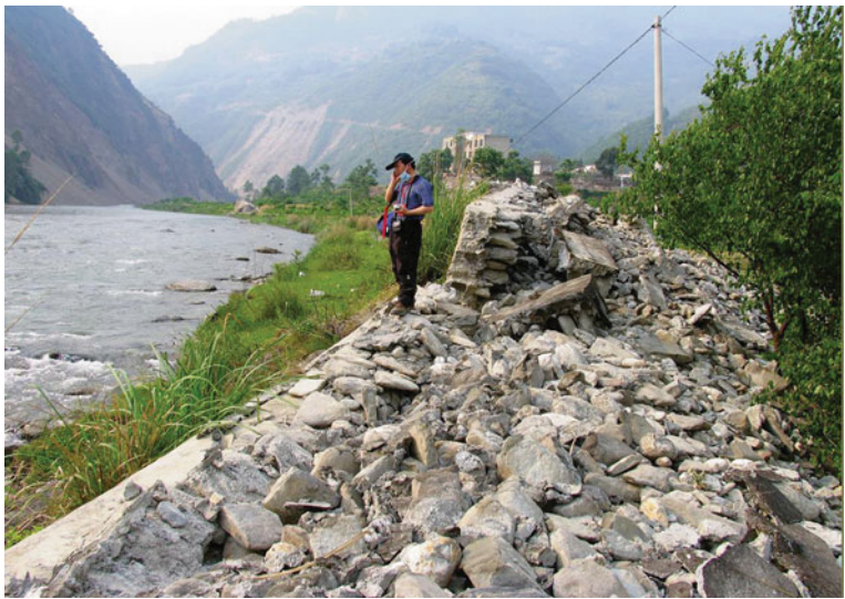
Fig. 4.86 The N50°E-trending fault-related fold scarp in the north of Pingtong Town, Pingwu County obliquely cuts the eastern dykes of the nearly S-N-extending riverbed of the Pingtong River. The scarp is dominated by both vertical offset and right-slip. Viewed to north
