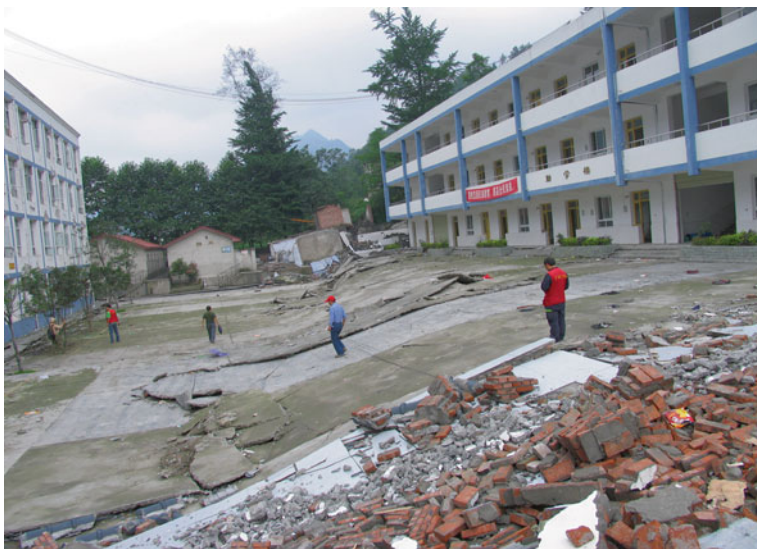
Fig. 4.126 A fault-related fold scarp at the Central School of Bailu Town, Pengzhou City. The scarp is 1.8 m high and strikes N20^{\circ}E . The distance between the scarp and the education building on the northwest side is only 3 m, but the building was undamaged, but the structures and buildings across the scarp in distance and close view were completely collapsed or tilted. Viewed to northwest
