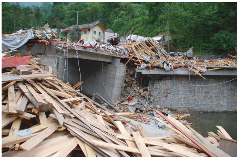
Fig. 4.136 The bridge at Shilong Mountain Villa, Xuanlonggou Village in between the Jinhua and Zundao Towns, Mianzhu City, was obliquely cut by a 1.5-m-high fault-related fold scarp. The bridge seat and its deck were tilted and damaged. Viewed to southwest
