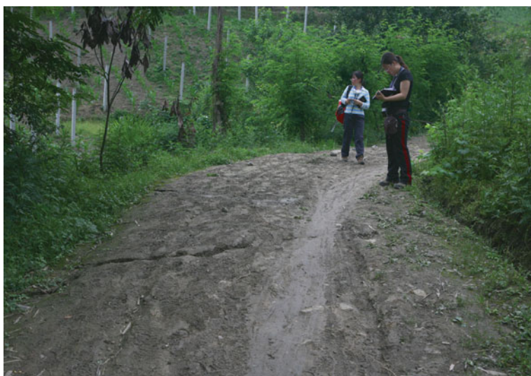
Fig. 4.160 A bent road and tension cracks were formed at the 9th Group of Honghuo Village, Xiang'e Township, Dujiangyan City. Viewed to north
