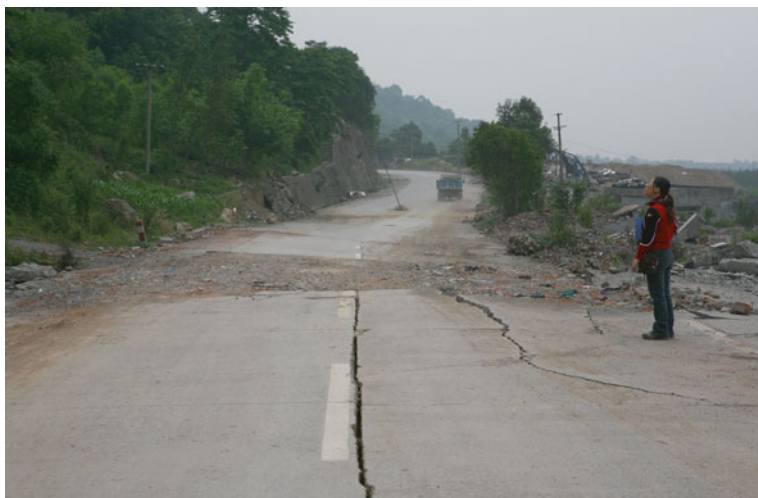
Fig. 4.150 Two imbricated N45^{\circ} – 50^{\circ} E-trending simple pressure ridges occurred on the road from Mianzhu to Maoxian at the eastern bank of the Qingshui River, Hanwang Town, Mianzhu City. The two ridges are 80 m apart and the central line of the road is right-laterally offset 47 cm. Viewed to south
