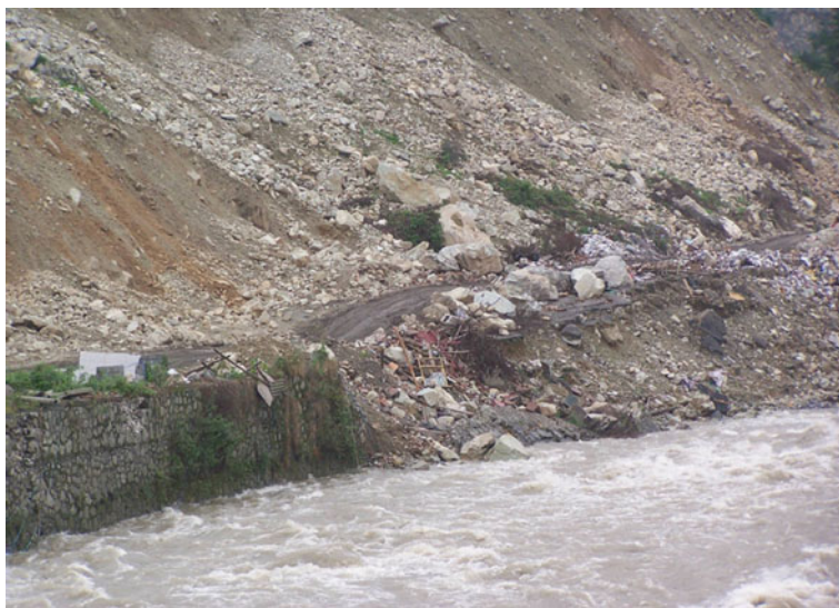
Fig. 4.7 Simple pressure ridge formed along the Yuzixi River and the road on its western bank to the northwest of Yingxiu Town, Wenchuan County. The strong deformation of the hanging wall caused the collapse of the slope and roadbed. Viewed to northwest
