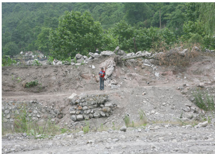
Fig. 4.145 A close-up view of the cross section of the surface rupture zone, which shows shortening of the cement plates of an old road at the western bank of the Qingshui River, Hanwang Town, Mianzhu City. Besides, the embankment was also broken and offset right-laterally about 55 cm. Viewed to west
