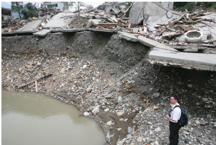
Fig. 4.55 The flexure and fold of the upper gravel deposits and the middle red-brown brick layers of the Jianjiang terrace in the vicinity of the Beichuan Grand Hotel, Qushan Town, Beichuan County. As a result, a 3.1 m-high fault-related fold scarp was formed, causing the brittle fracturing of the cement pavement of the highway, the central line of which was offset right-laterally for 2.4 m. Viewed to NNW
