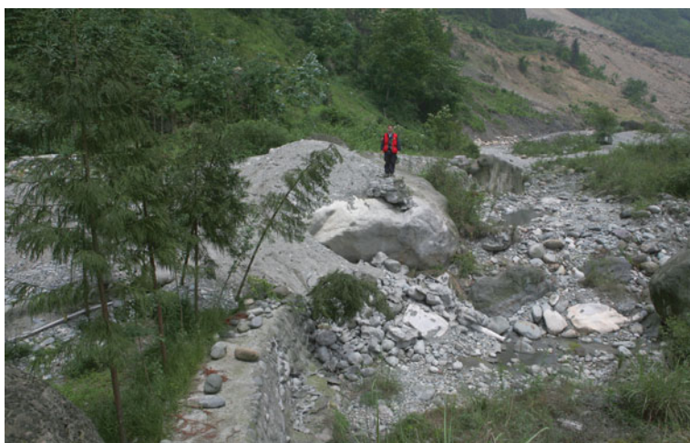
Fig. 4.16 The western embankment of the Baishahe River at Zhoujiaping village, Dujiangyan City, was offset by a dextral pressure ridge. The uplift is 3.1 m and the right-slip displacement is 1.9 m. Viewed to north
