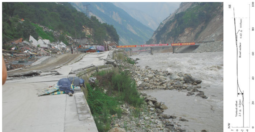
Fig. 4.9 The Minjiang River valley and the road from Dujiangyan to Wenchuan on the T1 terrace on the western bank of the Minjiang River to the north of Yingxiu Town, Wenchuan County were vertically offset to form 2.3 m-high simple pressure ridge. Brittle deformation occurred on the cement pavement of the road. Viewed to north
