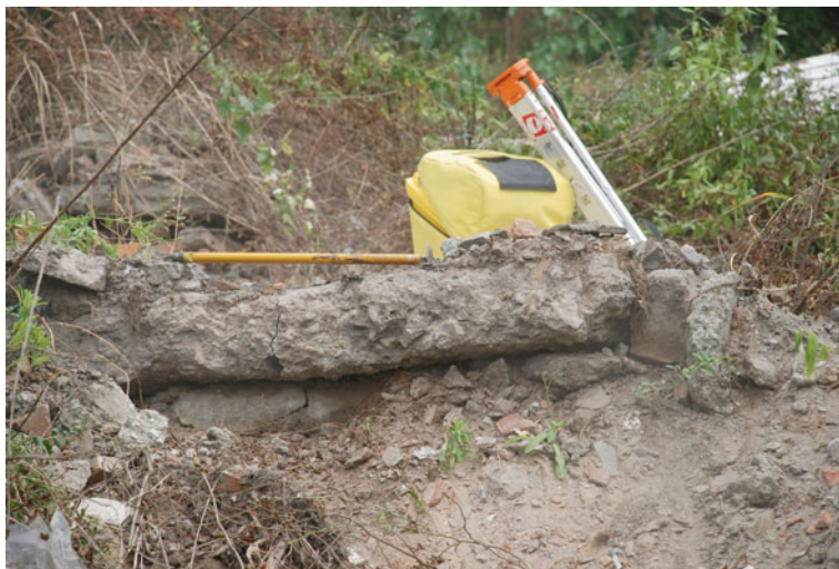
Fig. 4.152 Cement plates were superimposed each other on an abandoned road at the western side of the road from Mianzhu to Maoxian ( 31^{\circ}27'41.6''\text{N} , 104^{\circ}9'59.0''\text{E} ) at the eastern bank of the Qingshui River, Hanwang Town, Mianzhu City. The superimposition amount or the crustal shortening is at least 1.2 \pm 0.1 m. Viewed to east
