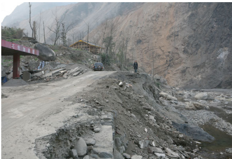
Fig. 4.103 The road near the Shikan Petrol Station at Shikan Township, Pingwu County was not only warped and folded, but its embankment was right-laterally offset about 2.4 m. Viewed to north
