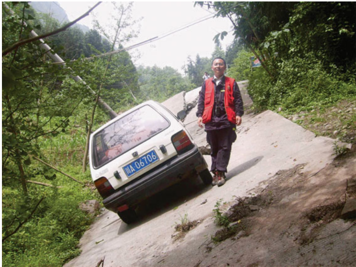
Fig. 4.11 The fault-related fold scarp has caused the SE-tilting of the cement pavement of a road at Shenxigou, Hongkou Town, Dujiangyan City. The dip angle may reach up to 35^{\circ}\sim 40^{\circ} , and the car on the road inclined with the inclination of the ground. Viewed to southwest
