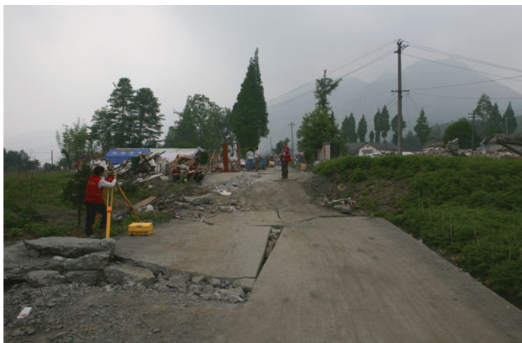
Fig. 4.169 A 1.47-m-high and NW-trending sinistral pressure ridge on a road to the north of Xiaoyudong Town. The left-slip offset is 2.3 m, and the cement pavement of the road near the scarp was broken. Viewed to southwest
