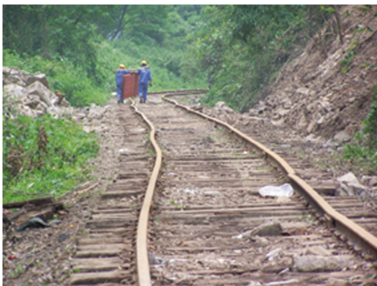
Fig. 5.31 Flexural deformation of the rails of the Muguaping Phosphorus Mine railway, Shifang City. Viewed to north
