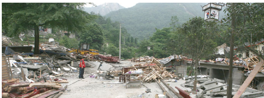
Fig. 4.139 Fault-related fold scarp at Shilong Mountain Villa, Xuanlonggou Village in between the Jinhua and Zundao Towns, Mianzhu City. The scarp is about 1.5 m high, the houses and bridge near the scarp were damaged. The bridge deck was tilted and brittle rupture occurred on the cement road. Viewed to north
