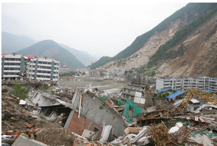
Fig. 5.19 The impact wave of the front of Wangjiayan landslide had caused the collapse of houses into ruins (close view) at Qushan Town, Beichuan County. The collapse of mountain had also caused the collapse of newly built Beichuan Middle School and the adjacent houses (in distance). Viewed to north
