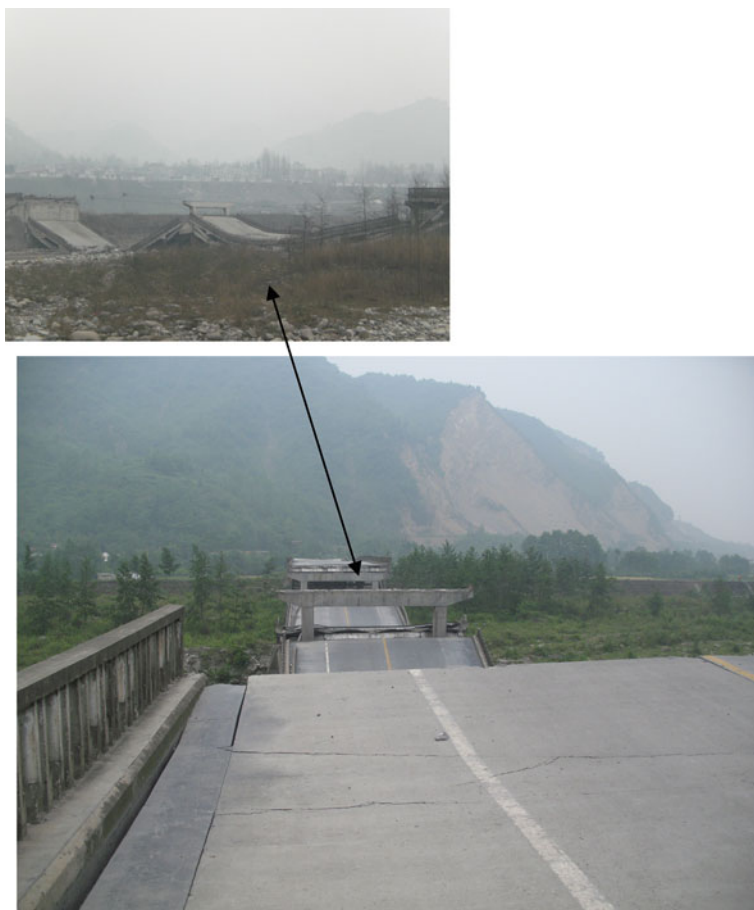
Fig. 5.27 The Xiaoyudong surface rupture zone obliquely cuts the river valley of the Baishuihe River and the eastern seat of the Xiaoyudong Bridge. The bridge on the hanging wall was displaced into several sections. Viewed to west
