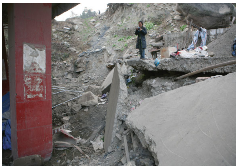
Fig. 4.102 A scarp vertically offset the cement pavement of the Shikan Petrol Station about 3 m at Shikan Township, Pingwu County; the broken cement plates near the scarp are nearly vertical. Viewed to southwest
