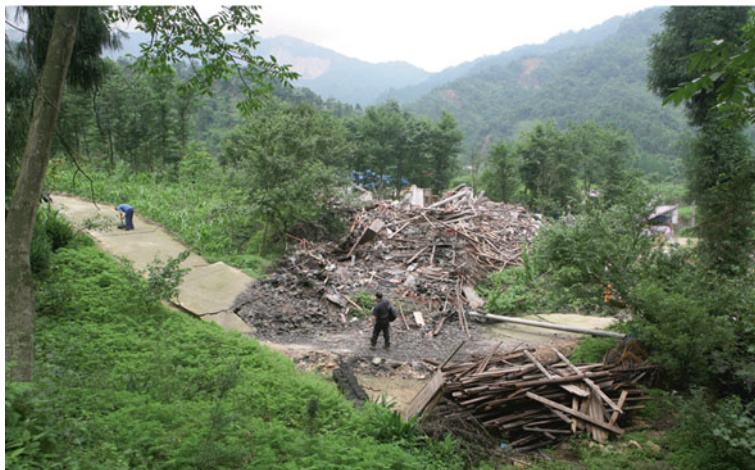
Fig. 4.120 A 2.2-m-high fault-related fold scarp cuts obliquely the cement road and peasant's houses and wire poles were completely collapsed at Wangjiaba Village, Bailu Town, Pengzhou City. The rupture zone on cement road is 21 m wide. Viewed to northeast
