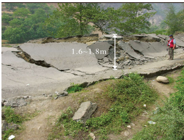
Fig. 4.99 The province highway No. 105 was vertically offset 1.6–1.8 m at a site about 1 km to the south of Shikan Township, Pingwu County. Viewed to NNE
