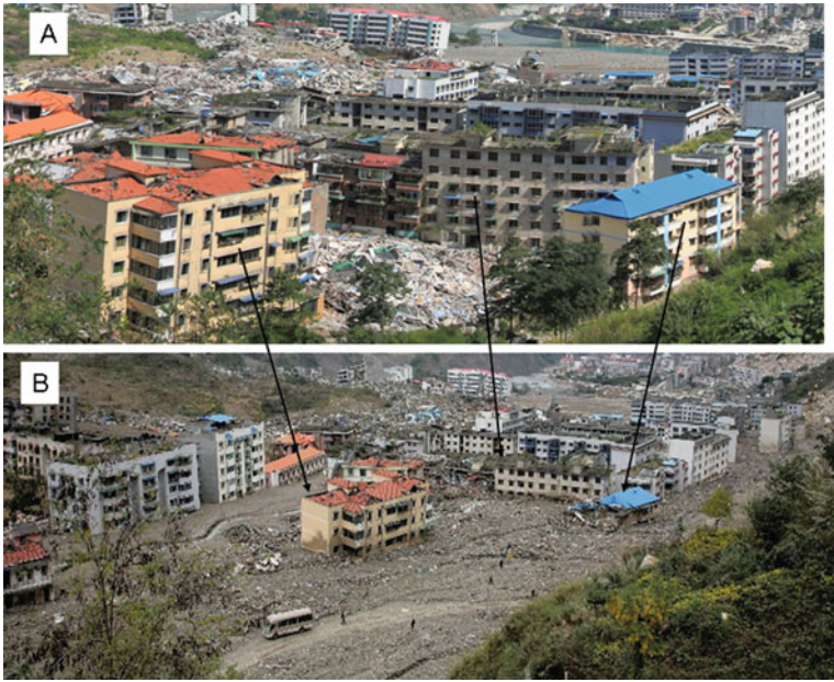
Fig. 5.23 The concrete buildings far from the fault zone in the center of Qushan town were survived during the Wenchuan earthquake (a), but buried by the later storm induced muddy flow (b)
