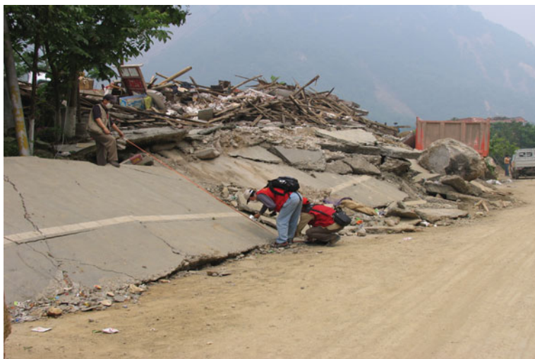
Fig. 4.53 The Anxian to Beichuan highway was offset by the earthquake fault to form a N20°E-trending about 3 m-high fault-related fold scarp higher in the west and lower in the east, at Renjiaping Village, 1 km to the south of the Beichuan County. Viewed to north
