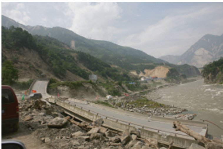
Fig. 5.30 The entire length of Dujiangyan-Yingxiu-Wenchuan express way along the bank of the Minjiang River was broken. Viewed to north
