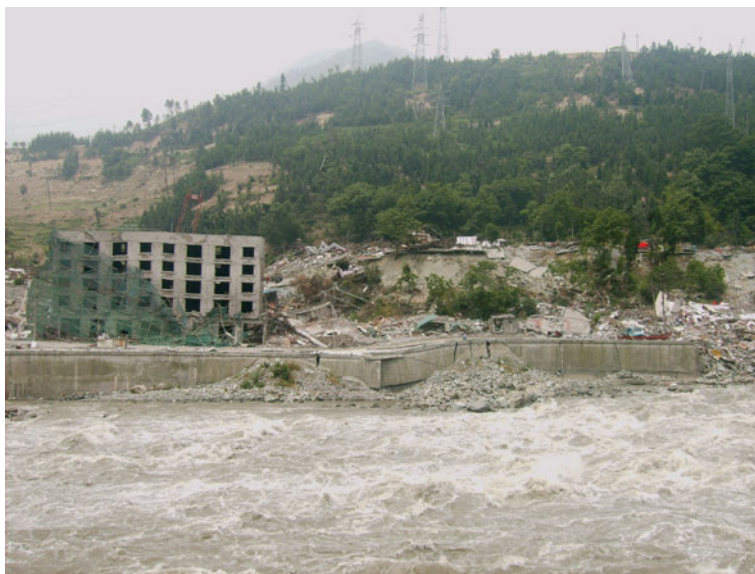
Fig. 4.8 The Beichuan fault co-seismically offset the Minjiang River valley and its multiple levels of terraces, resulting in simple pressure ridge and waterfall scarp. Near surface tension cracks occurred on the hanging wall of the scarp, and the residential buildings on the surface rupture zone were completely destroyed; a 6-storey building under construction on the foot-wall of the zone near the fault was damaged in its structures and the second floor was missed. Viewed to west
