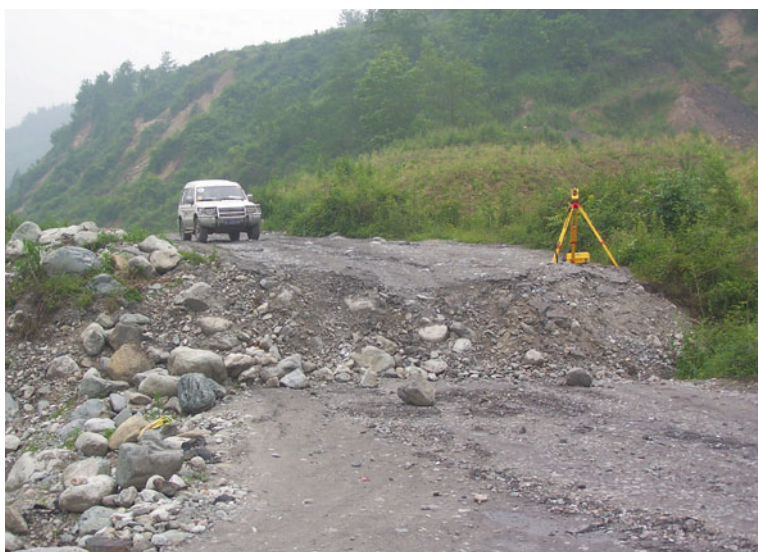
Fig. 4.176 A hanging-wall collapsed fault scarp on a road of the floodplain, eastern bank of a river to the northeast of Luoyang Village, Xiaoyudong Town. The scarp is NEE-striking and about 3.4 m high. Viewed to north
