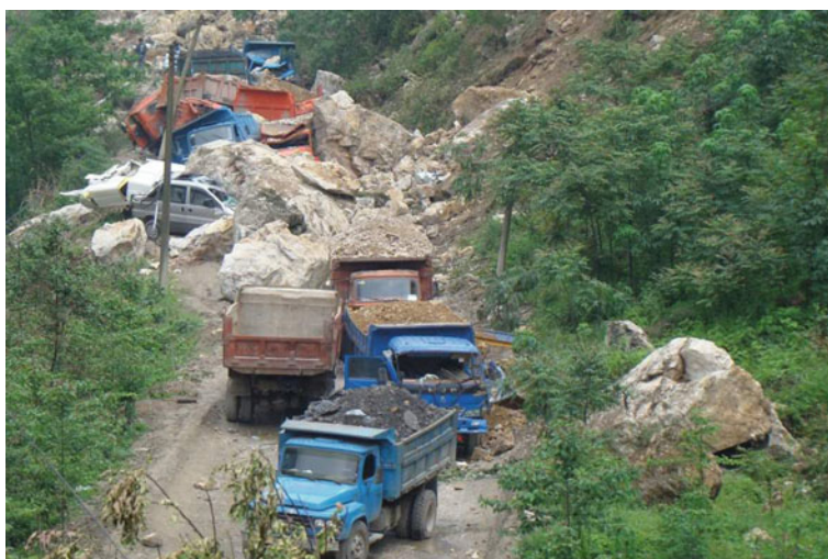
Fig. 5.33 The fallen rocks damaged the vehicles and blocked the Gaochuan road in Anxian County
