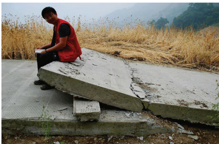
Fig. 4.90 Crocodile-mouth-like scarp at Pingtung Town, Pingwu County; the cement pavement of the road bulged and superposed; the superposition segment is 50–60 cm long. Viewed to northeast
