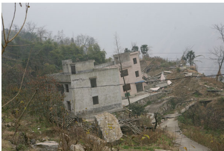
Fig. 5.41 The houses located on a normal fault scarp at Maoba Village, north of Qushan Town, Beichuan County, were collapsed (the scarp on the right side is about 5 m high). Two buildings on the hanging wall were tilted, and the tilting degree decreases with the increasing distance from the scarp. Viewed to southwest
