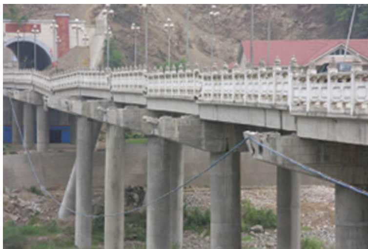
Fig. 5.29 Beichuan Bridge plate was shifted northeastward, whereas the bridge pillars were not displaced (view to NW)
