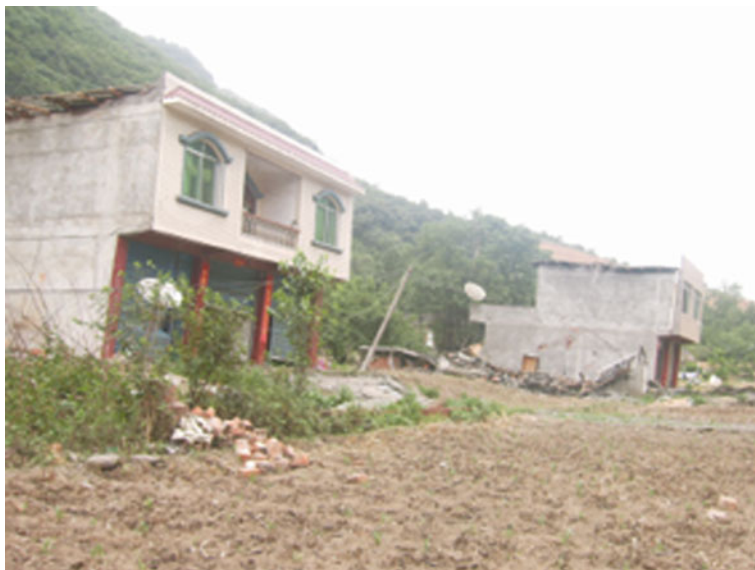
Fig. 5.42 A storied building located across an earthquake scarp (the building in distance) at Lizikan Village, Pingwu County, was structurally damaged and tilted, and the storied building on the hanging wall was tilted. Viewed to north
