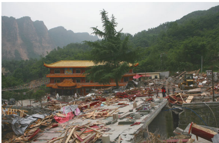
Fig. 4.135 The deck of a bridge and a single tree trunk on a 1.5-m-high fault-related fold scarp at Shilong Mountain Villa, Xuanlonggou Village in between the Jinhua and Zundao Towns, Mianzhu City were tilted southeastward. The bridge seat was cracked, the houses on the scarp and its hanging wall were collapsed, and the damages of villa buildings on the footwall are slighter. Viewed to southwest
