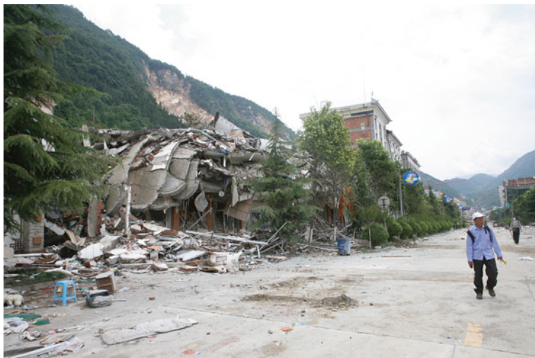
Fig. 5.20 A six-storey building in the north of Qushan Town, Beichuan County, remained only the first floor after the earthquake, while the above stories had been superimposed to make up a “sandwich structure”. Viewed to east
