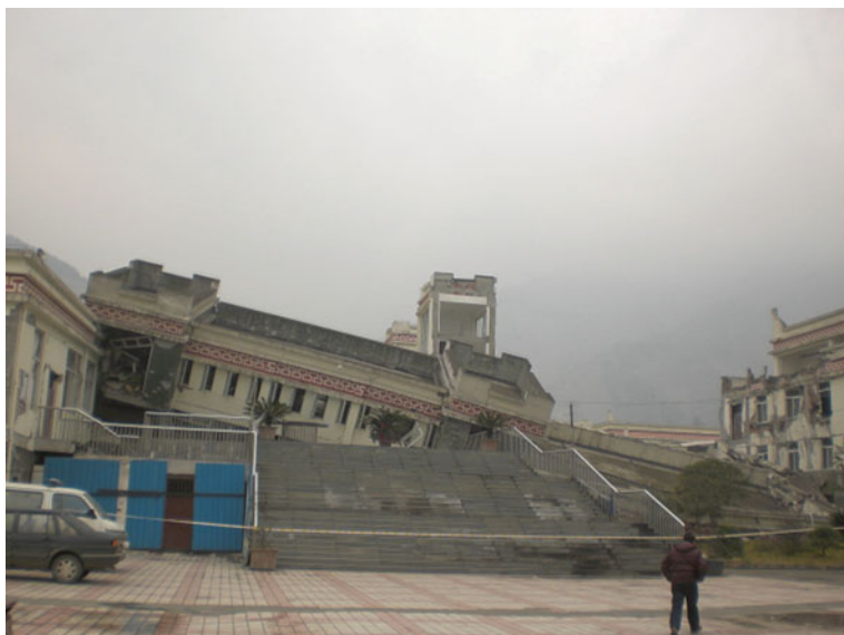
Fig. 5.12 The main teaching building of Yingxiu Middle School at Yingxiu Town, Wenchuan County, was collapsed by the earthquake. Viewed to north
