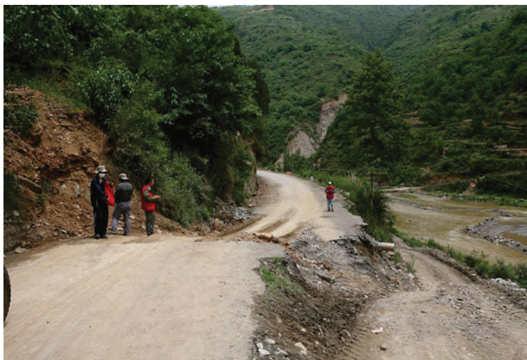
Fig. 4.93 Earthquake surface rupture zone at a site to the northeast of Nanba Town, Pingwu County. The rupture zone is N45^{\circ}\text{--}50^{\circ}\text{E} -striking; the northwest side of the road was uplifted 1.52 m and right-laterally offset 2.5\pm0.2 m. Viewed to southeast
