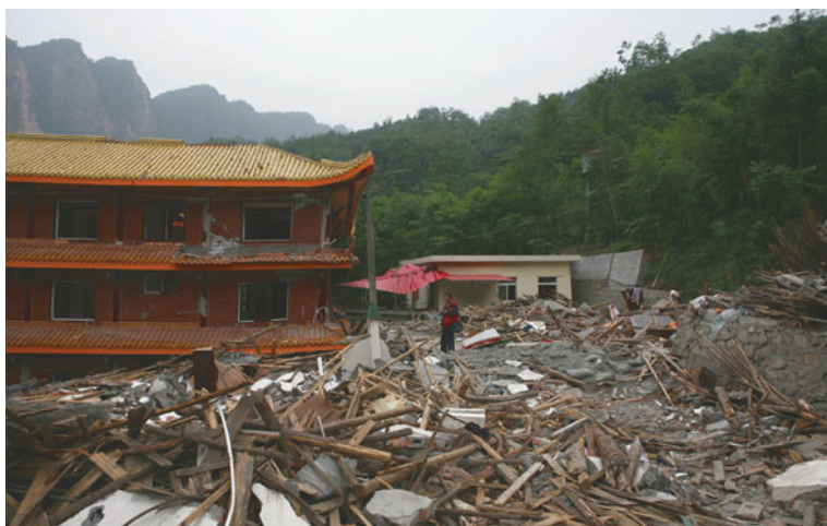
Fig. 4.137 The villa's buildings on the footwall near the scarp were cracked and warped and the milky white house on the scarp was tilted at Shilong Mountain Villa, Xuanlonggou Village in between the Jinhua and Zundao Towns, Mianzhu City, Viewed to southwest
