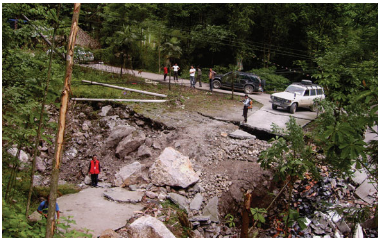
Fig. 4.13 Fault-crossing cement road was offset by the hanging-wall collapse scarp at Shenxigou, Hongkou Town, Dujiangyan City, displaying a right-slip offset of 4.5 m and vertical offset of 2.7 m. Viewed to northwest
