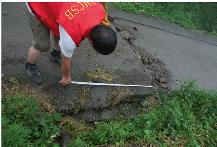
Fig. 4.133 A close-up view of about 1.2 m superimposition of cement plates north of Yinghua Town, Shifang City. Viewed to northwest
