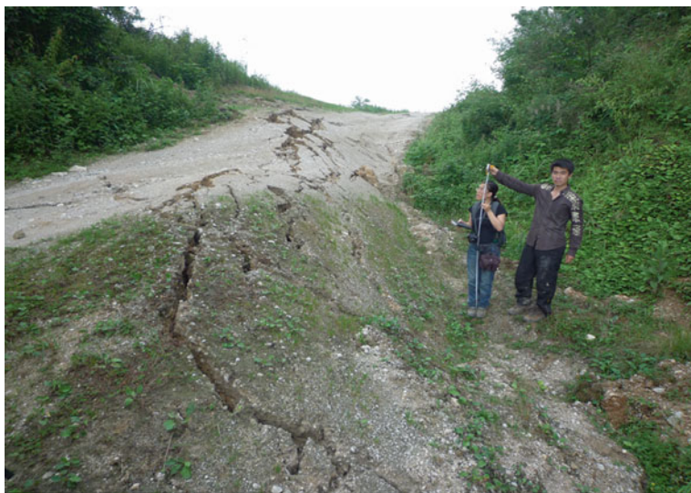
Fig. 4.131 A 1.7-m-high simple pressure ridge obliquely cutting a road at a big col between the Bailu and Bajiao Towns. Viewed to northeast
