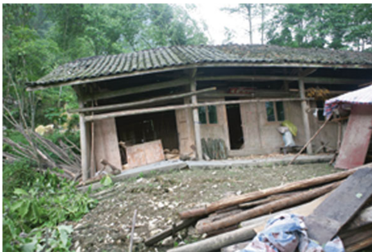
Fig. 5.43 A wood framework structured house at Shenxigou Village, Hongkou Township, Dujiangyan City, was tilted with the declination of fault scarp, and the upper wall was slightly tilted with the tilting of the ground. Viewed to west
