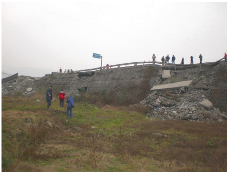
Fig. 4.165 The Xiaoyudong surface rupture zone obliquely cuts the river valley of the Baishuihe River and the eastern seat of the Xiaoyudong Bridge. The bridge on hanging wall was broken into several sections. Viewed to north
