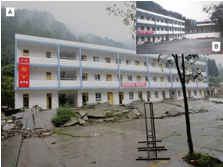
Fig. 5.45 The teaching building of the Bailu School in Pengxian County on the hanging wall of the scarp was relatively intact after the earthquake (a) with comparison of that before earthquake (b)
