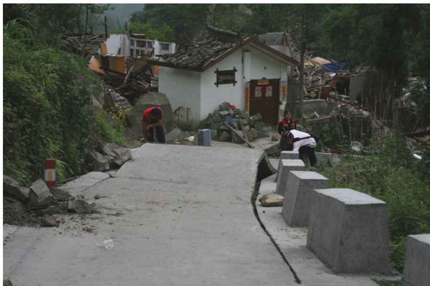
Fig. 4.138 Brittle rupture occurred on the cement pavement of a road on the hanging wall (away from the scarp) to form a tent-like pressure ridge and the houses nearby were damaged, north of Shilong Mountain Villa, Xuanlonggou Village in between the Jinhua and Zundao Towns, Mianzhu City. Viewed to south
