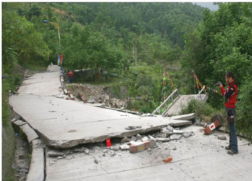
Fig. 4.140 A 2.0 m-high fault-related fold scarp (in distance) and a pavement suprarhrust scarp in front were developed on a cement road at Longquan Moutain Villa, Qingquan Village, Jiulong Town, Mianzhu City. The scarp is N25°E-trending. The cement plates were superimposed. Its superimposition amount on the hanging wall is about 1.5 m, and that on the footwall is 1.3 m, which shows a total shortening amount of about 2.8 m. Viewed to north
