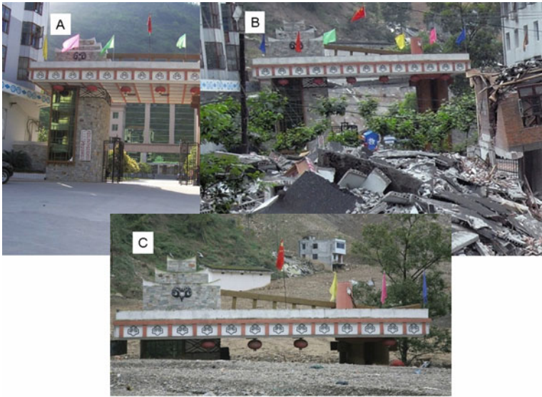
Fig. 5.22 Photographs of the outdoor gate of the Beichuan government taken at different time: (a) before the earthquake; (b) just after the earthquake but before the heavy storm in June 2008 and (c) after the storm, the gate was almost buried by the muddy flow
