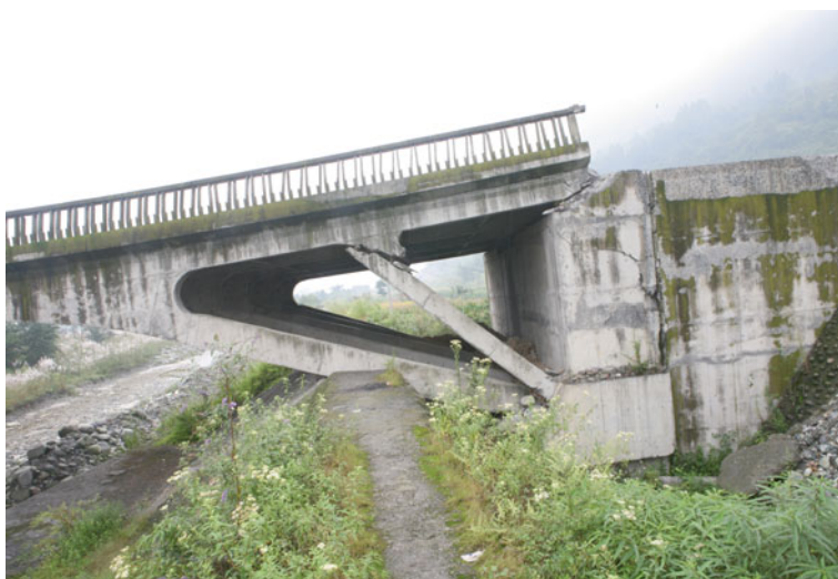
Fig. 4.166 The Xiaoyudong surface rupture zone obliquely cuts the eastern seat of the Xiaoyudong Bridge, causing fracturing of the oblique beam and the bending of the reinforced bars of the bridge. Viewed to north
