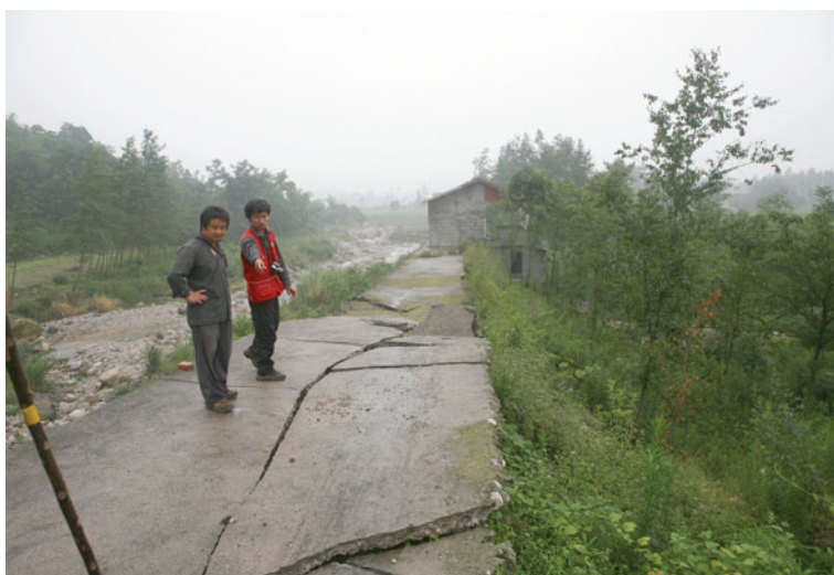
Fig. 4.153 Broken cement pavement and about 1-m-high fault-related fold scarp on the western dyke of the river at Quanxin Village, east of Hanwang Town, Mianzhu City. The sideline of the dyke shows that no horizontal offset occurred. Viewed to northeast
