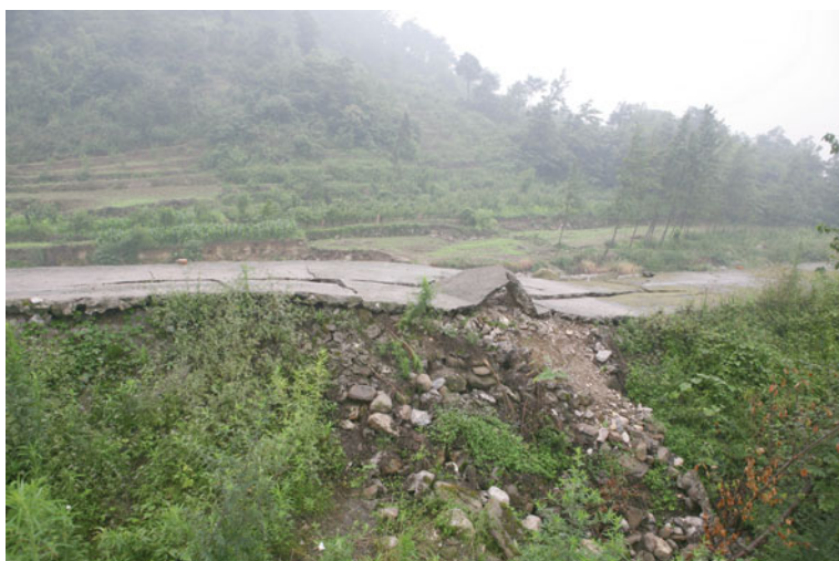
Fig. 4.151 The cement plates of western dyke of the river at Quanxin Village east of Hanwang Town, Mianzhu City, are fractured to form tent-like structure superimposed on the fault-related fold scarp. Viewed to northeast
