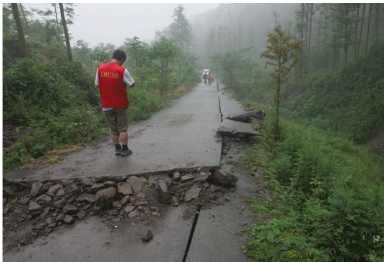
Fig. 4.132 Two sub-parallel brittle breaks occurred on cement pavement of a road and the cement plates were superimposed north of Yinghua Town, Shifang City. The amount of superimposition of cement plates in close view is 1.2 m, and at the site the people standing in front of a car in distance is 0.72 m, indicating crustal shortening of at least 1.9 m. Viewed to northwest
