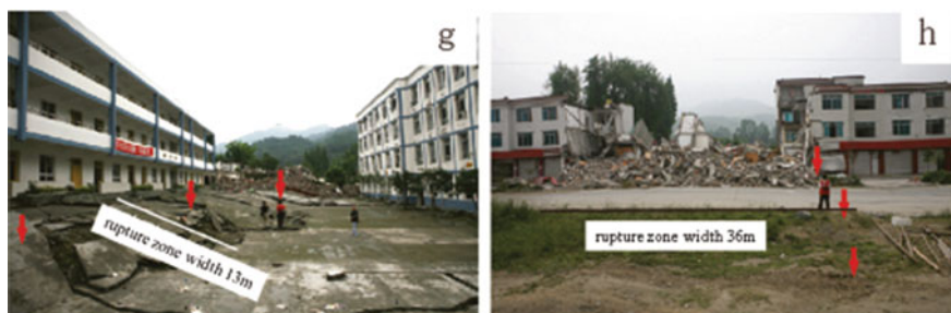
Fig. 5.40 (continued) northwest; (g) Simple pressure ridge on the Hanwang-Bailu surface rupture zone at Bailu Middle School, Pengxian County; the teaching building on the footwall of the scarp was fractured but not collapsed, and the building on the hanging wall was relatively intact; the scarp is N50°E-trending, and the width of the surface rupture zone is 13 m; viewed to northeast; and (h) The width of the simple thrust fault scarp and the collapsed buildings on the NE-trending Xiaoyudong surface rupture zone on the south street in Xiaoyudong Town; the width of the surface rupture zone is 36 m; viewed to northwest
