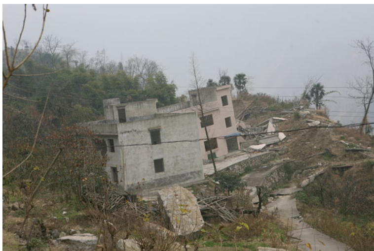
Fig. 5.21 The houses located on a normal fault scarp at Maoba Village, north of Qushan Town, Beichuan County, were collapsed (the scarp on the right side is about 5 m high); two buildings on the hanging wall were tilted, and the tilting degree decreases with the increasing distance from the scarp. Viewed to southwest
