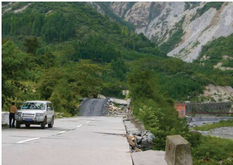
Fig. 4.31 A 3.8 m-high scarp with a right-slip offset of 1.5 m on the highway from Mianzhu to Maoxian at Qingping Village, Mianzhu City. On the background there is a swarm of landslides. Viewed to north
