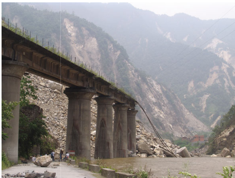
Fig. 5.26 Slope collapse and fracturing of railway bridge at Muguaping Phosphorus Mine, Pengzhou City. Viewed to north
