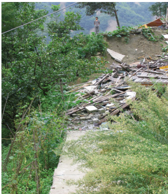
Fig. 4.65 The cement road was offset right-laterally 3.3 m and vertically 6 m at Shaba Village to north of Beichuan County. Viewed to northwest
