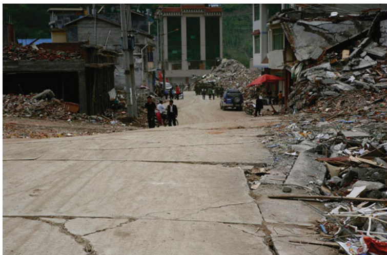
Fig. 4.89 The northwest wall of the road to Pingwu County town on the T2 terrace at Pingtung Town, Pingwu County was uplifted about 2.5 m relative to its southeast wall at Pingtung Town, Pingwu County; the road was offset right-laterally for 1.5 m, and the broken road pavement indicates that the width of the surface rupture zone is 41 m. Viewed south
