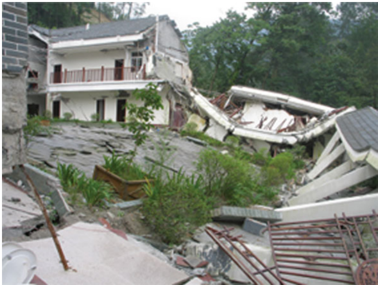
Fig. 5.44 The Bajiaomiao Sanatorium at Hongkou Twonship, Dujiangyan City, located on the fault scarp was collapsed, but the part on the hanging wall was fractured and relatively intact. Viewed to northeast
