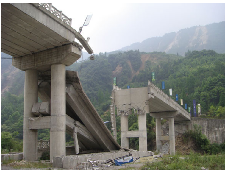
Fig. 5.25 The middle part of a bridge near Gaoyuan Village, Hongkou Township, Dujiangyan City was broken down. Viewed to northwest by north
