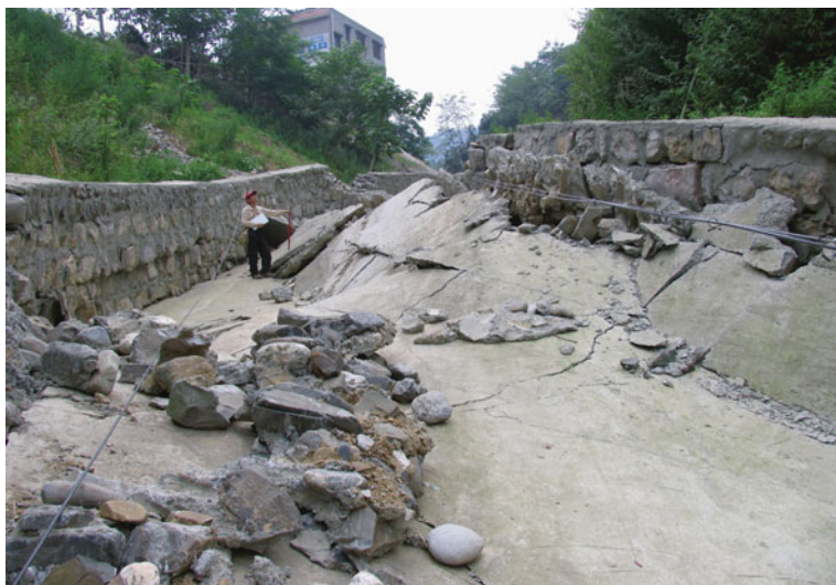
Fig. 4.54 The folded and broken man-made canal showing uplift of the northwest side and the warping of the cement bottom of the canal in the south of Qushan Town, Beichuan County. Viewed to north
