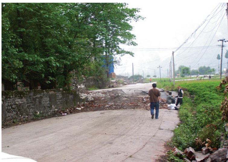
Fig. 4.168 The sinistral pressure ridge cutting through the enclosing walls, road and cropland at the Jianjiang Chemical Plant. The vertical offset was measured to be 1.2 m with a left-slip component. Viewed to southwest
