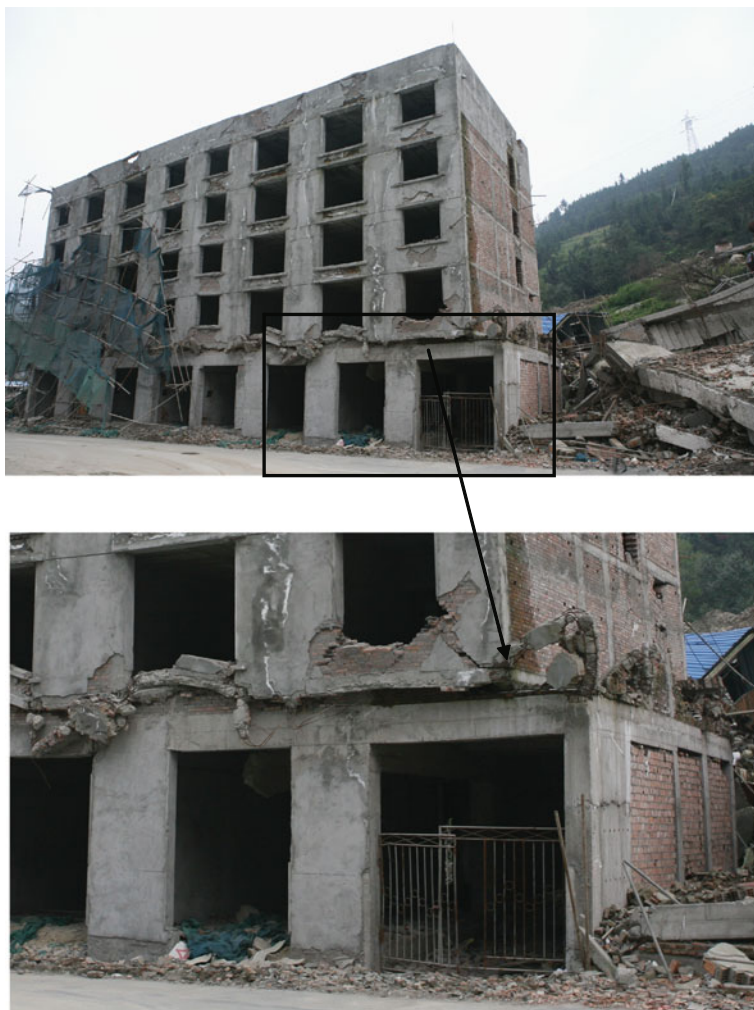
Fig. 5.11 The second storey of a six-storey building in construction on the footwall was lost after the earthquake. Viewed to west
