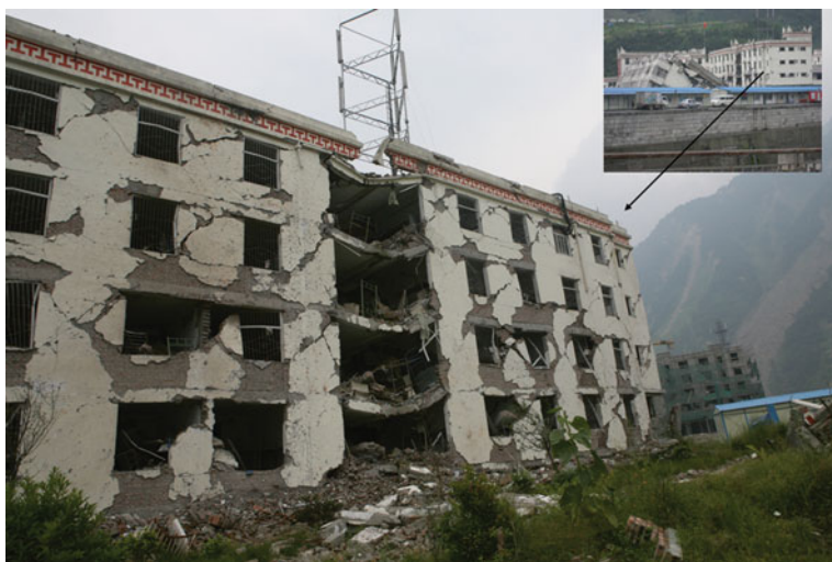
Fig. 5.13 The dormitory building of the Yingxiu middle school at Yingxiu Town, Wenchuan County, was damaged by X-shaped shearing cracks, and the first floor was lost after the earthquake. Viewed to north
