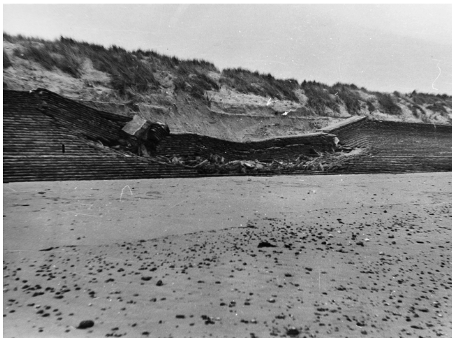
Fig. 14.3a The retaining sea wall at Horsey in Norfolk, taken on 4th February 1953 soon after the 31st Jan/1st February storm surge (Image courtesy of Norfolk County Council Library and Information Service)
