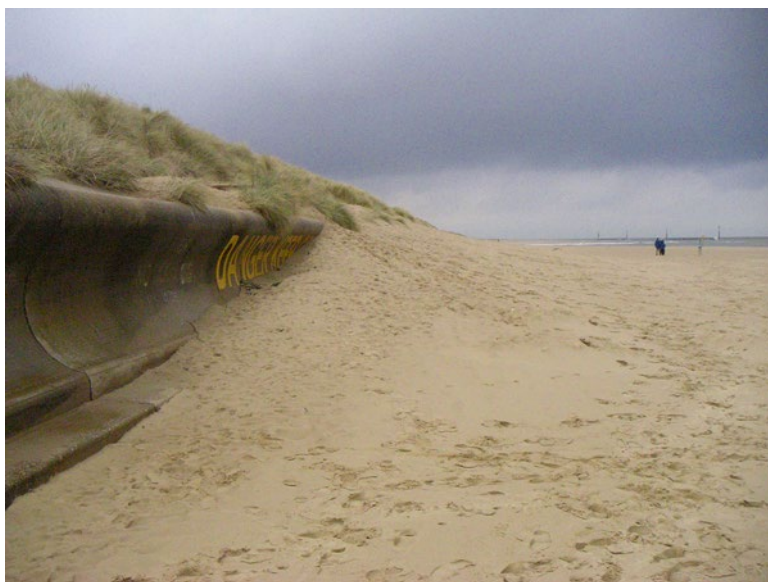
Fig. 9.2 The beach at Winterton with concrete sea wall in front of sand dune (Richard Dawson)
