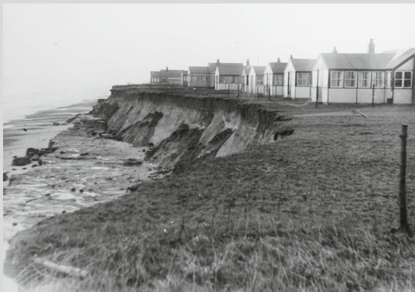
Fig. 12.4 Houses along beach road which once ran along the cliff top at Happisburgh, where the bay exists now (Image courtesy of Norfolk County Council Library and Information Service)
