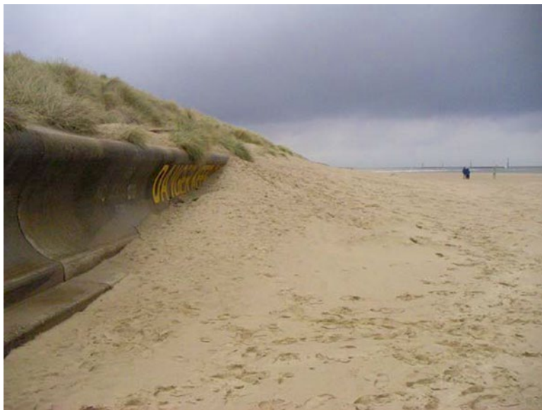
Fig. 1.13 Beach at Winterton with concrete seawall in front of sand dune on 31 October 2003 (the detached breakwaters are just visible on the horizon)
