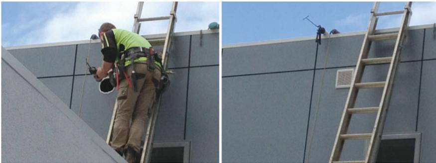
Fig. 12 Installation of roof ventilation, in total 4 of these vents were installed
