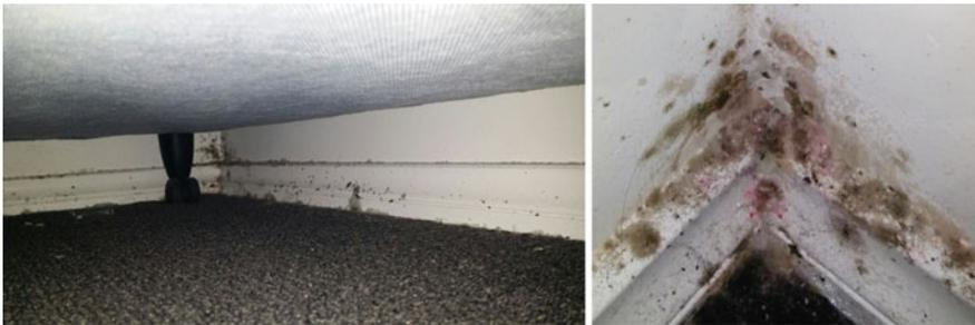
**Fig. 20** Under the bed, the wall and carpet have limited exposure to the heating and experience thermal bridging to the external walls
