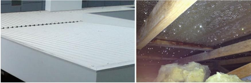
Fig. 13 The constantly wet, and often dripping underside of the roof
