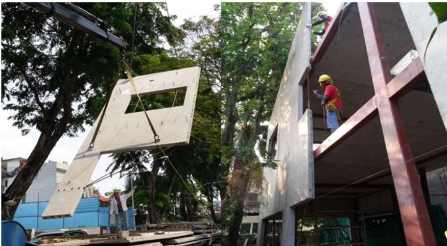
Fig. 7 Lifting of pre-cast wall and installing and clad onto modules at side elevation
