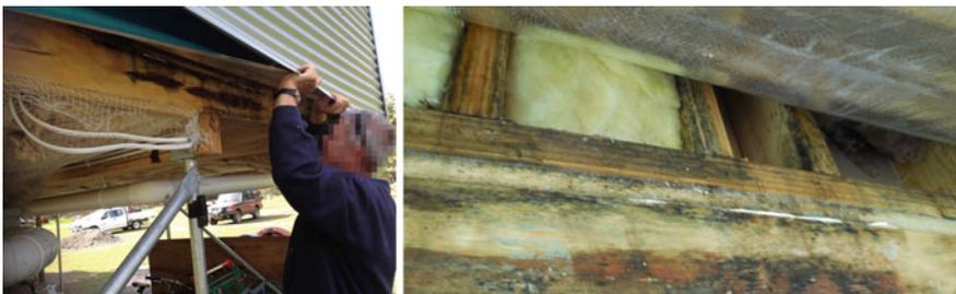
**Fig. 5** Often the true effect of condensation happens inside the wall framing. A builder helps dismantle the sheet metal cladding that is hard fixed against the studs (no battens) causing the wrap to be thermally bridged with the cold exterior. Indoor vapour, unable to pass through the foil wrap condenses on the insulation which acts as a reservoir, keeping the studs and bottom plate a moist breeding ground for mould
