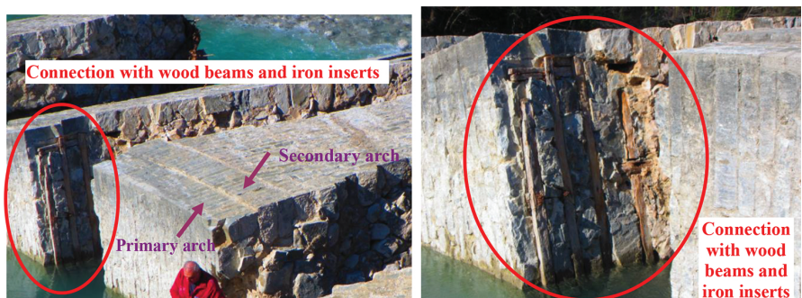
Figure 11. Connection with wooden beams and iron inserts between the primary and secondary arches of the Plaka Bridge.
