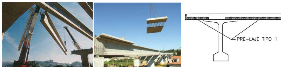
Figure 8. Placement of precast beams and pre-slabs.
