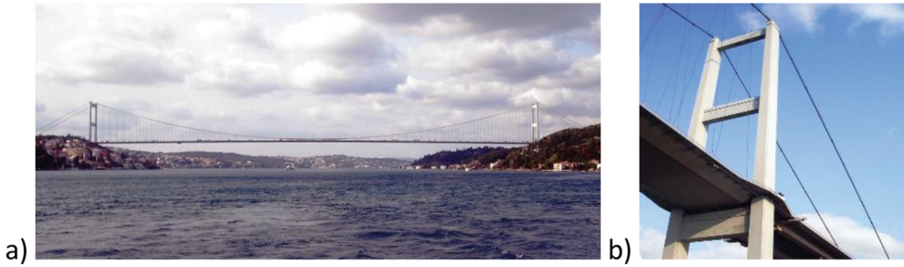
Figure 21. First Bosphorus Bridge: (a) side view; (b) tower and aerodynamic low profile deck.
