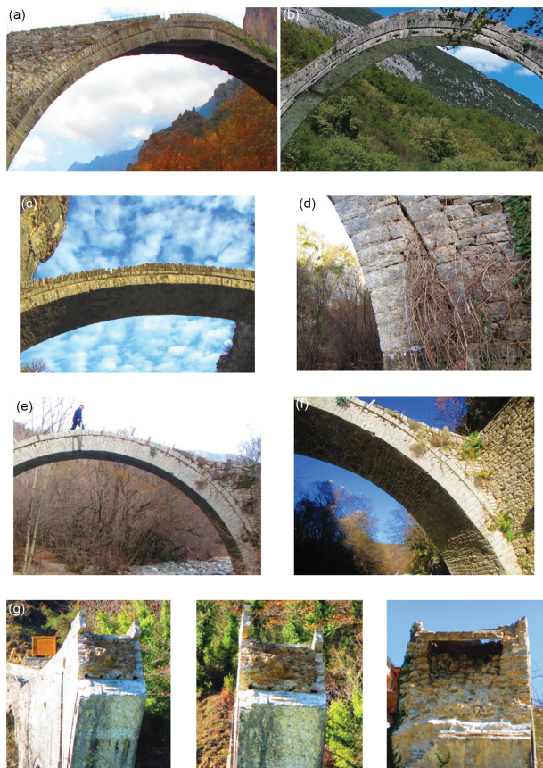
Figure 10. (a) Konitsa Bridge with the primary and secondary arches of the central span; (b) Plaka Bridge with the primary and secondary arches of the central span; (c) and (d) Kokorou Bridge with the primary and secondary arches of the central span; (e) and (f) Kontodimou Bridge with the primary and secondary arches of the central span; and (g) stone-masonry construction visible for the internal part of the mandrel walls of the remaining parts of Plaka Bridge.
