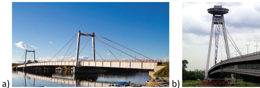
Figure 22. Cable stayed bridges: (a) Strömsund Bridge (1956) (photo by Lars Falkdalen Lindahl [25]); (b) the tower of the Bratislava SNU bridge, 1972.
