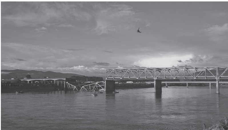
FIGURE 4.2 Skagit River Bridge collapse. (From https://commons.wikimedia.org/wiki/File:05-23-13_Skagit_Bridge_Collapse.jpg . Free to use by Wikipedia.)
