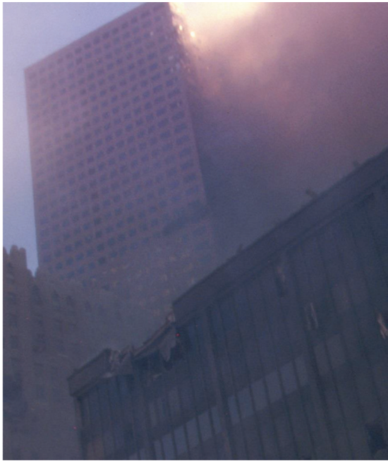
FIGURE 5.7 WTC7 collapse. (From http://upload.wikimedia.org/wikipedia/commons/thumb/0/0e/Wtc7onfire.jpg/511px-Wtc7onfire.jpg . Courtesy of the Prints and Photographs Division, Library of Congress, public domain.)
