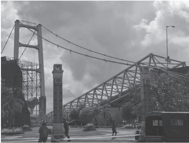
FIGURE 4.1 Collapse of the Kutai Kartanegara Bridge (From https://commons.wikimedia.org/wiki/File:Sisi_utara_jembatan.jpg , Free licence by Wiki.)
