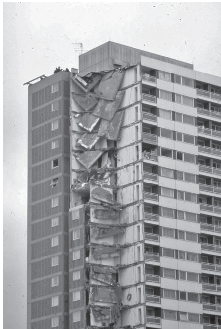
FIGURE 2.1 Ronan Point collapse. (From http://www.geograph.org.uk/reuse.php?id=2540477 . Image copyright © Derek Voller. This work is licensed under the Creative Commons Attribution—Share Alike 2.0 Generic Licence. To view a copy of this licence, visit http://creativecommons.org/licenses/by-sa/2.0/ or send a letter to Creative Commons, 171 Second St., Suite 300, San Francisco, CA 94105.)
