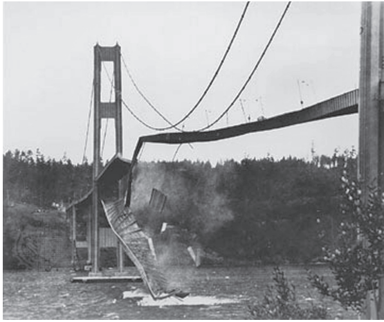
FIGURE 4.4 Tacoma Narrows Bridge collapse. (From https://upload.wikimedia.org/wikipedia/commons/4/4a/Tacoma-narrows-bridge-collapse.jpg . Public domain confirmed from Wikimedia.)
