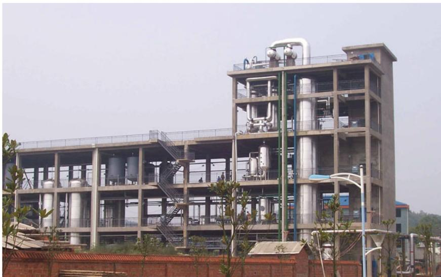
**Fig. 1** The first industrial plant for biodiesel production using lipase catalysis
