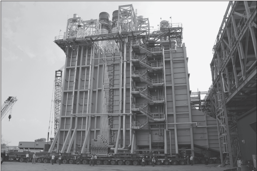
Fig. 1-1. Transporting this HRSG blocks road and access for hours. (Courtesy of KOG Transport, Inc., USA)
