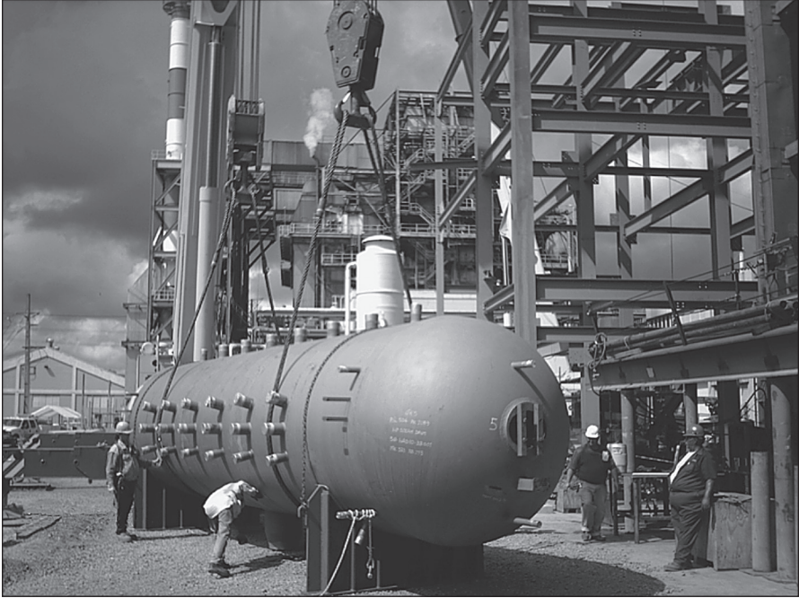
Fig. 1-2. Drum positioning with hydraulic cranes
