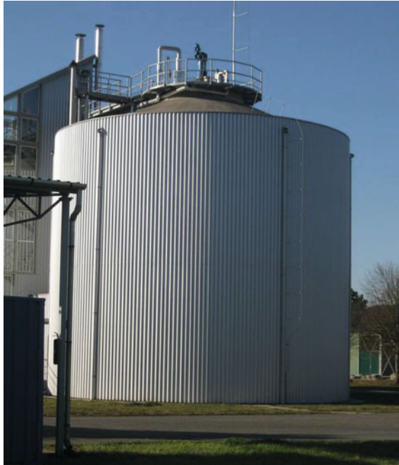
Fig. 2 Wastewater treatment plant, high digester tower. Source own photo
