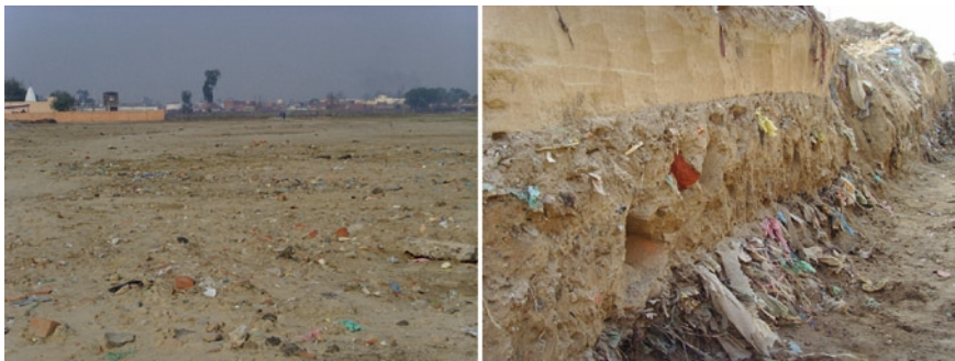
Fig. 3.21 Brownfield in Panipat, India ( left ), soil profile of the site ( right ) consisting of waste overlaid by a soil-waste mixture and a sandy layer; the soil properties exacerbate a future use of the built-up area
