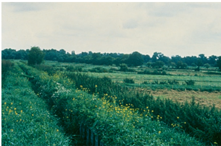
Fig. 5.17 Sewage sludge treatment field in Berlin, Germany; the field is surrounded by earthen dams and a sheet-pile wall of steel
