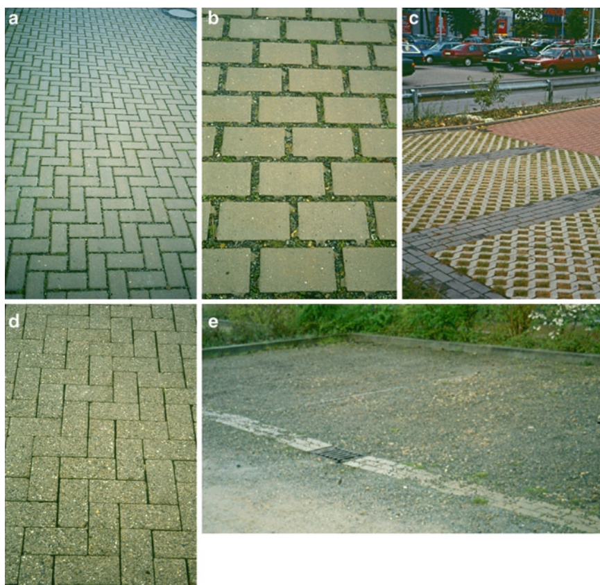
Fig. 6.2 (a) Sealing materials: small slabs with narrow joints (0.5 cm) and reduced water infiltration rate. (b) Sealing materials: small slabs with wide joints (2 cm) and high water infiltration rate. (c) Sealing materials: honeycomb-type paving stone with high water infiltration rate. (d) Porous perforated sealing material with decreasing water infiltration rate in the course of time because of blocking and clogging by dust. (e) Water-bounded cover with high water infiltration rate
