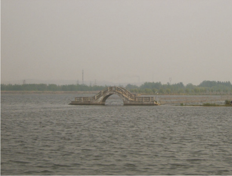
Fig. 6.9 Continuously progressing water logging and development of an artificial lake caused by subsidence in a coal mining area in Huaibei, China
