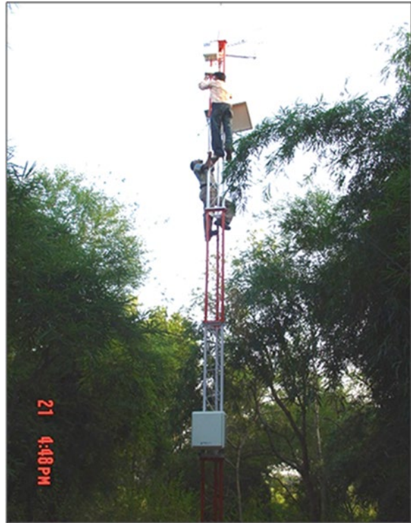
Fig. 3.7 Eddy covariance system installed at reclaimed site, Gumgaon, Nagpur. Eddy-covariance/eddy-flux systems measure three-dimensional wind direction and simultaneous gas concentrations
