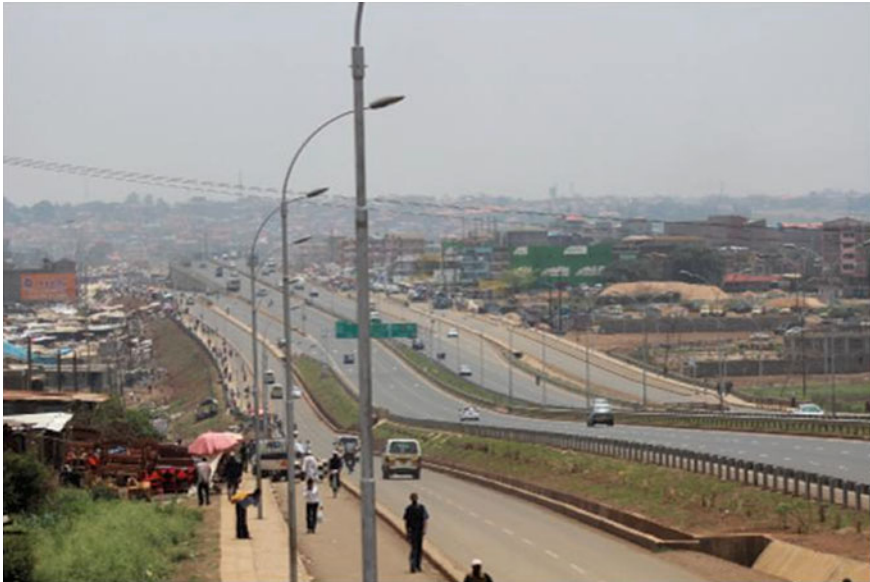
Fig. 6 Non-motorized areas on the Thika superhighway. Pedestrians using the incorporated non-motorized lanes on the Thika superhighway. Source GSC (2012)
