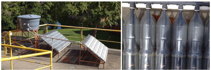
Fig. 12 Solar water heating system with PET bottles—PET bottles with Tetra Pak boxes. Source Alano (2009)
