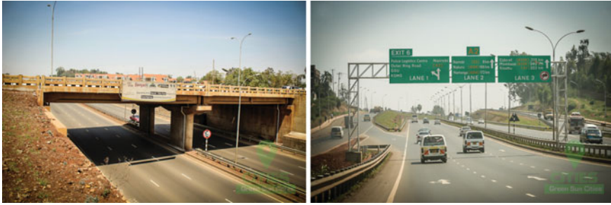
Fig. 3 Images of newly completed Thika superhighway. View of the eight-lane completed superhighway section underpass decongesting traffic in Nairobi. Source GSC (2012)
