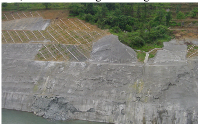
Fig.1. Slope with creep deformation on the left bank (0+480~0+530)
