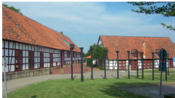
Fig. 2 New LED street lighting in the rural community of Schladen (Germany). Example of energy-saving RLAP
