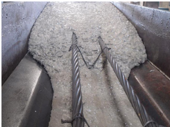
Fig. 4.2 Concrete pouring into the formwork
