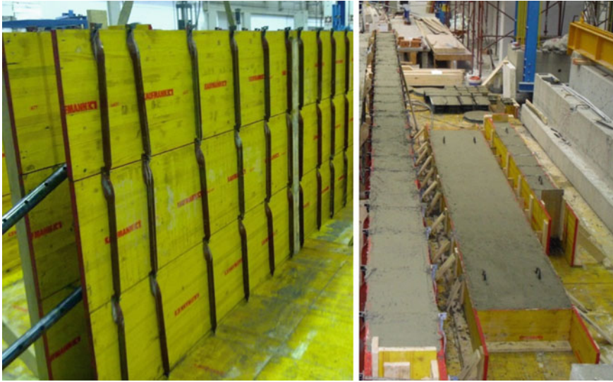
Fig. 5.11 Formworks and beams just casted
