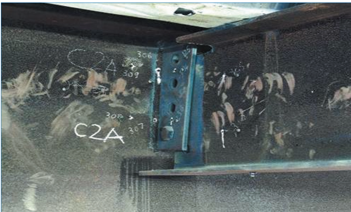
Figure 5.5 Shear failure of bolts in a steel connection
