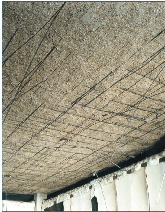
Figure 5.2 Spalling of concrete 48
