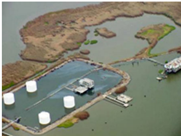
Fig. 6 Flooded wastewater treatment plants (EPA 2012)
