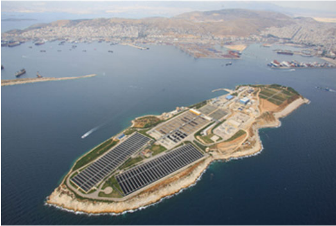
Fig. 5 Psittalia wastewater treatment plant, Athens, Greece (Psittalia 2013)
