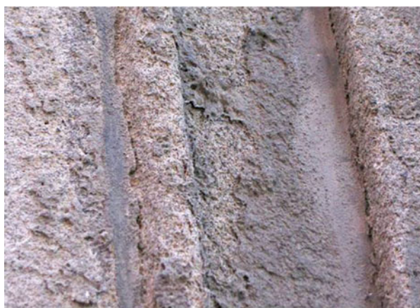
Fig. 1.10 Suspected application of protective treatment that is thought could have contributed to further erosive processes (resulting from salt crystallisation at interface with substrate)
