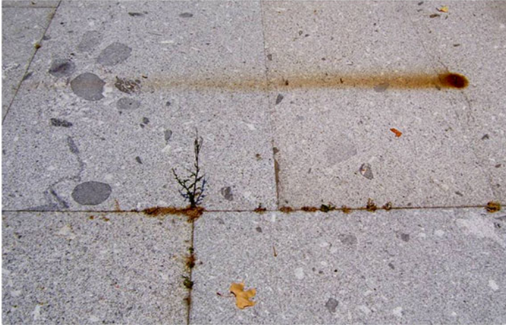
Fig. 1.9 Stains related to alteration of petrographic heterogeneity on granite pavement slabs (the distribution of the stain crossing the slabs edges shows that it develop after emplacement of the stones)
