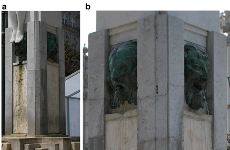
Fig. 1.5 Erosive marks on carbonate stones on a fountain related to the circulation of water ( a, b )
