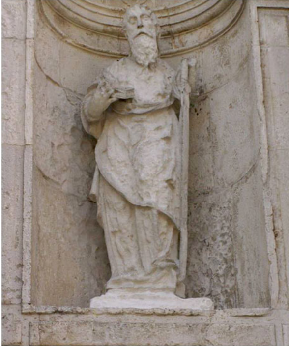
Fig. 1.7 Physical disruption processes leading to erosion of material in limestone statuary (exemplifying a situation in which consolidation procedures could be considered to avoid the progression of erosion and further loss of detail)
