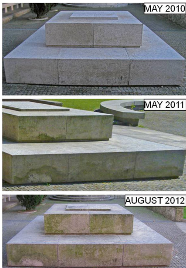
Fig. 1.4 Comparison of stones cleaned in the first semester of 2010 showing the recurrence of biological colonisation ( greenish-greyish stains )
