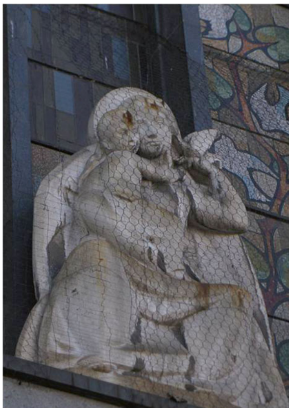
Fig. 1.2 Stains in statuary that seem related to alteration of metallic structures
