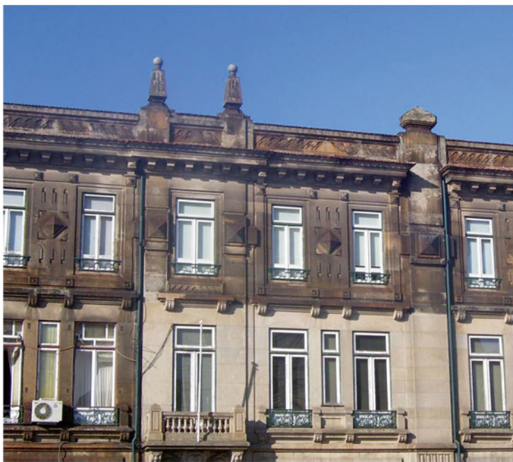
Fig. 1.1 Example of façade cleaning where the evaluation of the whole result might be a polemical subject
