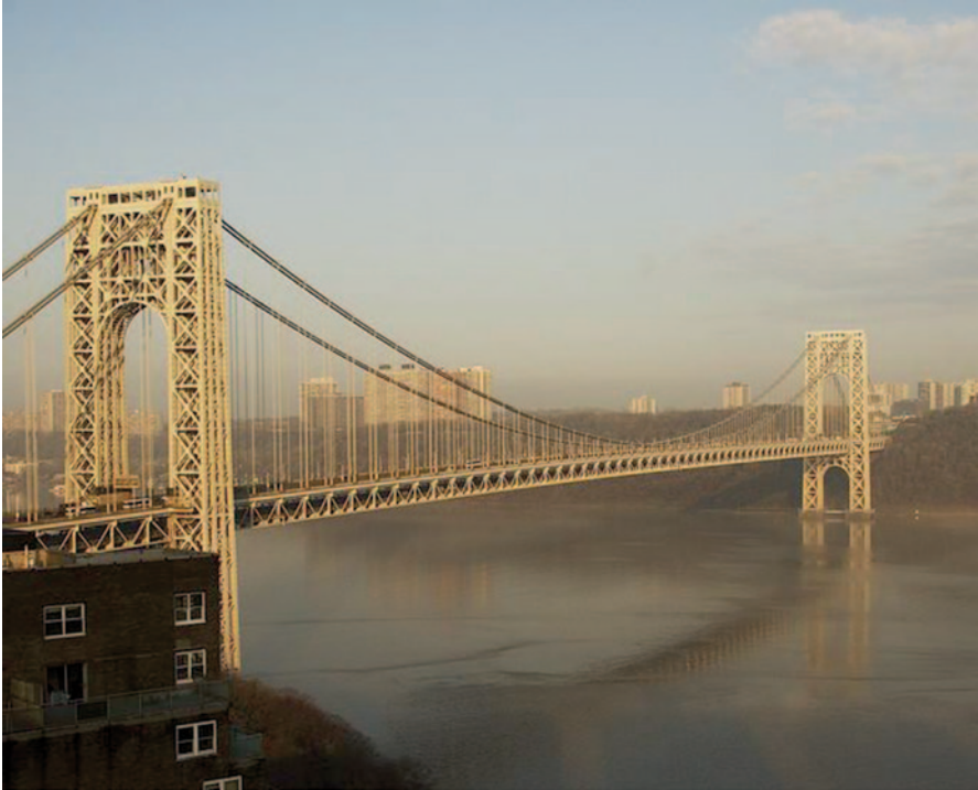
Fig. 12.2 George Washington Bridge looking from Manhattan to New Jersey. (Source: Fly Navy (28 April 2007) available at http://www.flickr.com/photos/mgreene/476286568/ )
