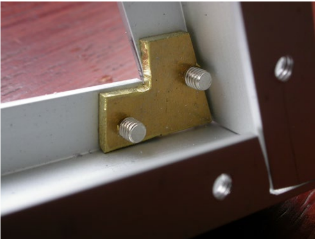
Figure 7-13. The brass corner fixings
