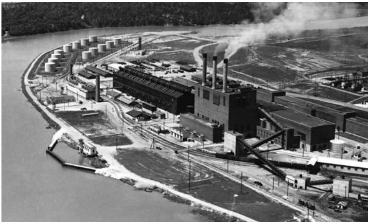
Fig. 5.29 The S-50 facility. The main process plant is the long, dark building to the left of center. The K-25 powerhouse (three smokestacks) is to its right, and a tank farm for supplying oil for the “new boiler plant” is to the left. The new boiler plant itself is between the main process building and the river. Source http://commons.wikimedia.org/wiki/File:S50plant.jpg
