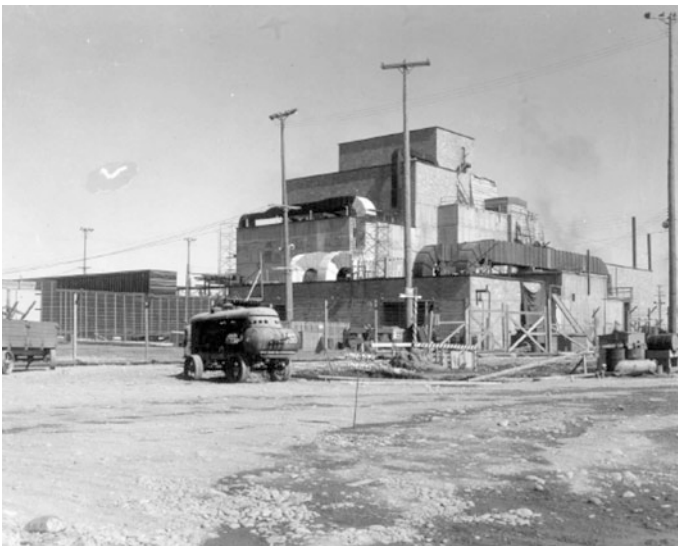
Fig. 6.4 The B-pile building under construction. (HAER, Photo 3)
