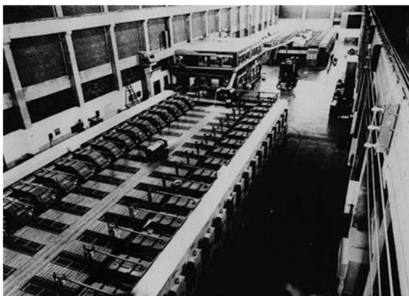
Fig. 5.18 This photograph, reproduced from Manhattan District History microfilms, shows two Beta tracks, one in the foreground and one in the background. Source A1218(10), image 0231
