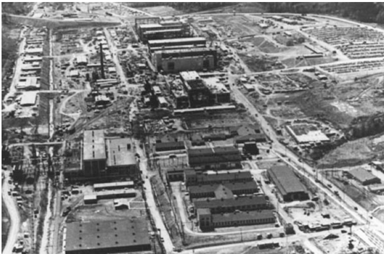
Fig. 5.22 Construction at Y-12, 1944. Source http://www.y12.doe.gov/about/history/getimages.php
