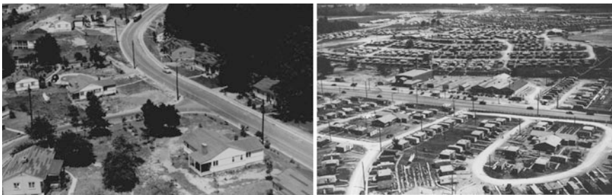
Fig. 5.1 Typical cemesto homes and a trailer-housing area at Oak Ridge. Source http://www.y12.doe.gov/about/history/getimages
