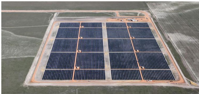
Fig. 12.8 Greenough river 10 MW solar electricity farm near Geraldton. All of its production is purchased by WA water corporation to offset part of the energy used at Southern seawater desalination plant
