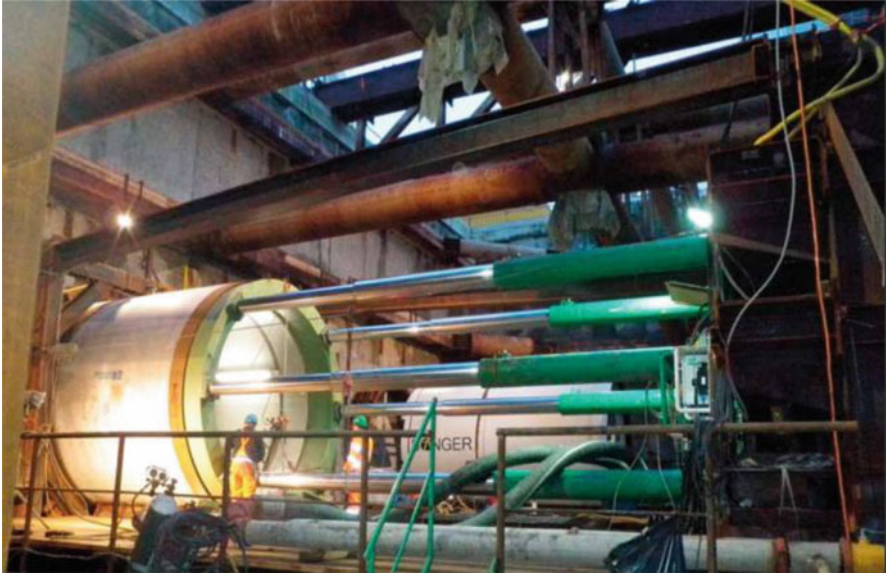
Fig. 6.6 Jacking cylinder pushing machine ahead from launch shaft
