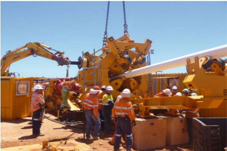
Fig. 6.13 Pipe Thrusters in operation to install supply line
