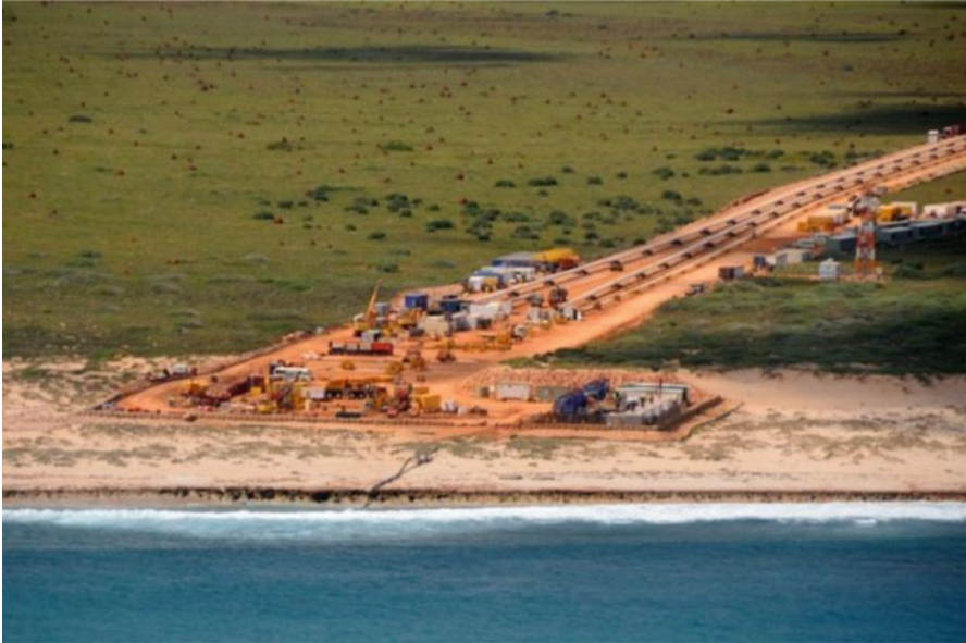
Fig. 6.12 View on jobsite Barrow Island
