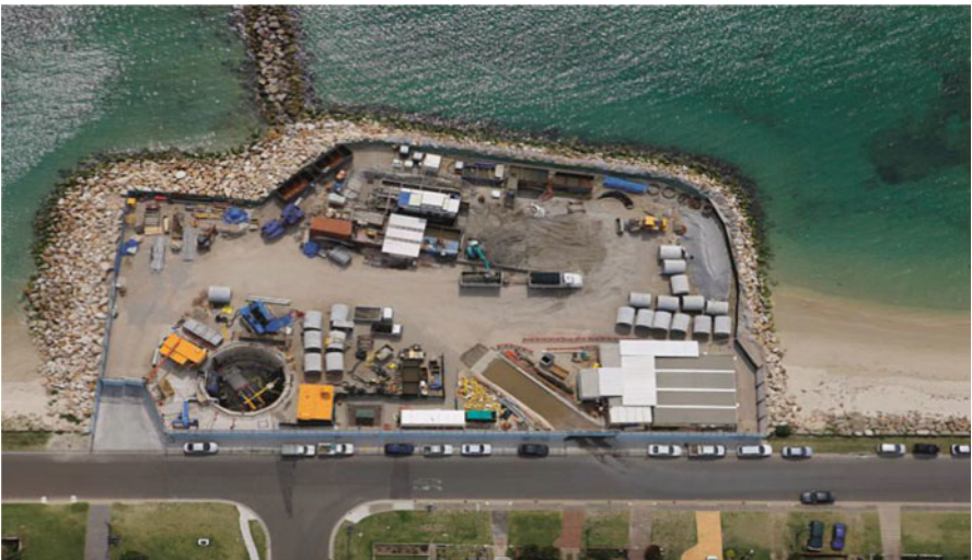
Fig. 6.10 Launch shaft of AVND 2000
