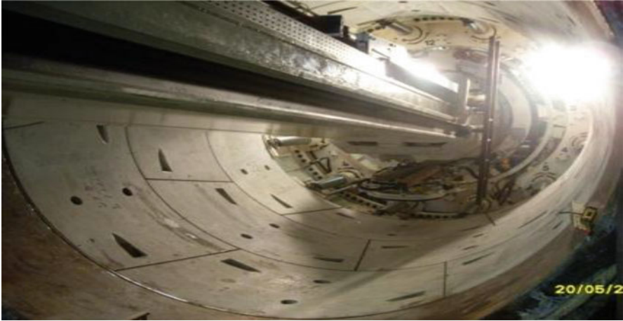
Fig. 6.9 View into machine and segment ring construction with erector
