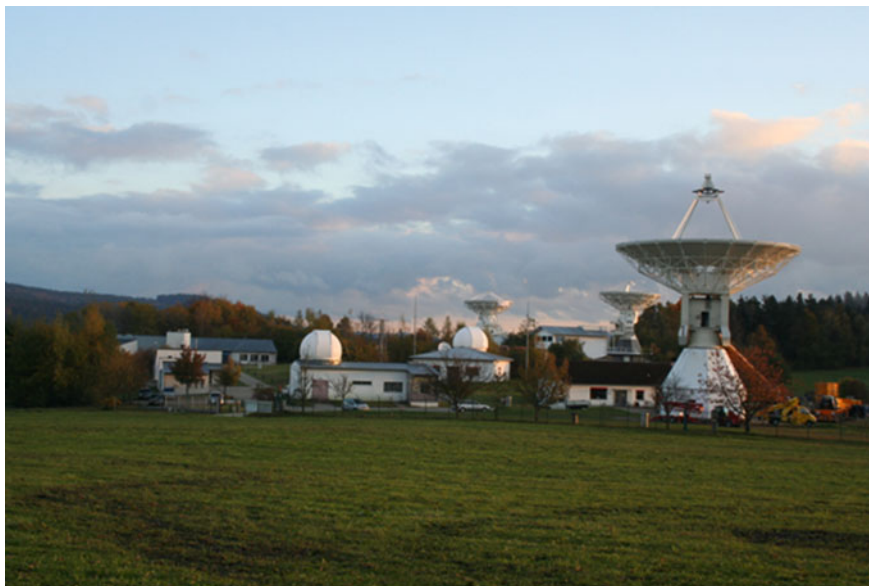
Fig. 3.5 Geodetic Observatory Wettzell (Germany) with co-located VLBI, SLR, and GPS instruments. The observatory is jointly operated by the Bundesamt für Kartographie und Geodäsie ( BKG ) and the Forschungseinrichtung Satellitengeodäsie ( FESG ), Technische Universität München. Clearly visible are the recently installed twin telescopes, the 20 m radiotelescope and two laser ranging systems (Courtesy: A. Neidhardt, FESG)
