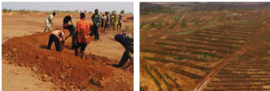
Fig. 16.3 Construction of contour bunds ( left ). Rows of contour bunds ( right ) (Source: GIZ 2012)
