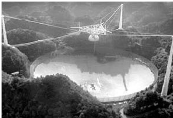
Fig. 14.28. Radiotelescope of Arecibo in Puerto Rico. The antenna lies on the bottom of a 300-meter diameter volcano. (Photo credit: National Astronomy and Ionosphere Center, Cornell U., NSF http://antwrp.gsfc.nasa.gov/apod/ap981129.html .)
