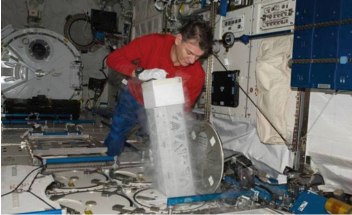
Fig. 2.10 ESA astronaut and ISS Engineer Paolo Nespoli, services the Minus Eighty deg Laboratory Freezer for ISS (MELFI-1) in the ISS Kibo laboratory in December 2010 (Source: NASA)
