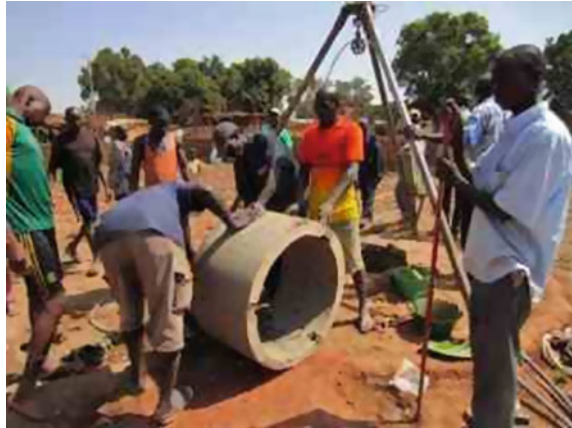
Fig. 13 A well-drilling team in Burkina Faso (Source WI 2014)
