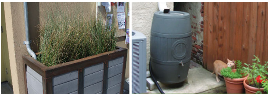
Fig. 7 Flow-through planter ( left ) and rain barrel ( right ) (Source PWD 2013)
