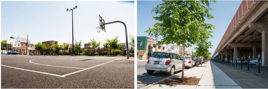
Fig. 6 Porous pavement ( left ) and tree trench ( right ) [Source CDM Smith (the support of CDM SMITH in providing reference material is kindly acknowledged)]
