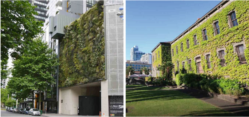
Fig. 5 A green wall ( left ) and a green façade ( right ) in Melbourne ( Source DEPI (2014))
