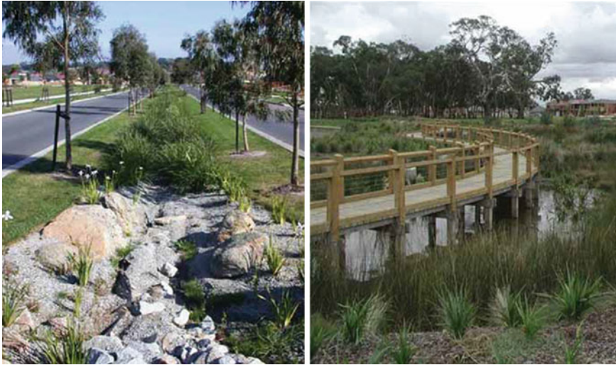
Fig. 3 Biofiltration systems ( left ) and artificial wetland ( right ) in Lynbrook Estate ( Source wsud.org; Brown and Clarke 2007)
