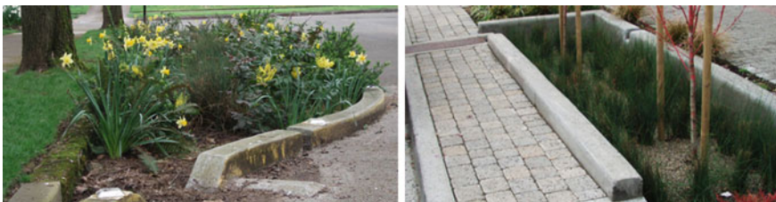
Fig. 9 Stormwater bump-out ( left ) and stormwater planter ( right ) ( Source PWD 2013 )
