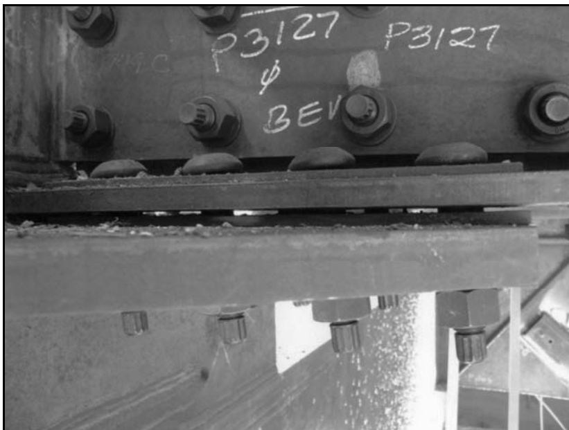
Poor Bolt Fit-up
