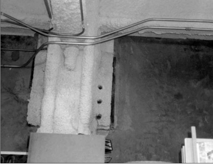
Shear failure of bolts at shear plate at tilt-up wall Northridge Earthquake, Los Angeles, 1994
