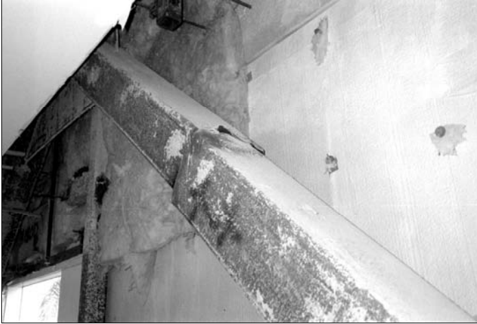
Fracture of steel tube brace member at center of brace Northridge Earthquake, Los Angeles, 1994
