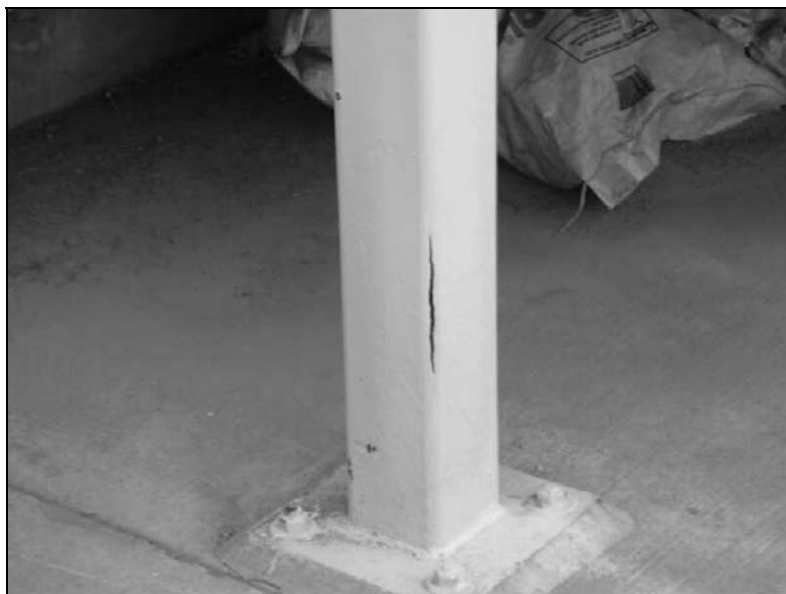
Cracked Post at Stair
