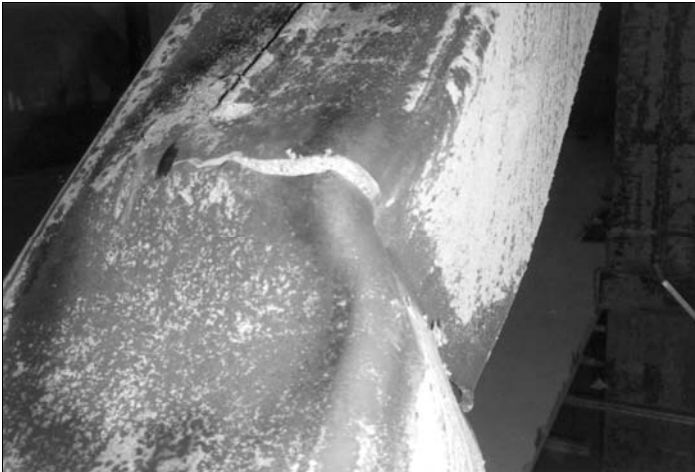
Local buckling of steel tube brace member at center of brace Northridge Earthquake, Los Angeles, 1994
