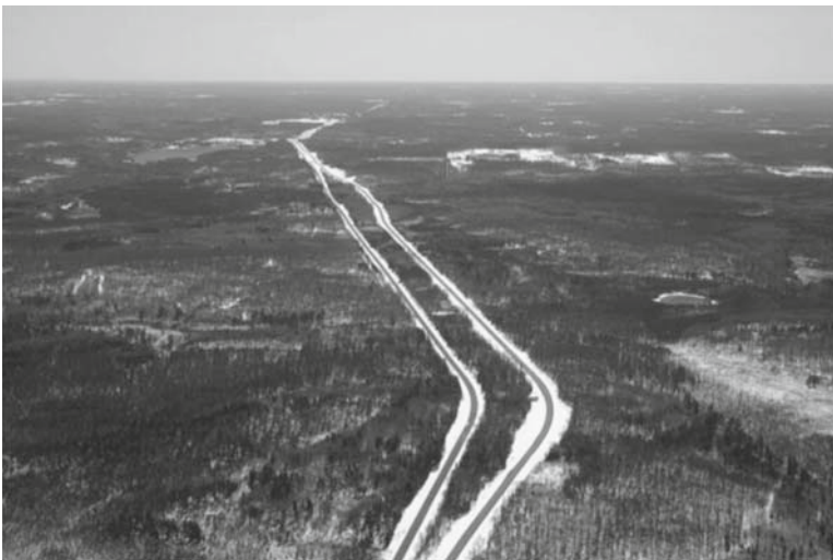
Fig. 14.2 One of the seven “ballooned strips” constructed along US 53 to facilitate wolf crossings of the upgraded highway. Natural vegetation was maintained in a \geq 100 -m median between center-lines of the two lanes. Wolves crossing the highway in ballooned strips encountered traffic coming from only one direction at a time. (WDNR photo by Joseph F. Sprenger 2007)
