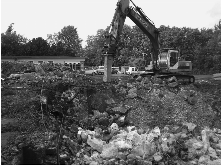
8.8 Use of hydraulic breakers to destroy fundamentals of a building.
