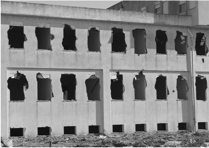
7.4 Punching out of windows, using heavy mechanical equipment.
