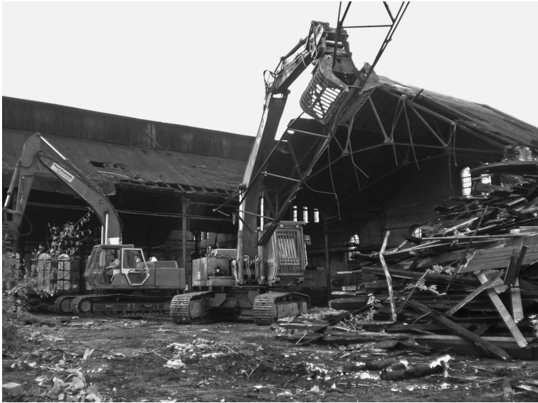
8.7 Grabbing lightweight parts of, for example, the roof structure.
