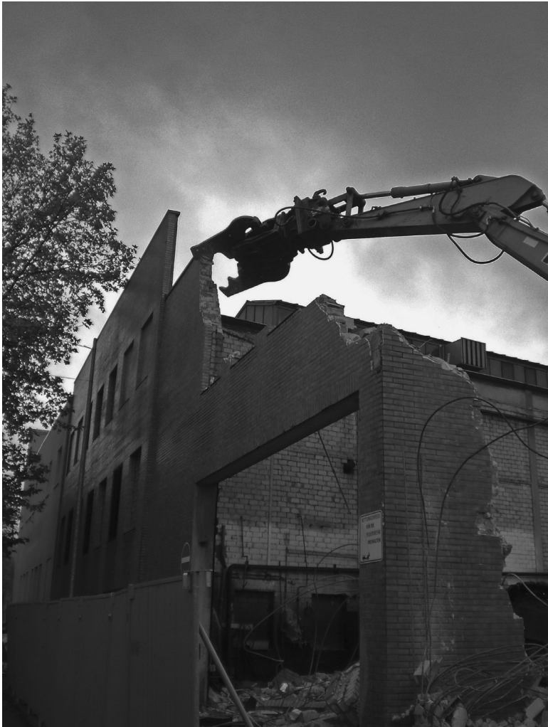
8.4 Cracking shears only affect small surrounding areas. This causes a high level of control.
