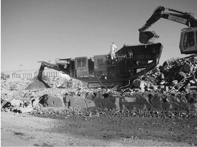
9.2 Mobile crushing unit, with magnetic separator, without grain size separation capacity.
