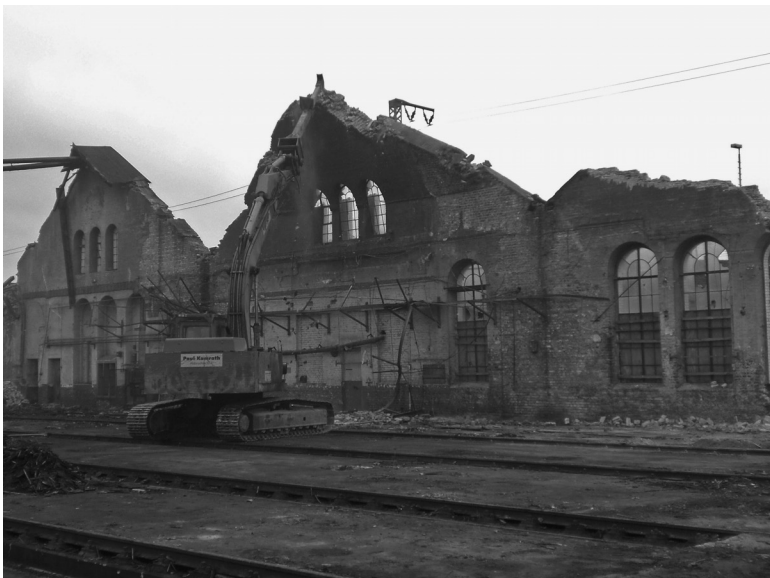
8.6 To extend the reach of the excavator, special pushing/pulling devices can be used.
