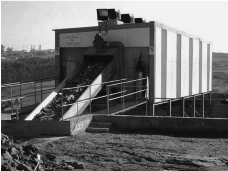
9.3 Manual separation cabin, at a fixed level 1 CDW recycling plant.
