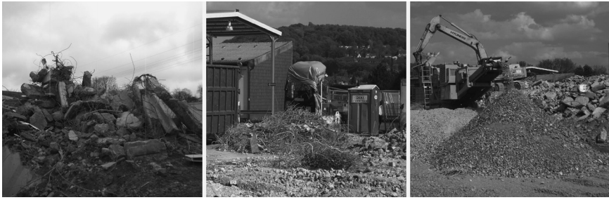
8.1 States of concrete during recycling progress: Concrete as given after deconstruction by machines (left), separated core wires (middle) and gravel of concrete (right).
