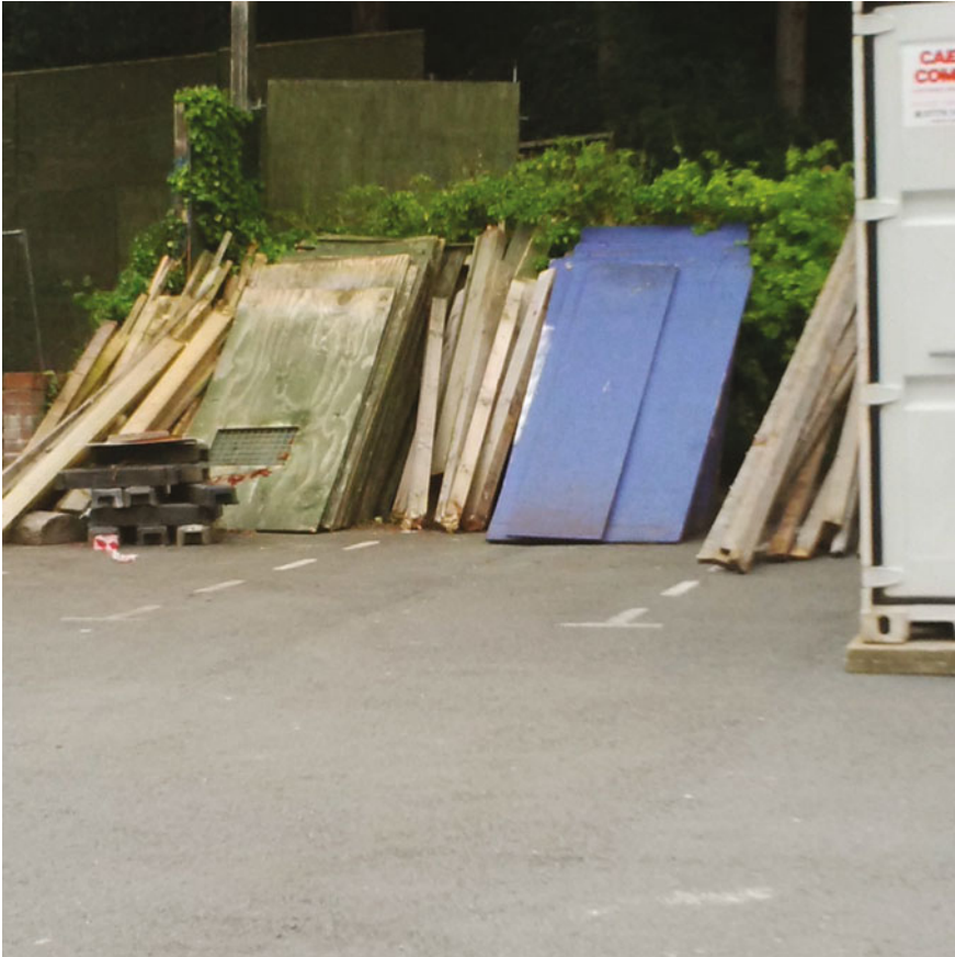
Fig. 15 Timber removed during construction work may be a mixture of structural material from the building, and site-generated waste such as hoardings, covers and formwork timbers
