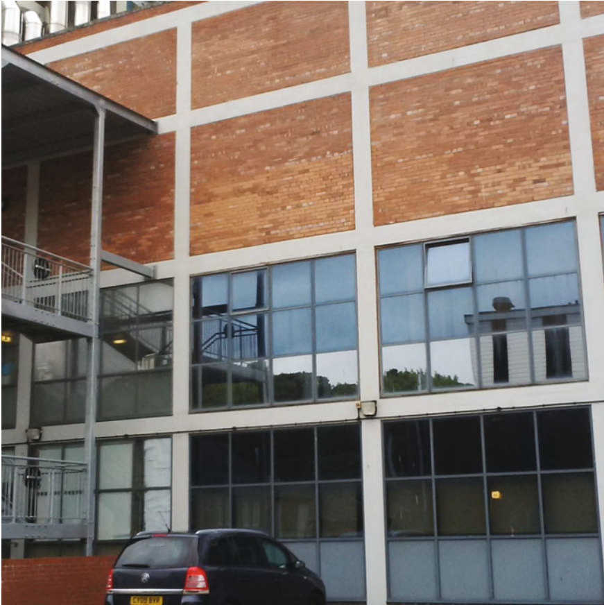
Fig. 4 Modern buildings may not appear to contain much timber
