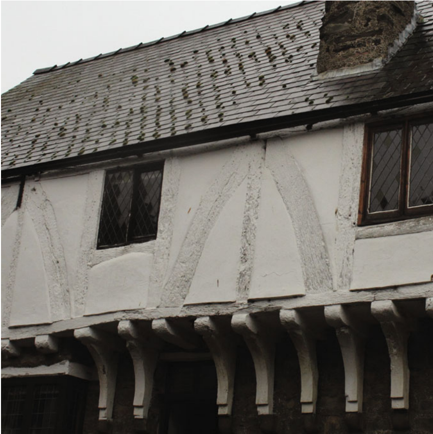
Fig. 1 Early buildings in Britain frequently used wood as the primary structural elements
