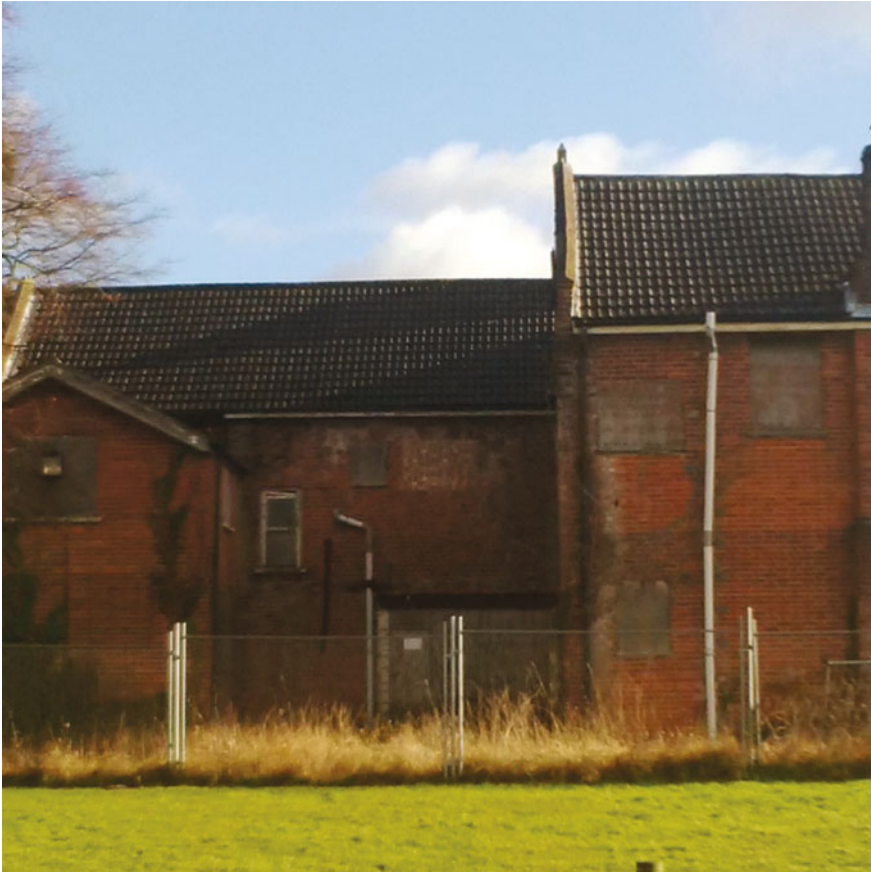
Fig. 9 Typical brick and block construction awaiting demolition or remodelling
