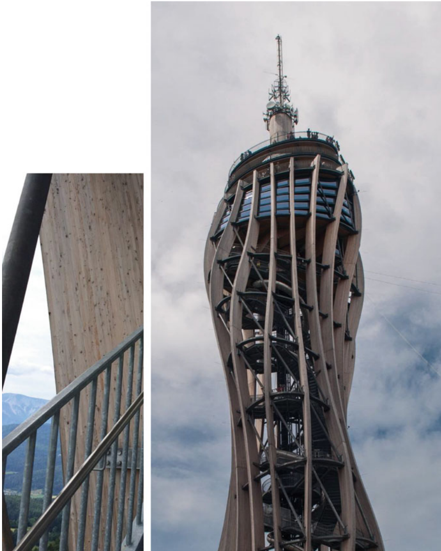
Fig. 1 Use od glulam in “Pyramidentower” in Carinthia, Austria (Photo: Andreja Kutnar)
