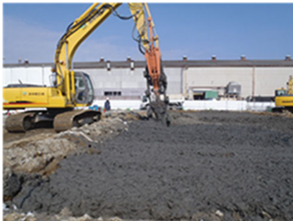
Fig. 7.8 On-site immobilization of fluoride-polluted soil using DCPD
