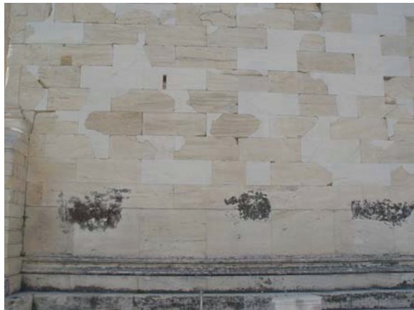
Fig. 5.5 Black biofilm on specific places in the restored backside of the Erechtheion (Akropolis, Athens, Greece). Ancient and replaced marble blocks are recognised by different biopatina. Black biofilm spreads in places where – behind the wall – water can pass
