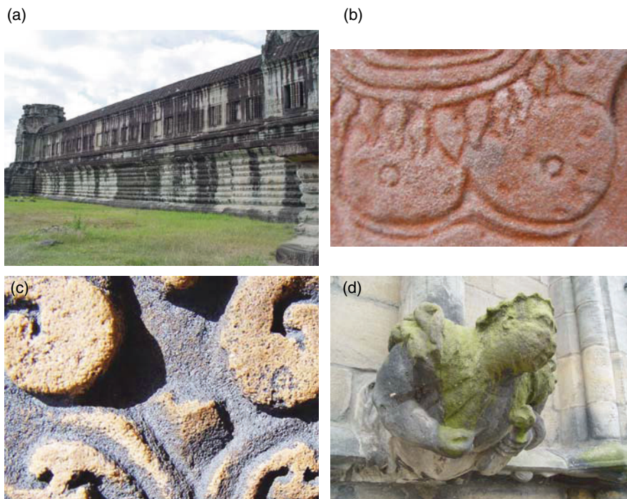
Fig. 5.7 Biofilm cover at different sites. Upper left : Black biofilms composed of algae, cyanobacteria, and fungi at Angkor Wat; upper right : Angkor Wat Temple freeze with red pigment of lichen growth and biopitting fungi; lower left : blue biofilm pigment from lichen growth in Thai temple, Southern Thailand; lower right : black and green biofilm on lion heads at Sterling Castle, Scotland. In all cases neither pollution nor artificial paint traces exist, it is pure biological growth
