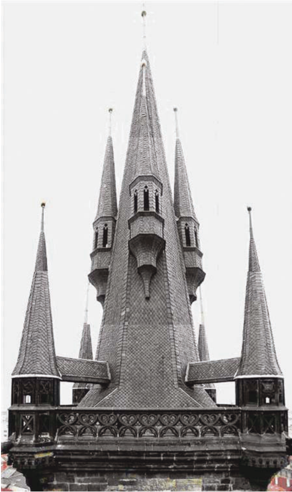
Fig. 8.7 A typical gothic tower, with sharp edges used as the prototype tower for numerical studies
