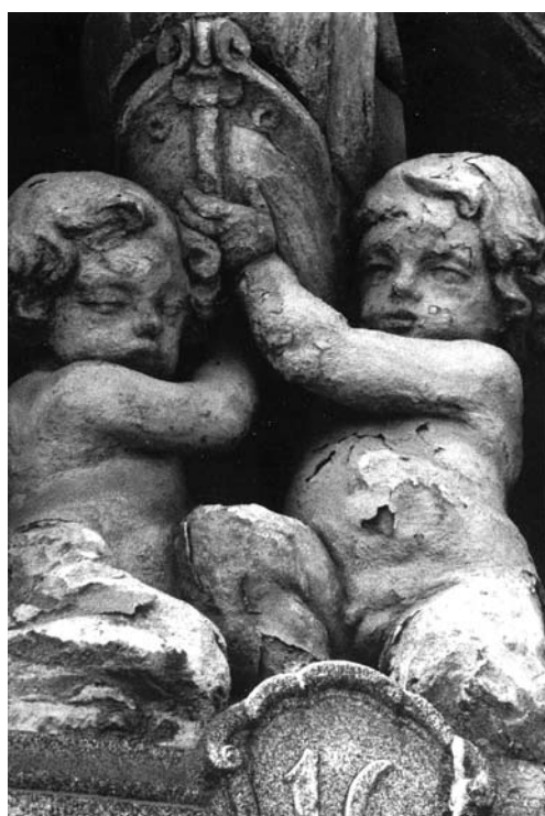
Fig. 3.2 Portal figures of sandstone in the Old Town in Stockholm
