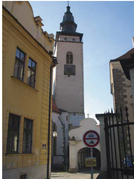
Fig. 8.26 Environmental, economy and life cycle data for Gothic Building, St Jacob’s Church, Telc
