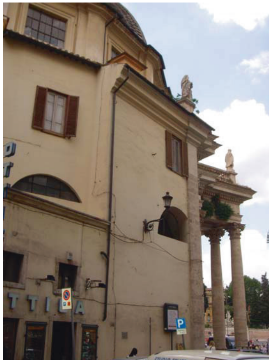
Fig. 6.30 Frontage on the Piazza del Popolo (90% travertine, 10% painting) and side on the Via del Babuino n° 199 (5% travertine, 95% painting) of the Santa Maria del Monte Santo Church, Rome
