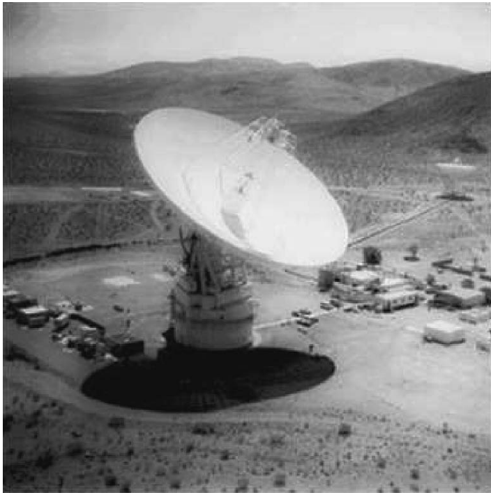
Fig. P.1. Aerial view of Deep Space Network (DSN) at Goldstone, Mojave Desert, Southern California. The giant 70 m dish is in the foreground, a dozen other smaller dishes are located around it spaced up to 10 km from one another. Courtesy NASA/JPL-Caltech
